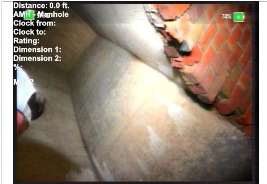
At: 0 ft. AMH - Manhole Joint: No MH12
