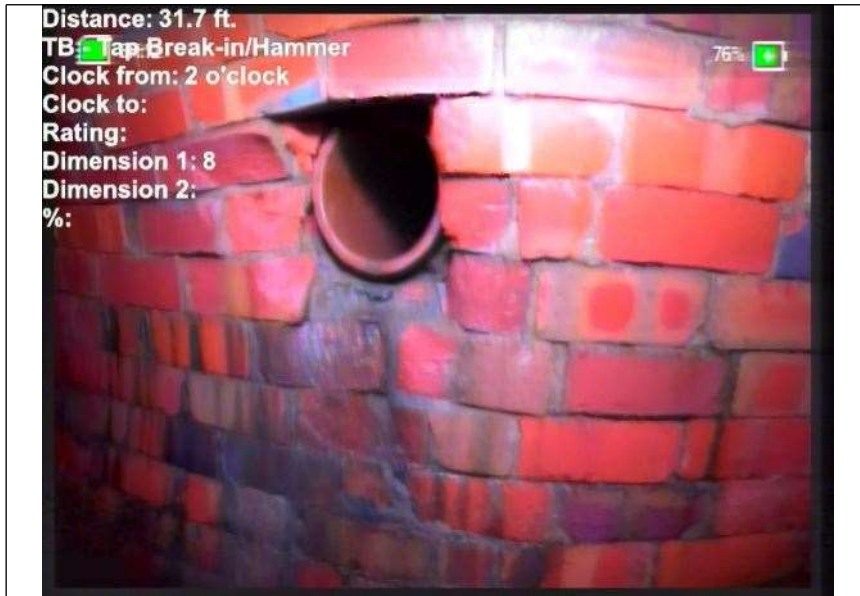
At: 31. TB - Tap Break-in/Hammer 7000007629 395 ft. 2/.
