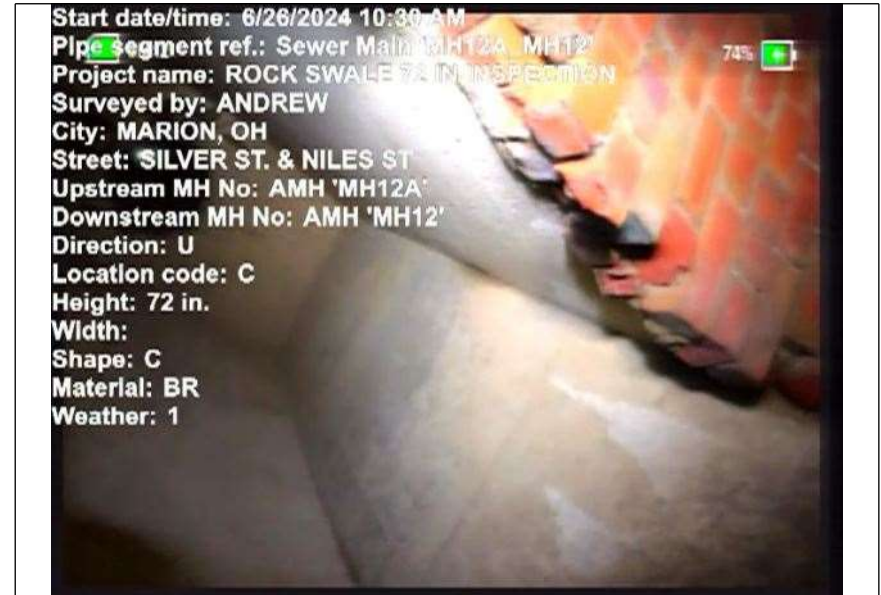
At: 0 ft. AMH - Manhole Joint: No MH12
