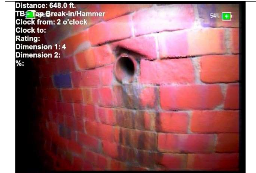
At: 648 ft. 2/. TB - Tap Break-in/Hammer Joint: No
