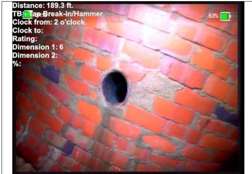
At: 189. TB - Tap Break-in/Hammer 3000030517 58 ft. 2/.
