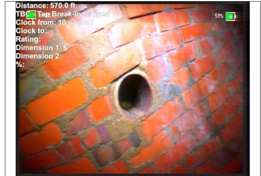
At: 570 ft. 10/. TBC - Tap Break-in Capped Joint: No
