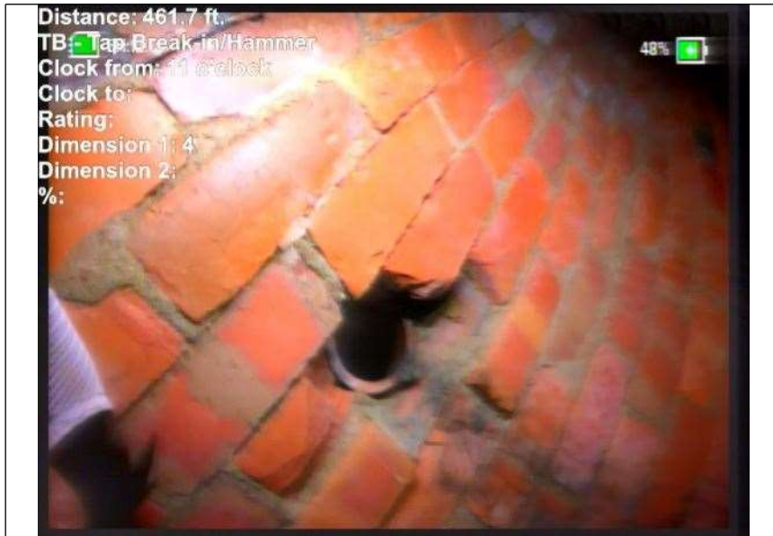
At: 461. TB - Tap Break-in/Hammer 7000122070 31 ft. 11/.
