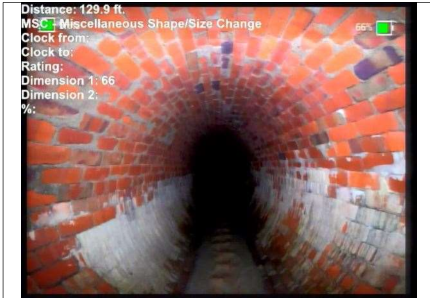
At: 129. MSC - Miscellaneous Shape/Size Change 8999938964 84 ft.
