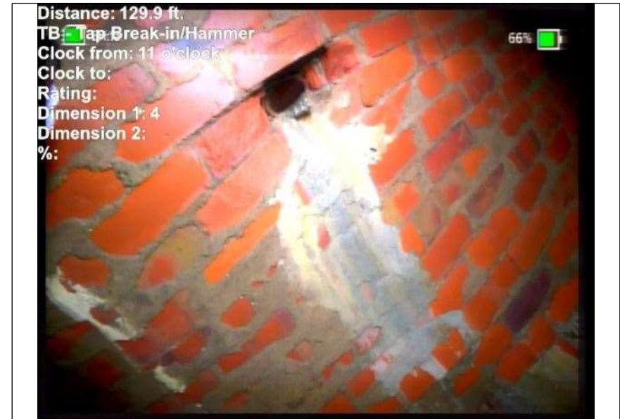
At: 129. TB - Tap Break-in/Hammer 8999938964 84 ft. 11/.
