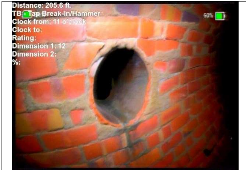
At: 205. TB - Tap Break-in/Hammer 6000061035 16 ft. 11/.
