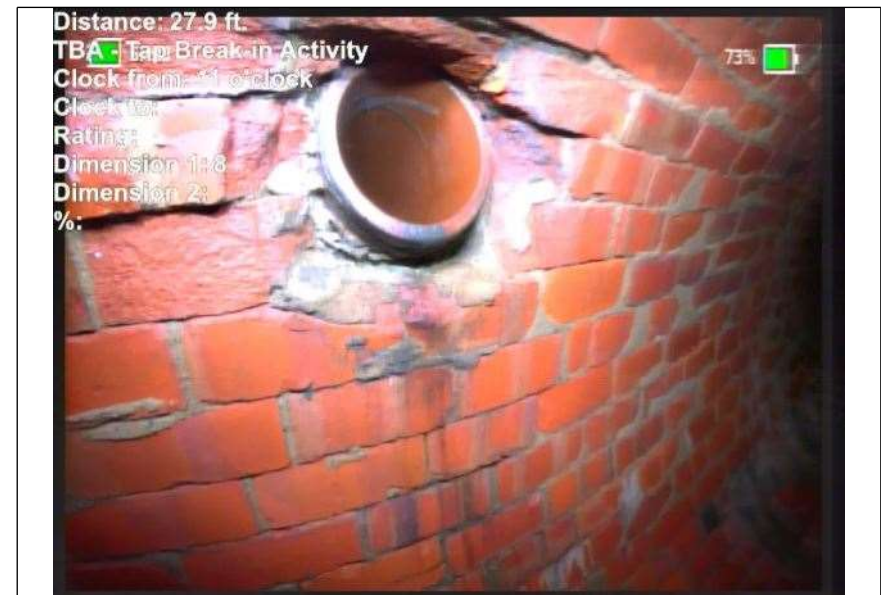
At: 27.9 ft. TBA - Tap Break-in Activity 8999996185 303 ft. 11/. Joint: No
