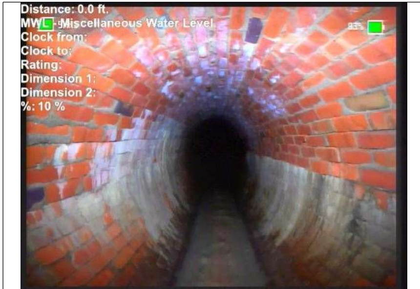
At: 0 ft. MWL - Miscellaneous Water Level Joint: No 10 %
