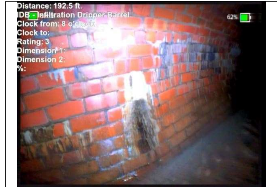
At: 192.5 ft. 8/. IDB - Infiltration Dripper Barrel Joint: No
