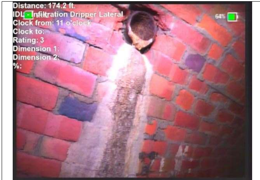
At: 174. IDL - Infiltration Dripper Lateral 1999969482 42 ft. 11/.
