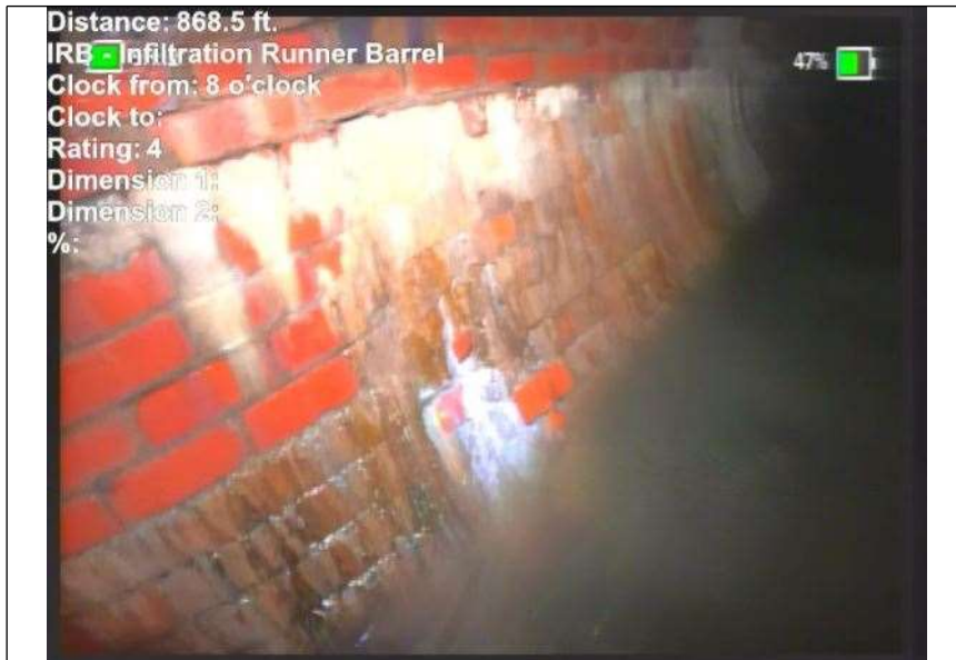
At: 868.5 ft. 8/. IRB - Infiltration Runner Barrel
