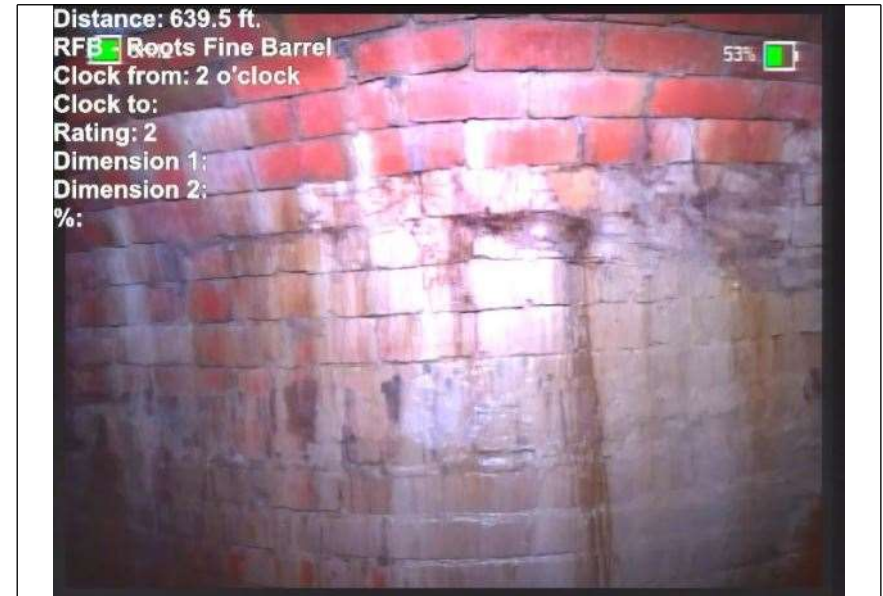
At: 639.5 ft. 2/. RFB - Roots Fine Barrel Joint: No
