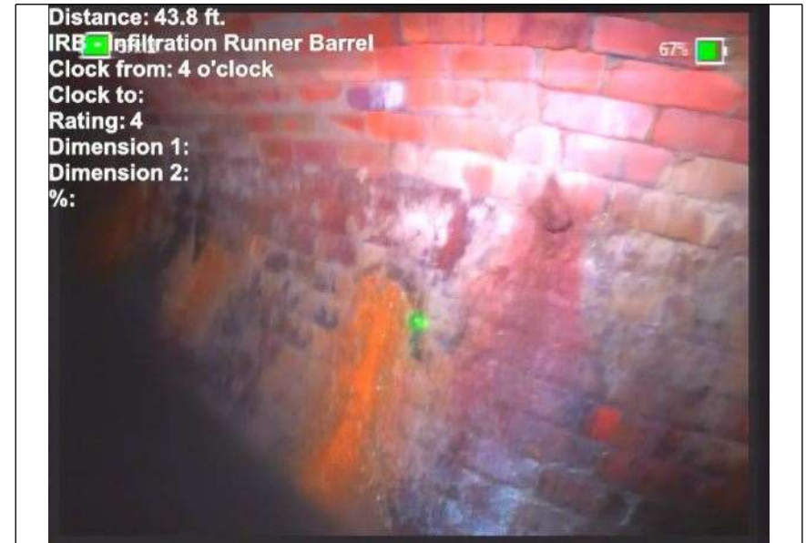
At: 43.8 ft. IRB - Infiltration Runner Barrel 7999992370 605 ft. 4/. Joint: No
