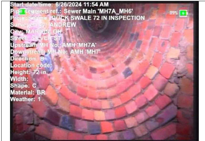
At: 0 ft. AMH - Manhole Joint: No MH7A
