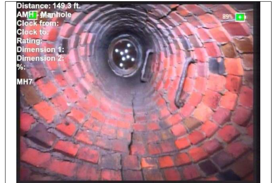
At: 149. AMH - Manhole 3000030517 58 ft.
