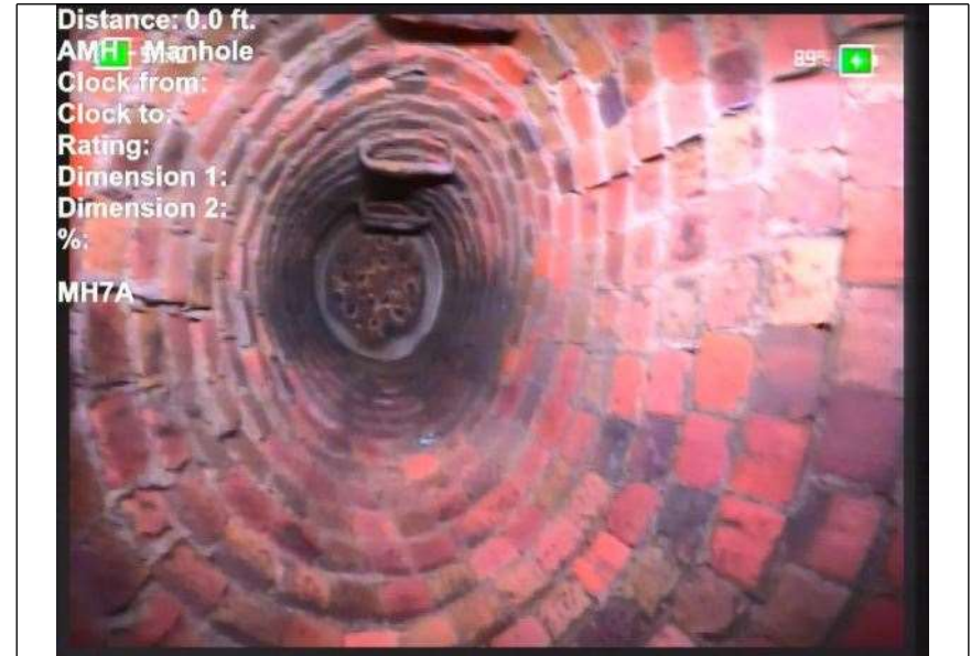
At: 0 ft. AMH - Manhole Joint: No MH7A
