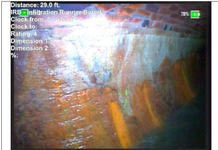
At: 29 ft. 8/. IRB - Infiltration Runner Barrel
