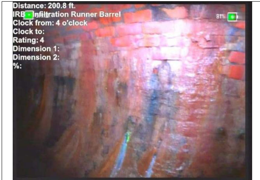
At: 200. IRB - Infiltration Runner Barrel 8000030517 58 ft. 4/.
