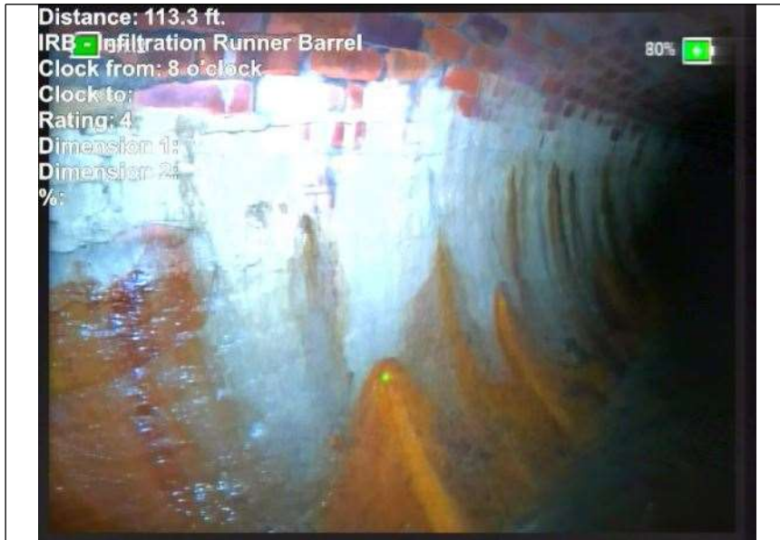
At: 113. IRB - Infiltration Runner Barrel 3000030517 58 ft. 8/.
