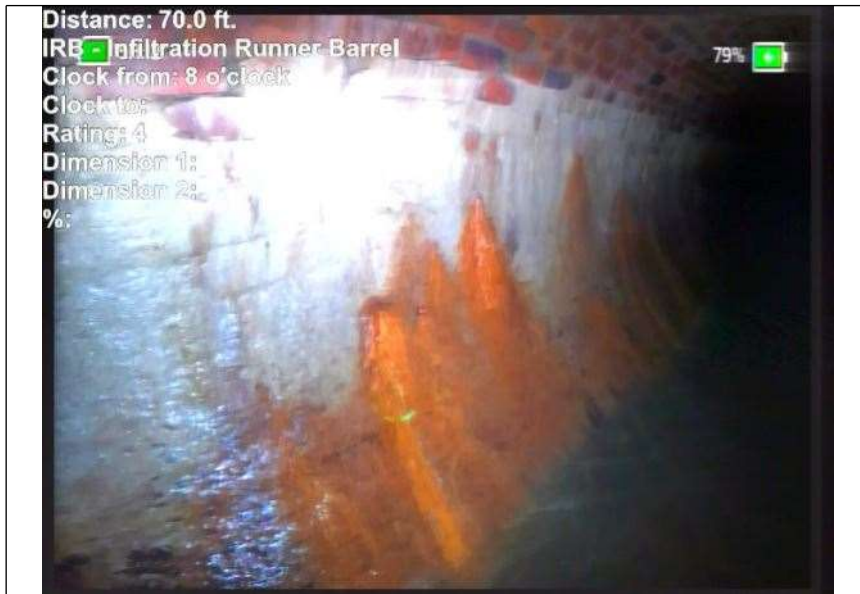
At: 70 ft. 8/. IRB - Infiltration Runner Barrel
