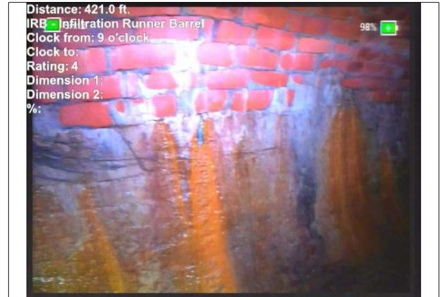
At: 421 ft. 9/. IRB - Infiltration Runner Barrel Joint: No
