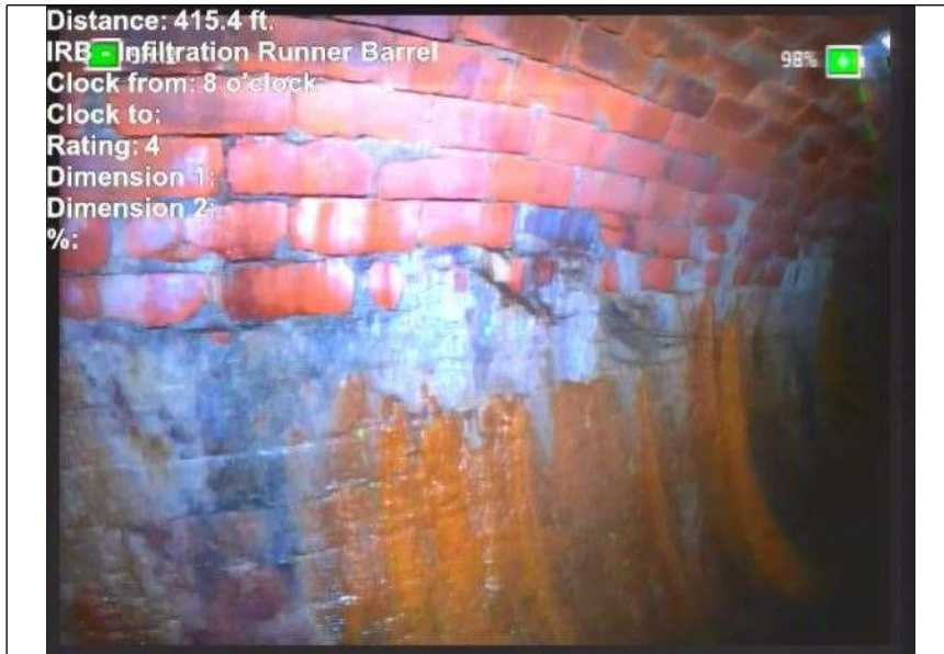
At: 415. IRB - Infiltration Runner Barrel 3999938964 84 ft. 8/.
