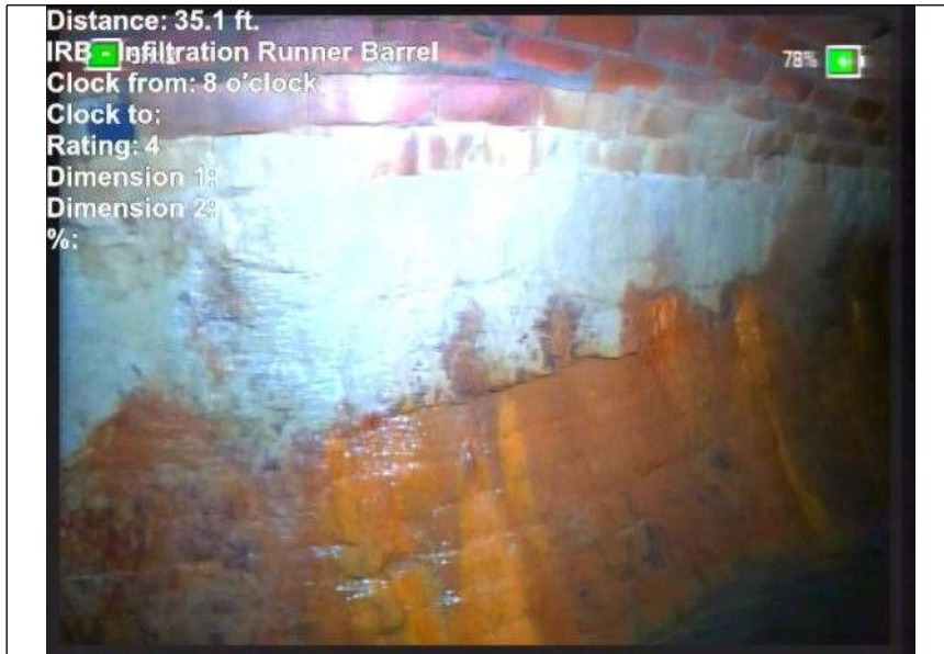
At: 35. IRB - Infiltration Runner Barrel 0999984741 211 ft. 8/.
