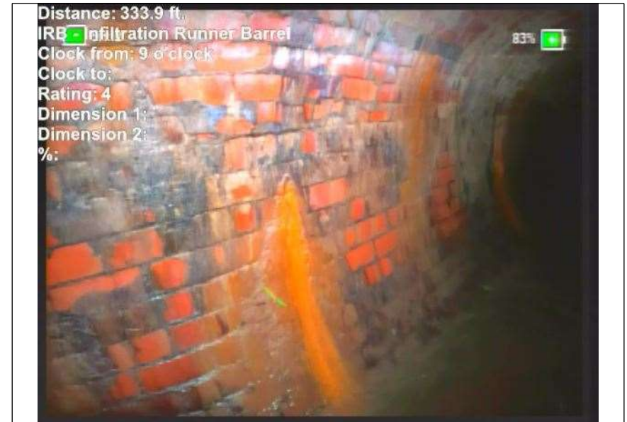
At: 333. IRB - Infiltration Runner Barrel 8999938964 84 ft. 9/ Joint: No
