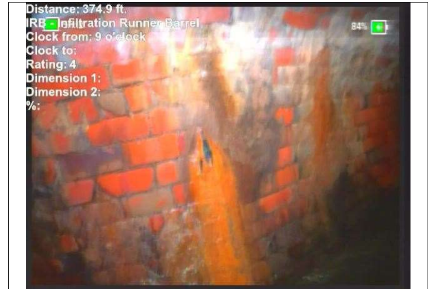
At: 374. IRB - Infiltration Runner Barrel 8999938964 84 ft. 9/.
