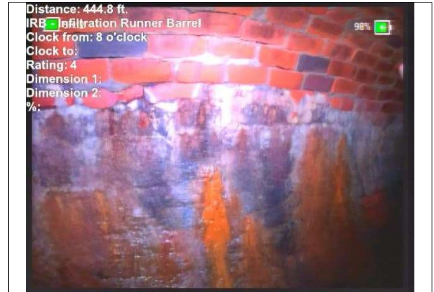
At: 444. IRB - Infiltration Runner Barrel 7999877929 69 ft. 8/.
