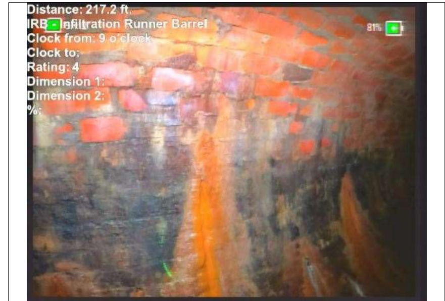
At: 217. IRB - Infiltration Runner Barrel 1999969482 42 ft. 9/.
