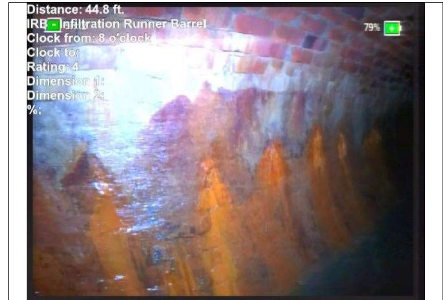
At: 44. IRB - Infiltration Runner Barrel 7999992370 605 ft. 8/.
