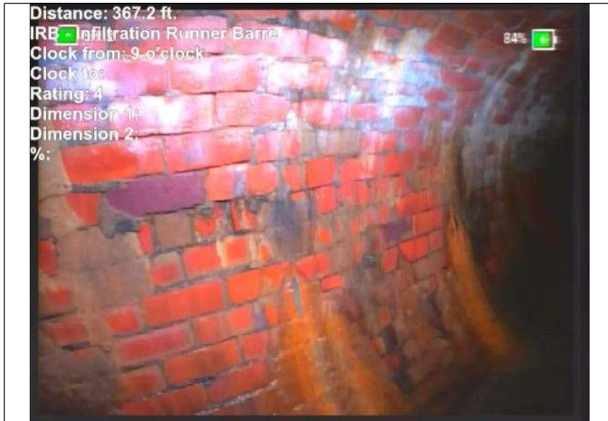
At: 367. IRB - Infiltration Runner Barrel 2000122070 31 ft. 9/.
