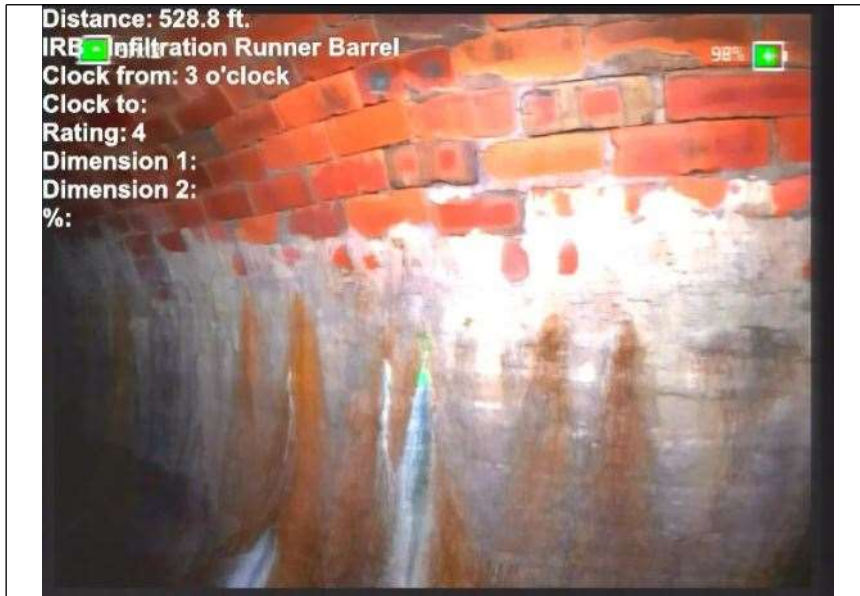
At: 528. IRB - Infiltration Runner Barrel 7999877929 69 ft. 3/.
