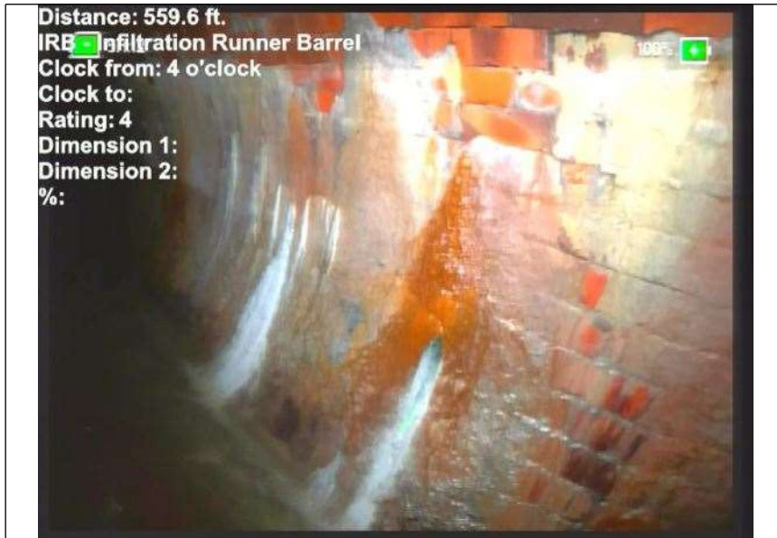
At: 559. IRB - Infiltration Runner Barrel 5999755859 38 ft. 4/.
