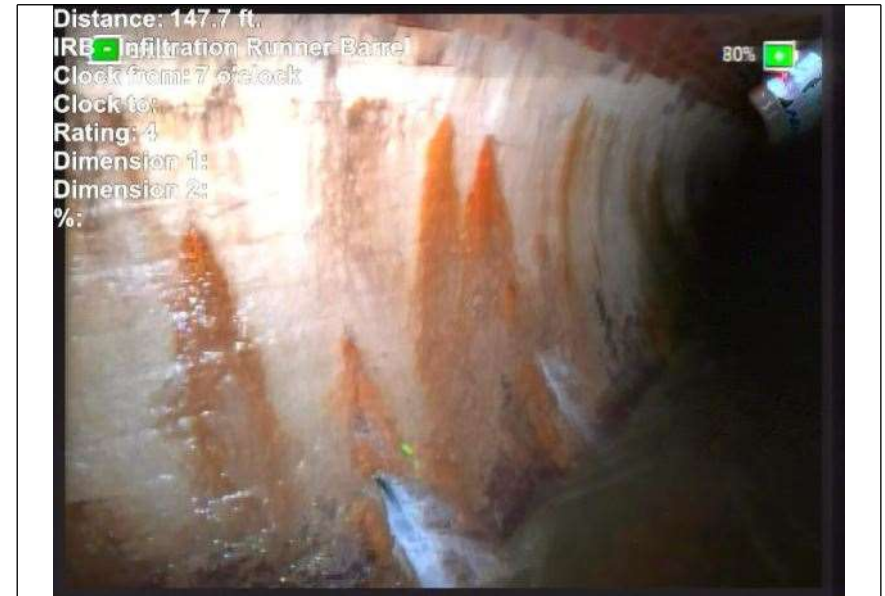
At: 147. IRB - Infiltration Runner Barrel 6999969482 42 ft. 7/.
