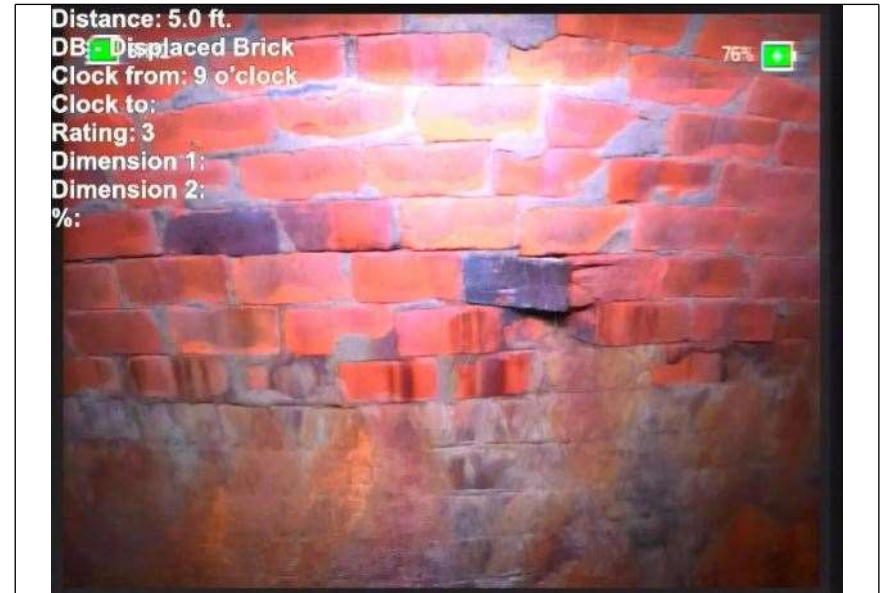
At: 5 ft. 9/. DB - Displaced Brick Joint: No
