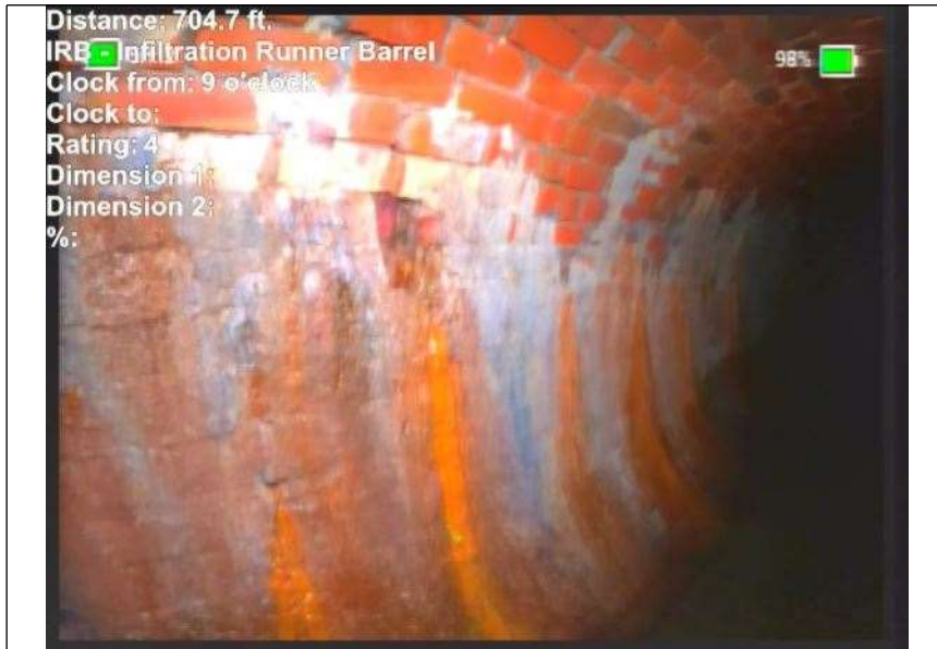
At: 704. IRB - Infiltration Runner Barrel 7000122070 31 ft. 9/.
