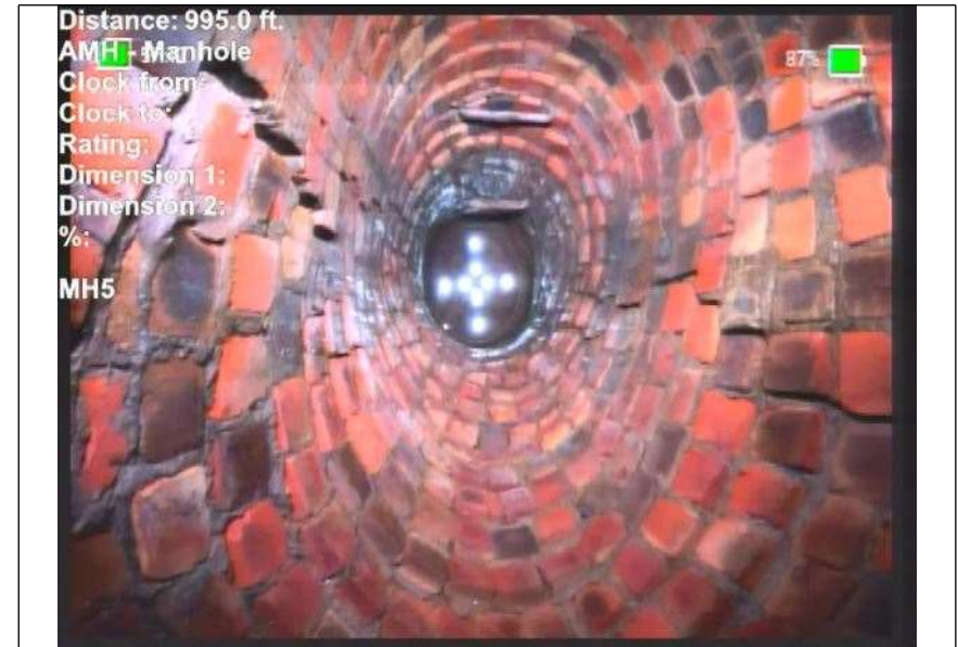
At: 995 ft. AMH - Manhole Joint: No MH5
