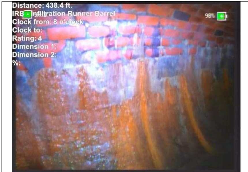
At: 438. IRB - Infiltration Runner Barrel 3999938964 84 ft. 8/.
