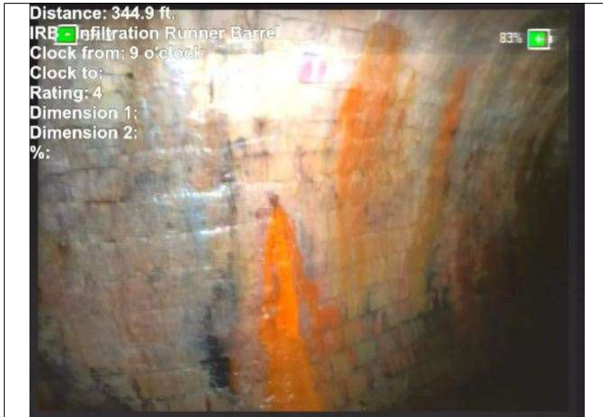
At: 344. IRB - Infiltration Runner Barrel 8999938964 84 ft. 9/.
