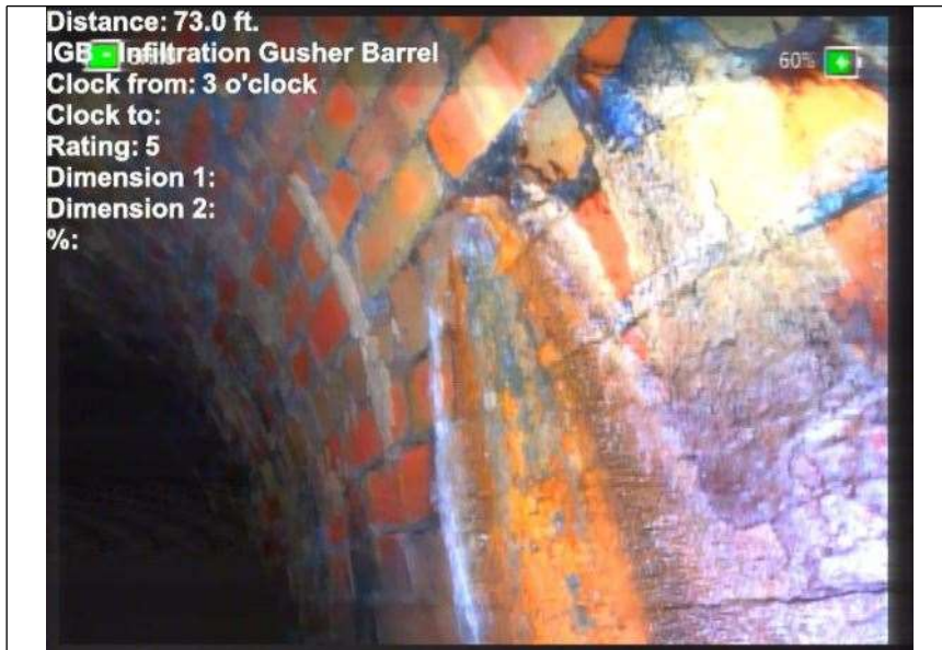
At: 73 ft. 3/. IGB - Infiltration Gusher Barrel
