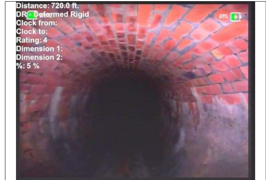
At: 720 ft. DR - Deformed Rigid Joint: No 5 %
