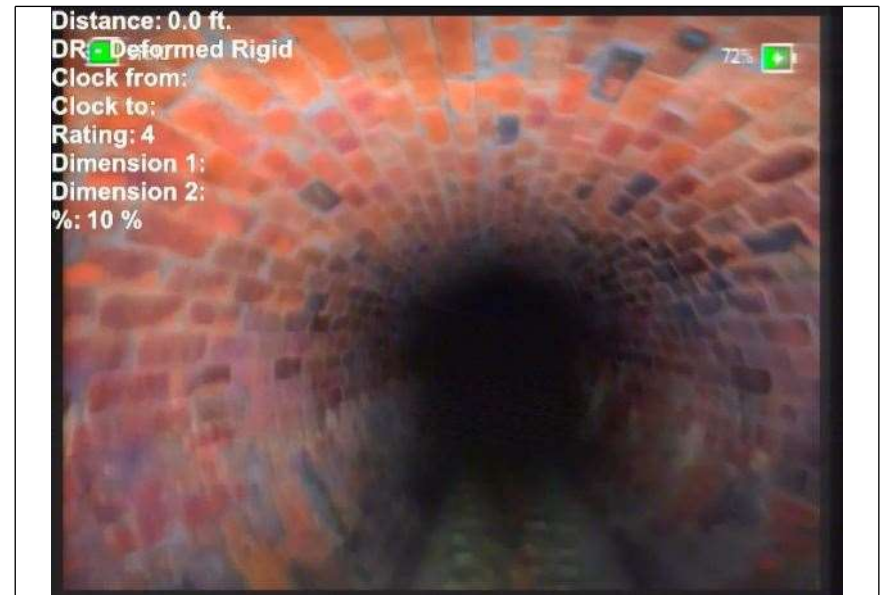
At: 0 ft. DR - Deformed Rigid Joint: No 10 %
