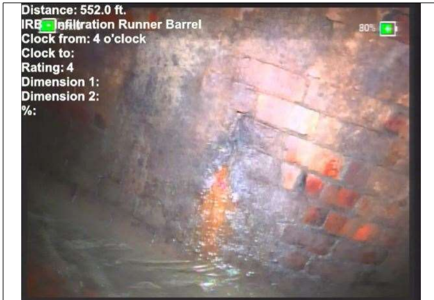
At: 552 ft. 4/. IRB - Infiltration Runner Barrel
