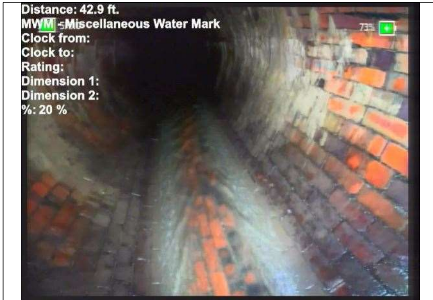
At: 42. MWM - Miscellaneous Water Mark 9000015258 789 ft.
