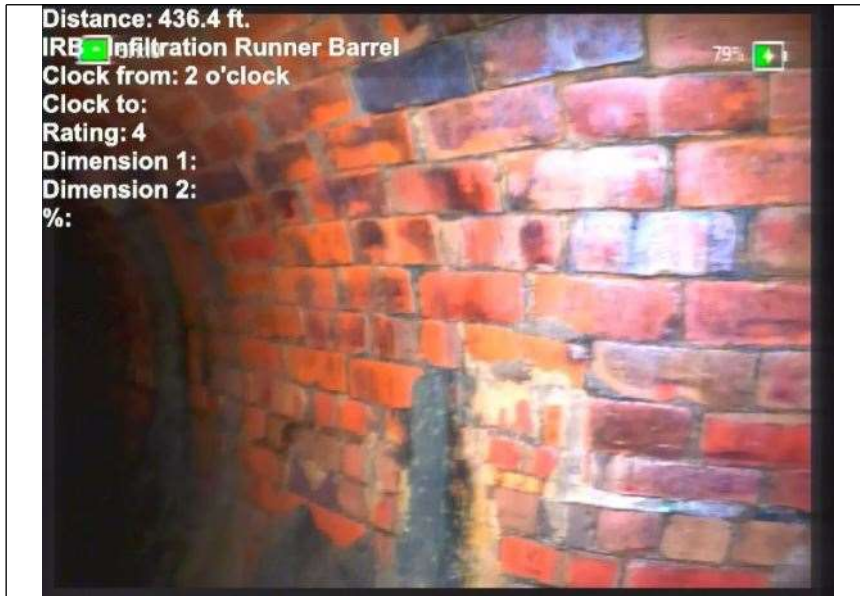
At: 436. IRB - Infiltration Runner Barrel 3999938964 84 ft. 2/.
