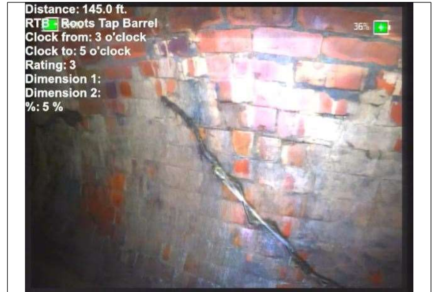
At: 145 ft. 3/5 RTB - Roots Tap Barrel Joint: No 5 %
