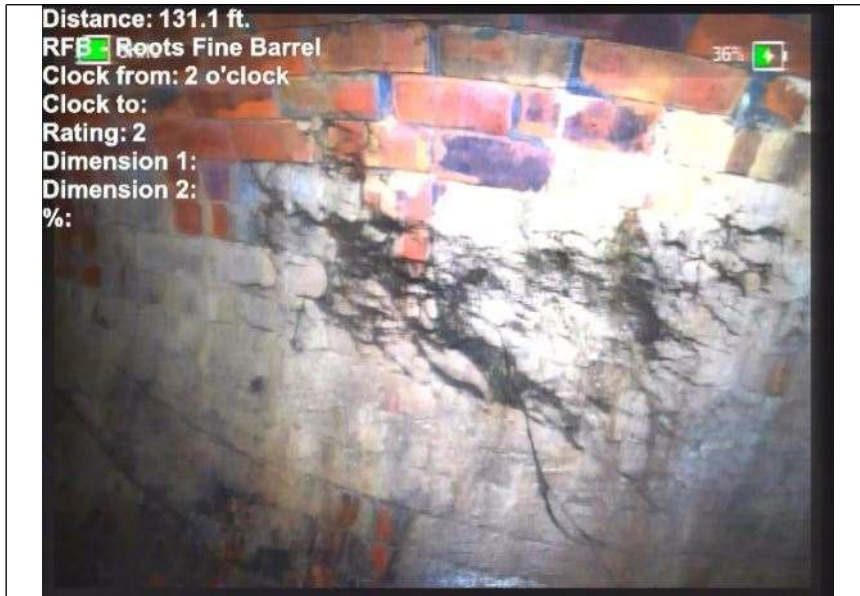
At: 131. RFB - Roots Fine Barrel 1000061035 16 ft. 2/. Joint: No
