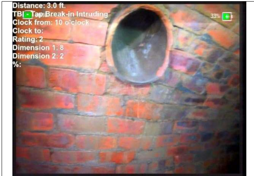
At: 3 ft. 10/ TBI - Tap Break-in Intruding Joint: No
