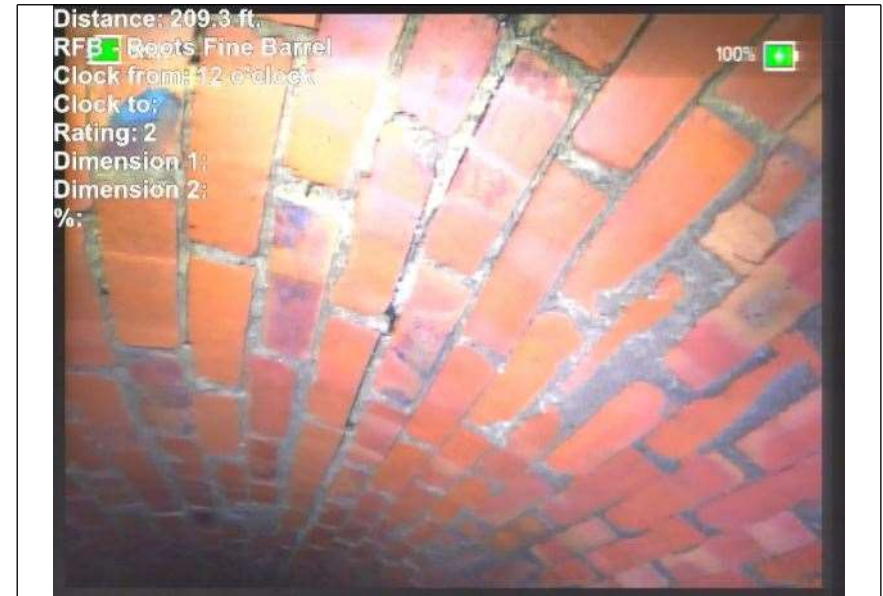
At: 209. RFB - Roots Fine Barrel 3000030517 58 ft. 12/.
