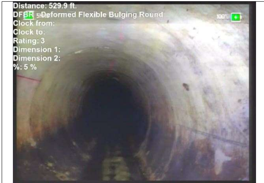
At: 529.9000244140 DFBR - Deformed Flexible Bulging Round 63 ft.
