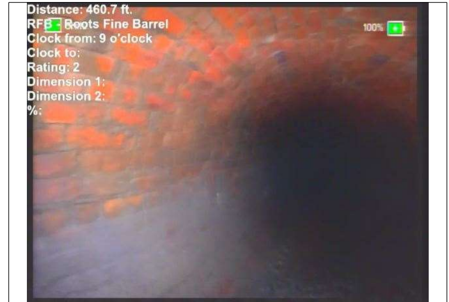
At: 460. RFB - Roots Fine Barrel 7000122070 31 ft. 9/. Joint: No
