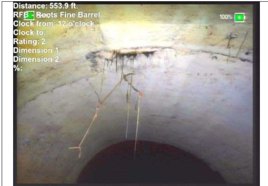
At: 553. RFB - Roots Fine Barrel 9000244140 63 ft. 12/.
