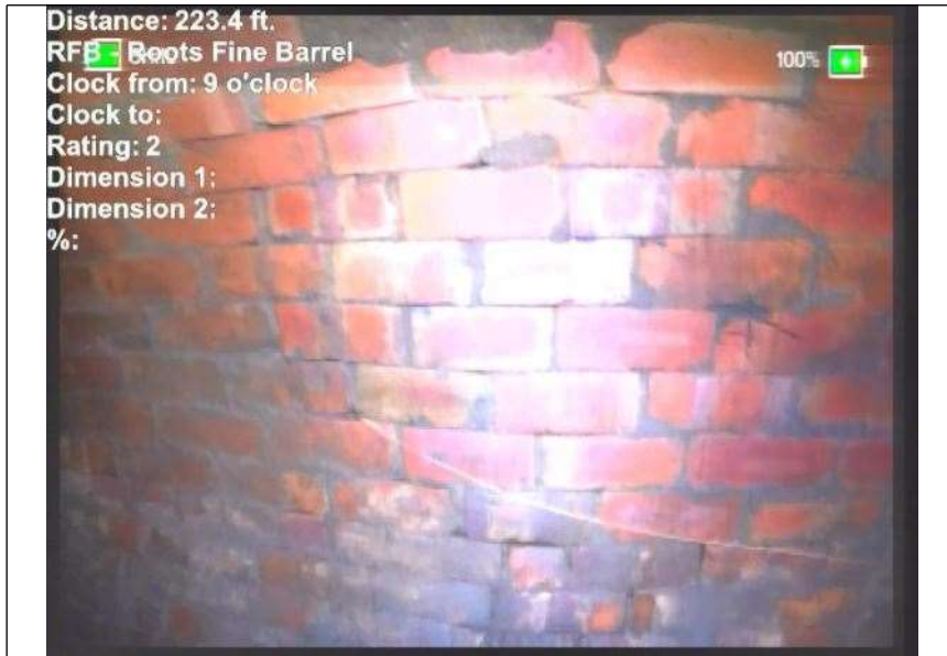
At: 223. RFB - Roots Fine Barrel 3999938964 84 ft. 9/.
