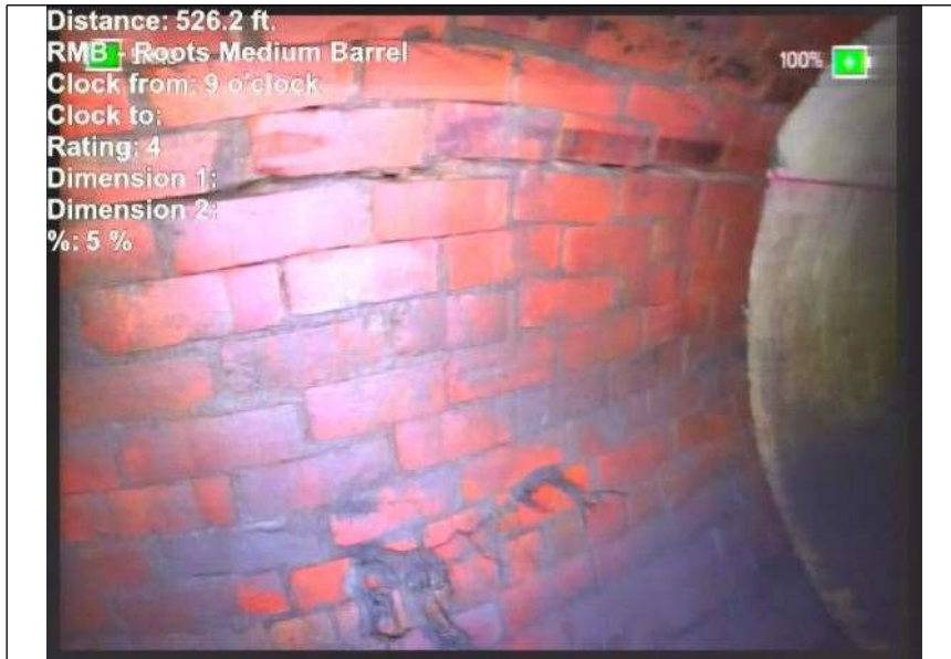
At: 526. RMB - Roots Medium Barrel 2000122070 31 ft. 9/.
