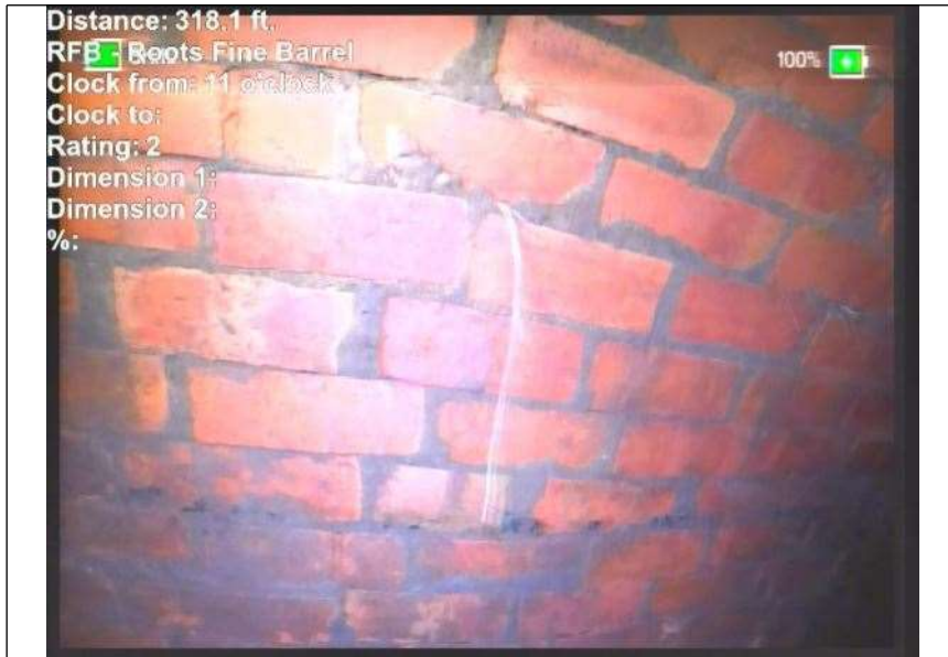
At: 318. RFB - Roots Fine Barrel 1000061035 16 ft. 11/. Joint: No
