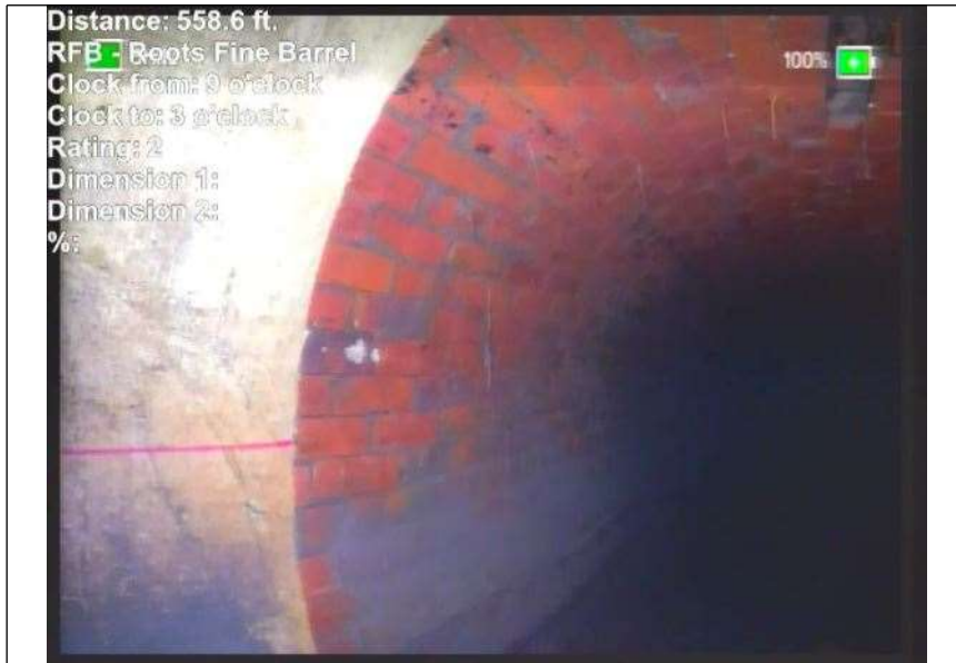
At: 558. RFB - Roots Fine Barrel 5999755859 38 ft. 9/3
