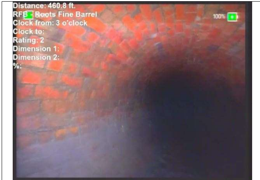
At: 460. RFB - Roots Fine Barrel 7999877929 69 ft. 3/.
