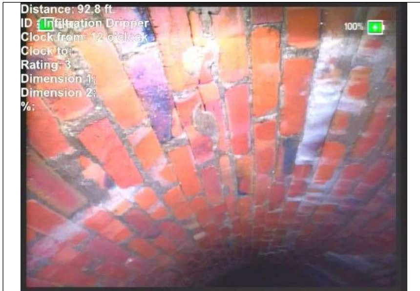
At: 92. ID - Infiltration Dropper 8000030517 578 ft. 12/.
