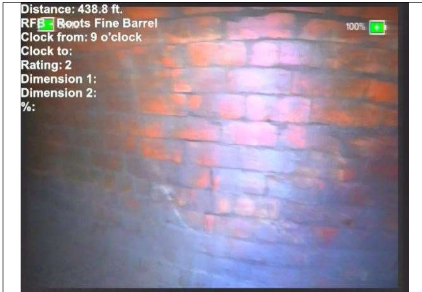
At: 438. RFB - Roots Fine Barrel 7999877929 69 ft. 9/.
