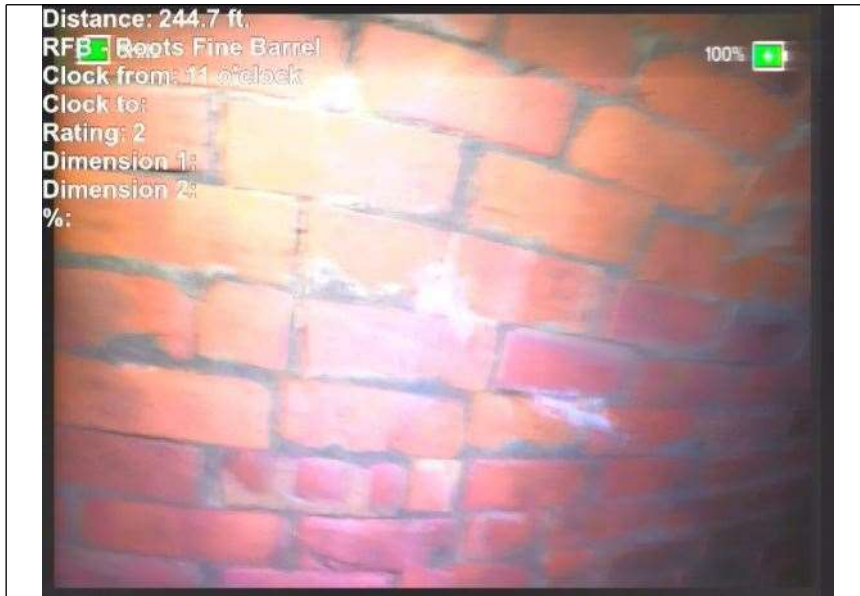
At: 244. RFB - Roots Fine Barrel 6999969482 42 ft. 11/.
