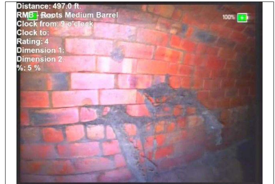
At: 497 ft. 9/. RMB - Roots Medium Barrel
