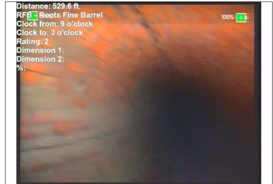
At: 529.6 ft. 9/3 RFB - Roots Fine Barrel
