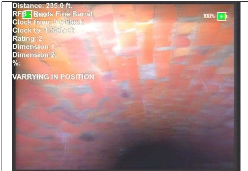
At: 235 ft. 9/1 RFB - Roots Fine Barrel
