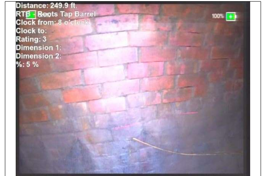
At: 249. RTB - Roots Tap Barrel 8999938964 84 ft. 8/.
