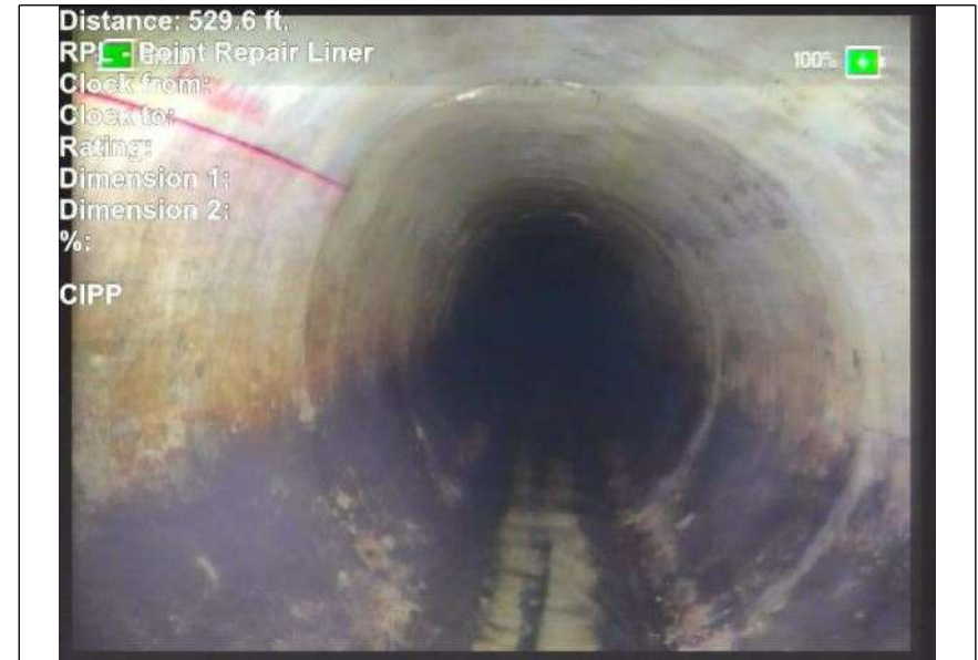
At: 529. RPL - Point Repair Liner 5999755859 38 ft.
