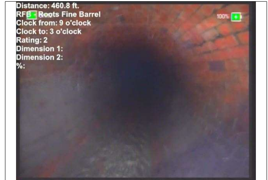
At: 460. RFB - Roots Fine Barrel 7999877929 69 ft. 9/3
