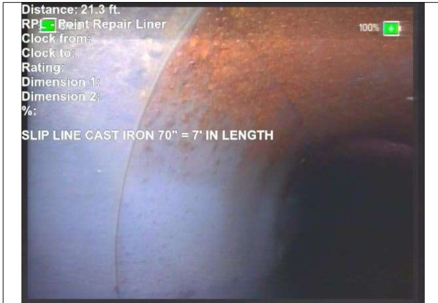
At: 21. RPL - Point Repair Liner 2999992370 605 ft.
