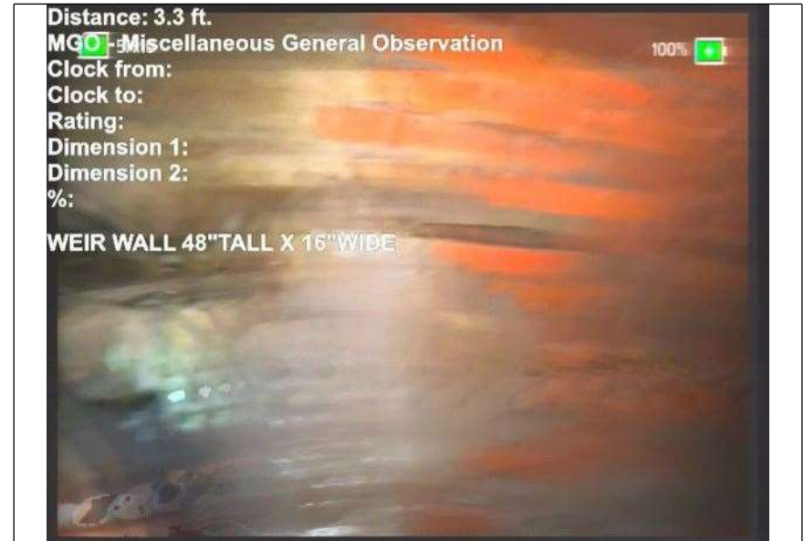
At: 3. 2999999523 1628 ft. Joint: No WEIR WALL 48" TALL X 16" WIDE
