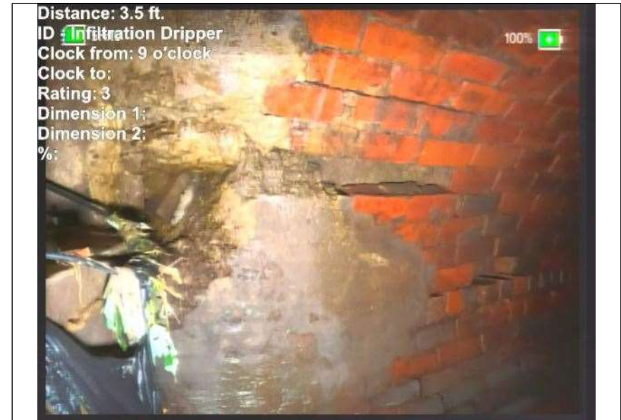
At: 3.5 ft. 9/. ID - Infiltration Dripper Joint: No
