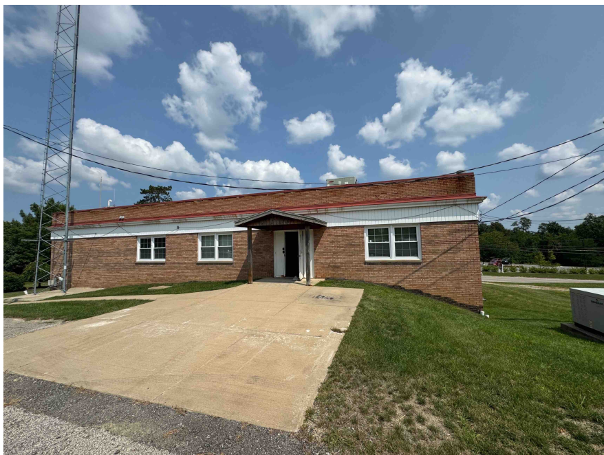
HA #13 Assumed Roofing System
