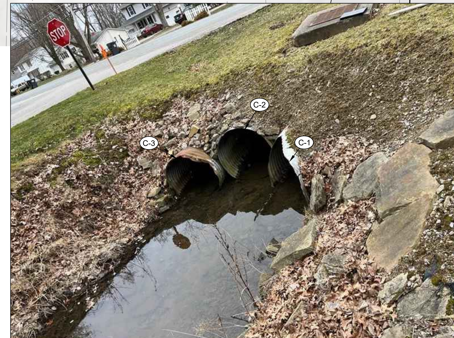
* PHOTO PER FIELD VISIT CONDUCTED BY CT CONSULTANTS ON 2/29/2024 (FACING WEST)
