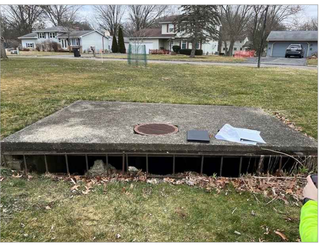
EXISTING JUNCTION CHAMBER
