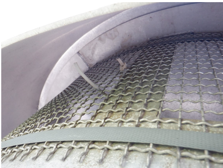
24) The external roof vent screen is intact.
