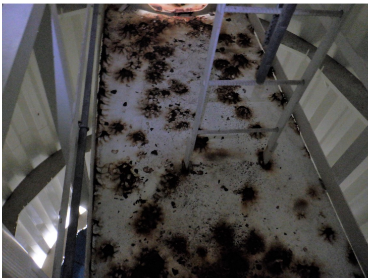
39) The top platform coating is in poor condition with numerous failures.
