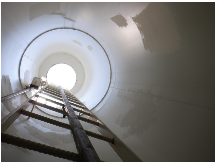
51) The access tube ladder is in good condition. The ladder is equipped with a fall prevention device.
