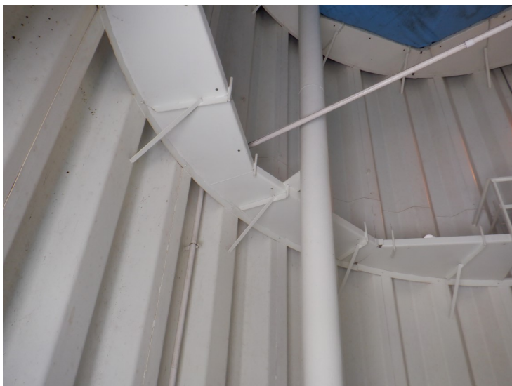
30) There is minor rust bleedthrough on the stiffeners below the condensate tarp in the dry interior.
