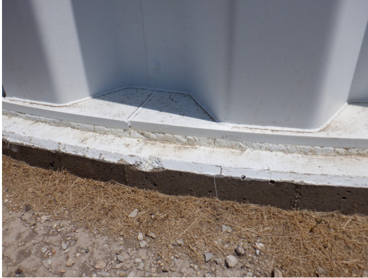
1) The concrete foundation is in good condition overall with some minor chips.
