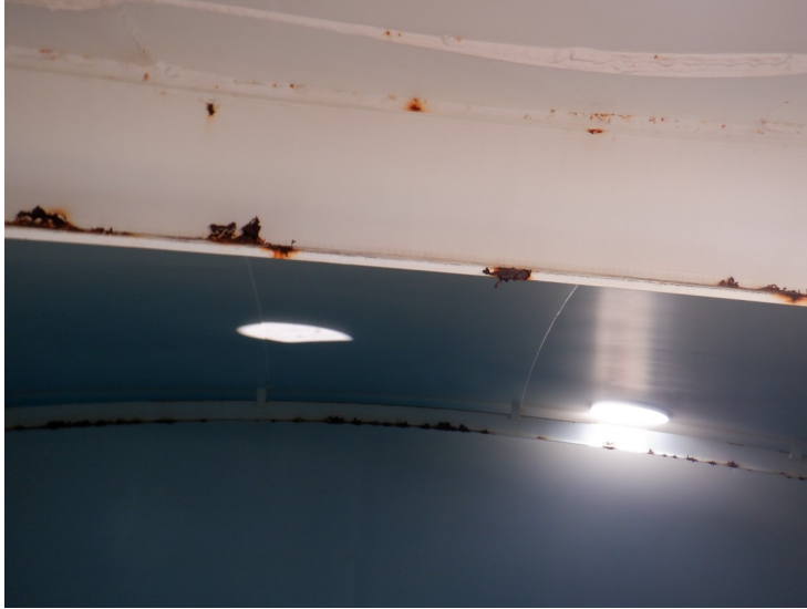
52) The wet interior roof coating is in fair condition overall with a few failures.
