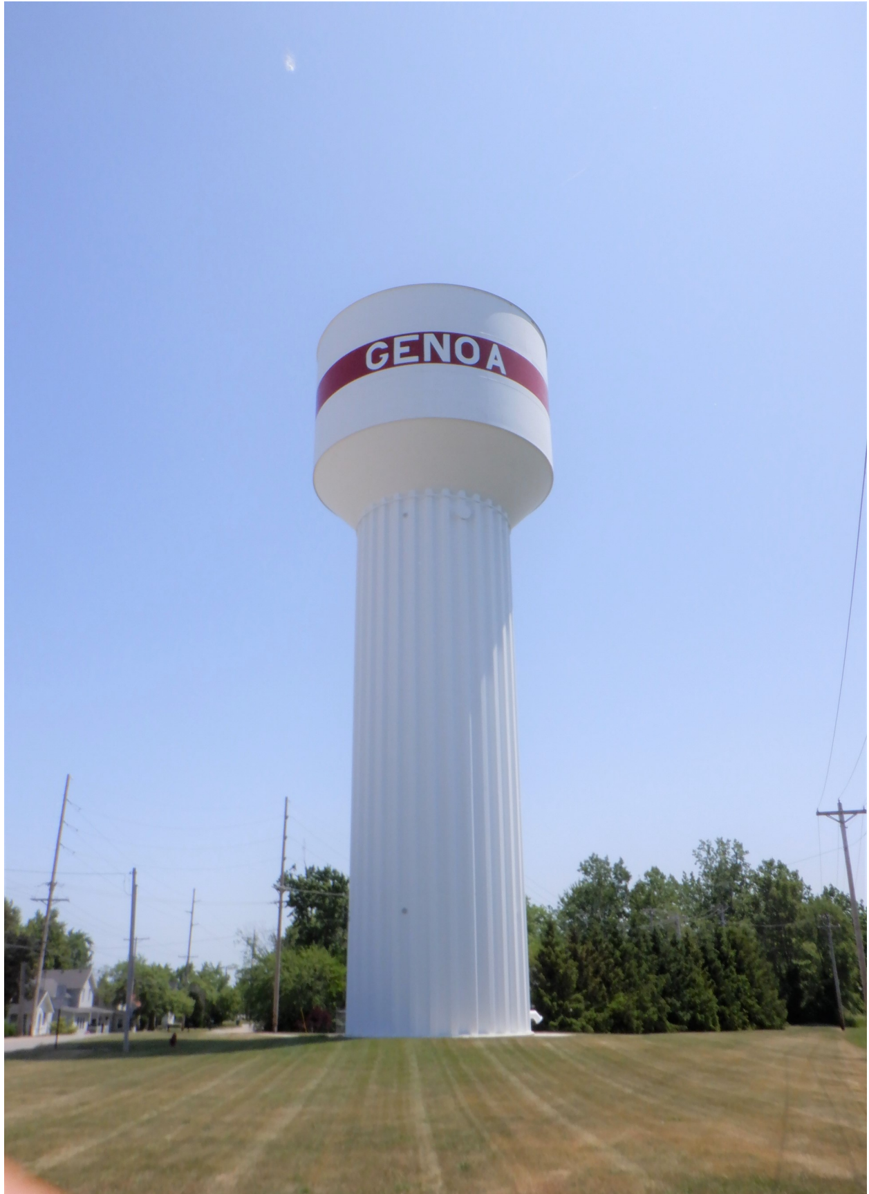
500,000 gallon fluted column elevated water storage tank owned by the City of Genoa, Ohio.
