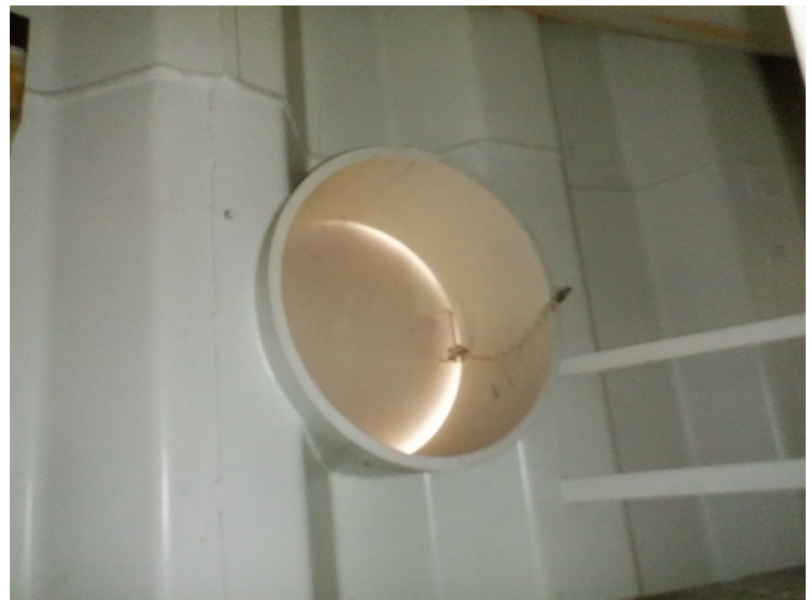
38) There is no handhold above the painter's hatch at the top of the column.
