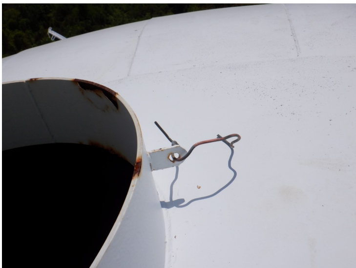
21) There is no gasket on the wet interior roof hatch.
