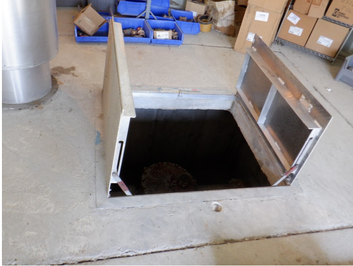
58) The metal hatch covering the pit is in good condition.
