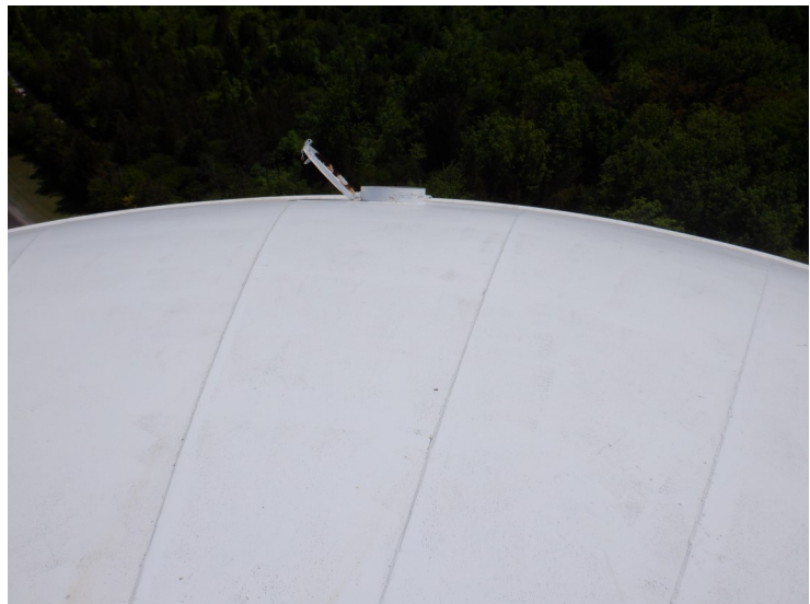
20) The secondary roof hatch was open upon inspection and not safely accessible.
