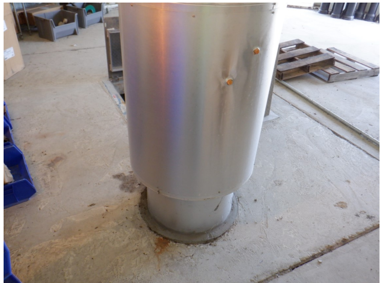
29) The expansion joint on the fill/draw pipe at the bottom of the column is covered with insulation and not accessible for inspection.
