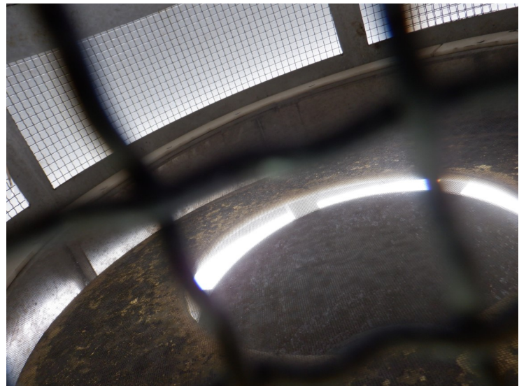
26) The interior roof vent screen is in good condition but oversized.
