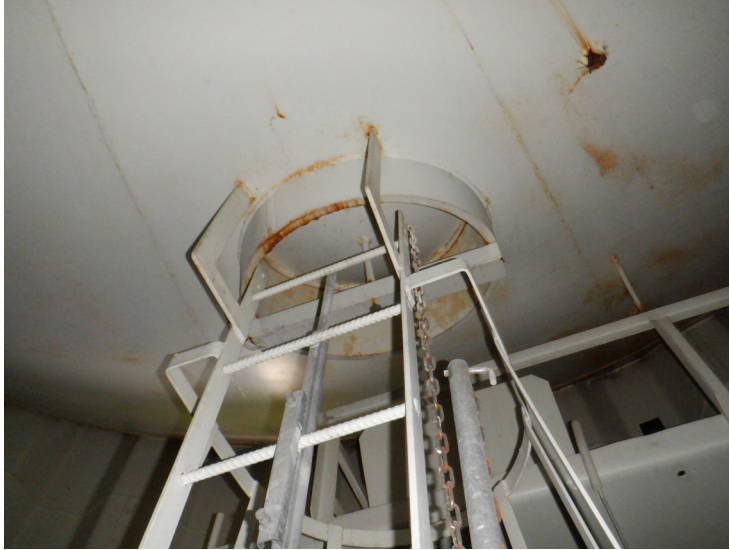
43) The wet interior manway in the bowl is in good condition. The ladder to the manway is equipped with a fall prevention device.
