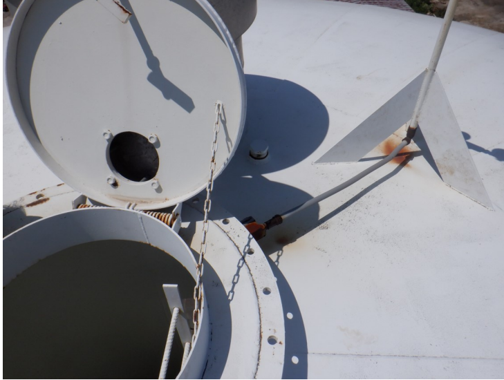
22) There is no handhold at the access tube roof hatch.
