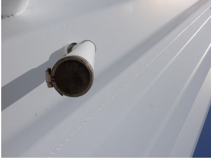
10) The condensate tarp drain pipe is screened on the exterior.
