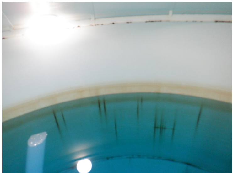
56) The wet interior sidewall coating is in poor condition with numerous failures.
