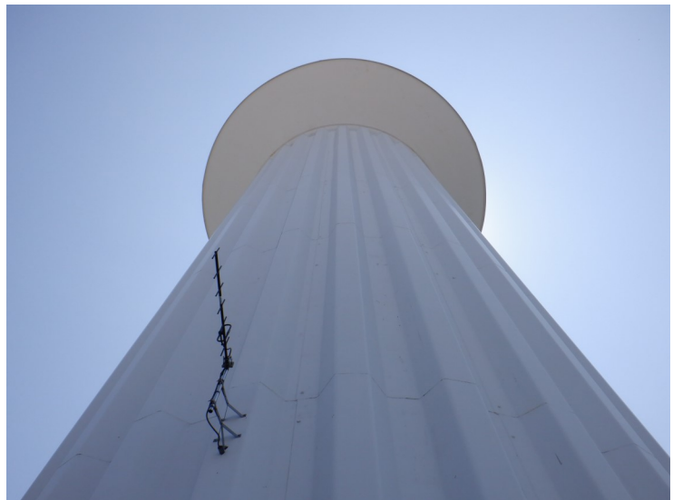
11) The bowl coating is in fair condition with a few areas of delaminated topcoat.
