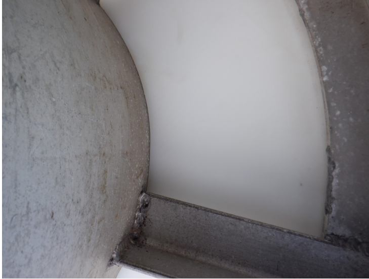
25) The roof vent pressure plate was found to be properly aligned.
