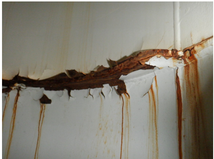
47) There is heavy corrosion on the access tube stiffeners.
