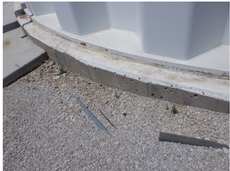
2) The grout between the steel baseplate and concrete foundation is intact.
