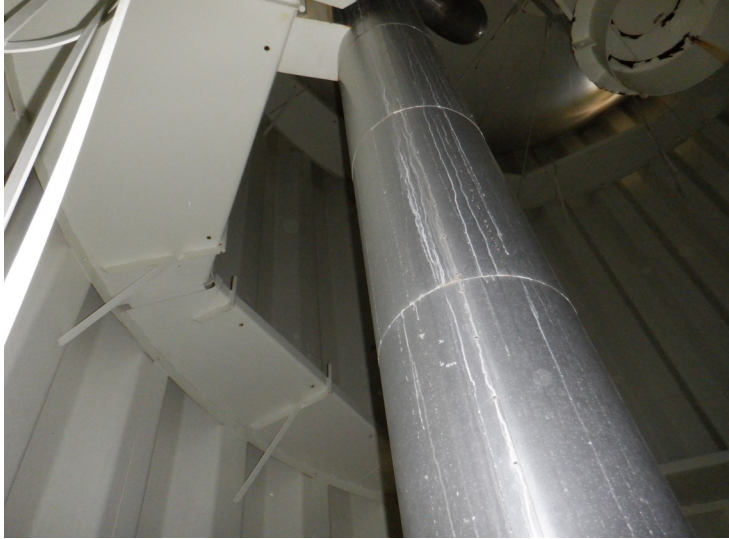
37) The insulation and aluminum cover on the fill/draw pipe is in good condition.
