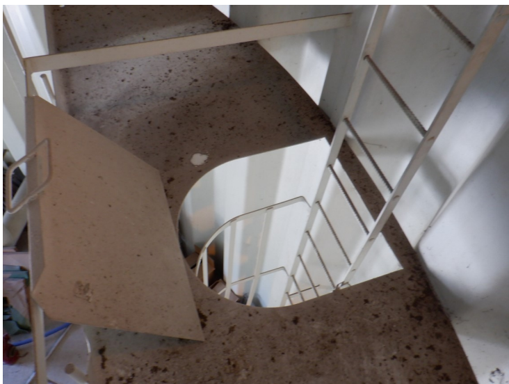
33) The ladder openings in the platform hatches are equipped with hinged covers.
