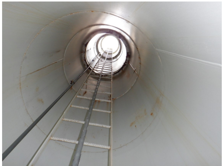
50) The access tube coating is in fair condition overall.
