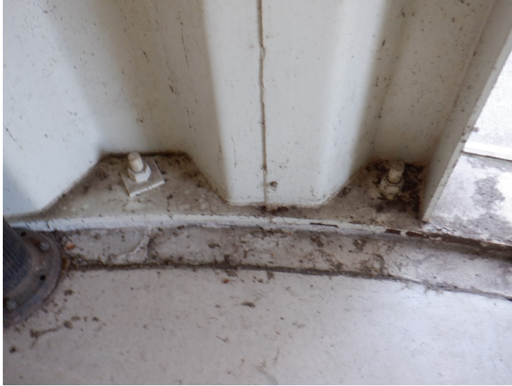
28) The anchor bolts in the dry interior are in good condition.
