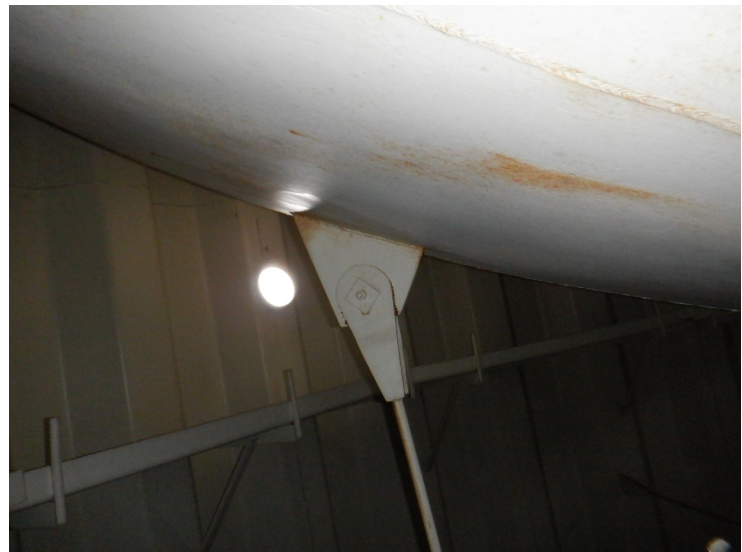
44) The bowl coating is in fair condition with a few failures.
