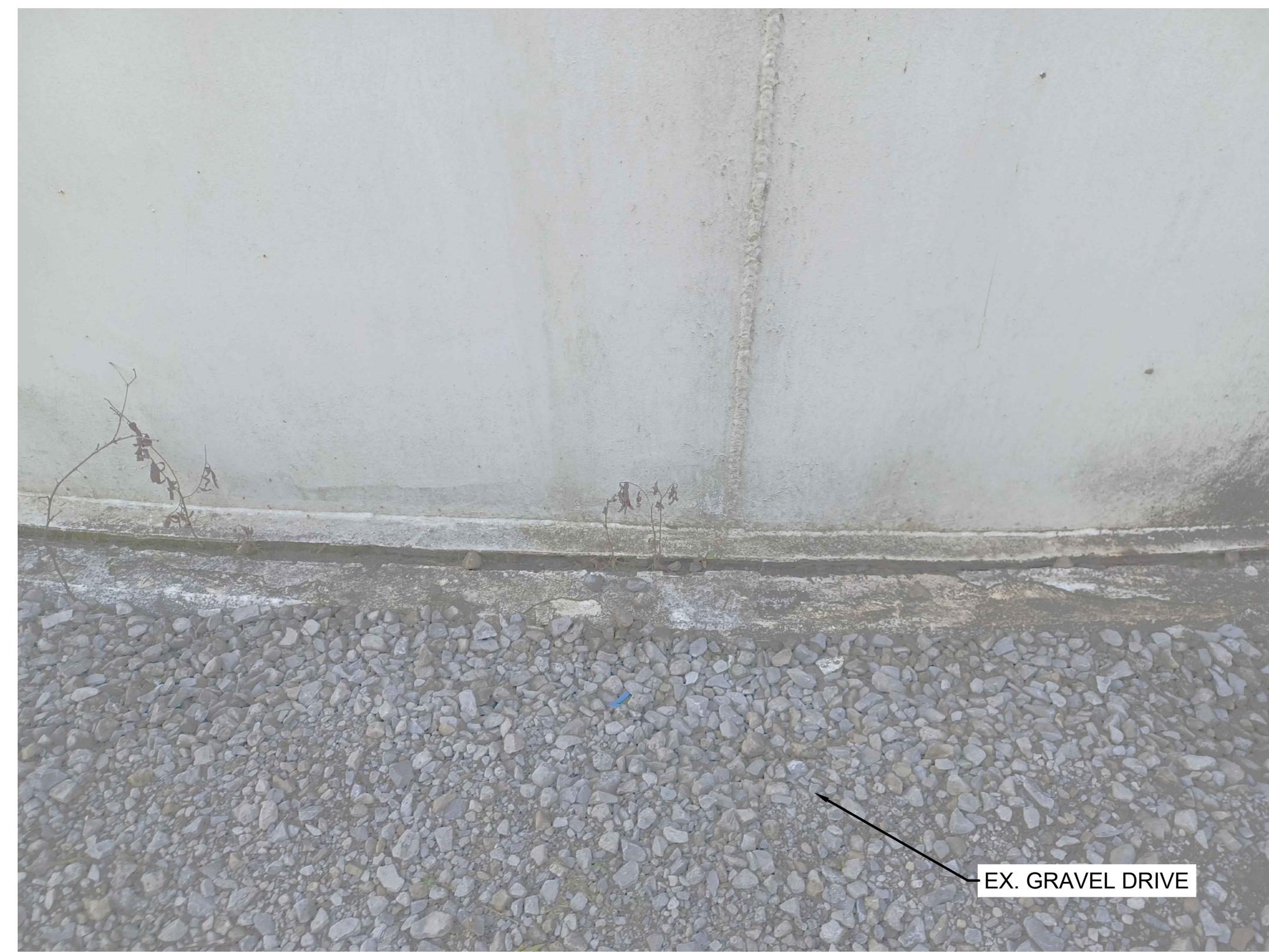
PHOTO 2 - PALMER AVE. TANK GROUT BETWEEN STEEL BASE AND FOUNDATION
