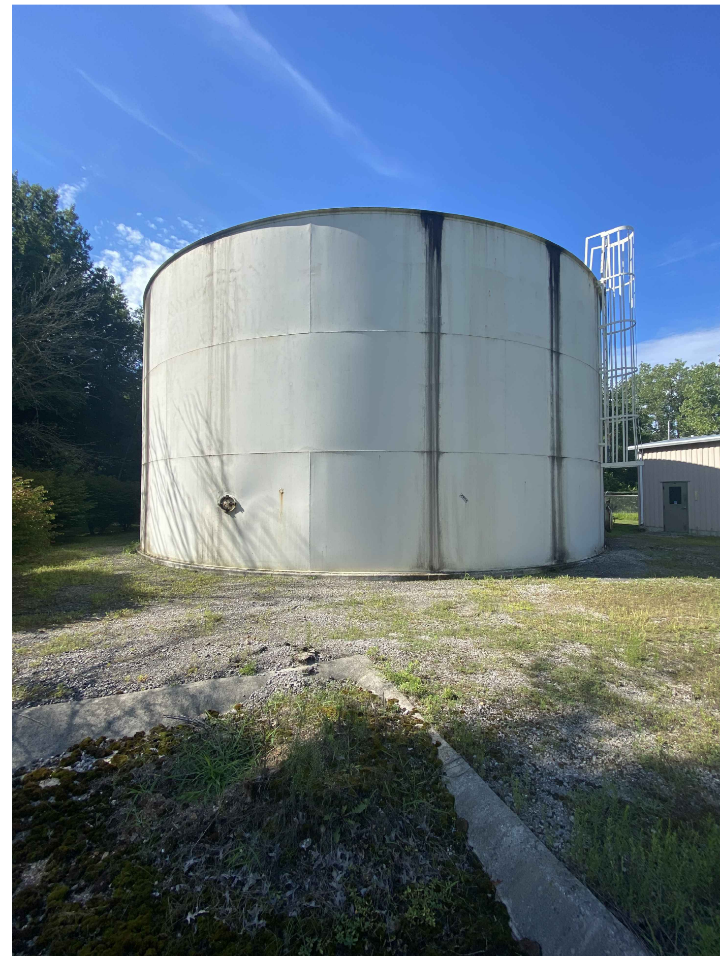
PHOTO 3 - PALMER AVE. TANK TANK SITE
