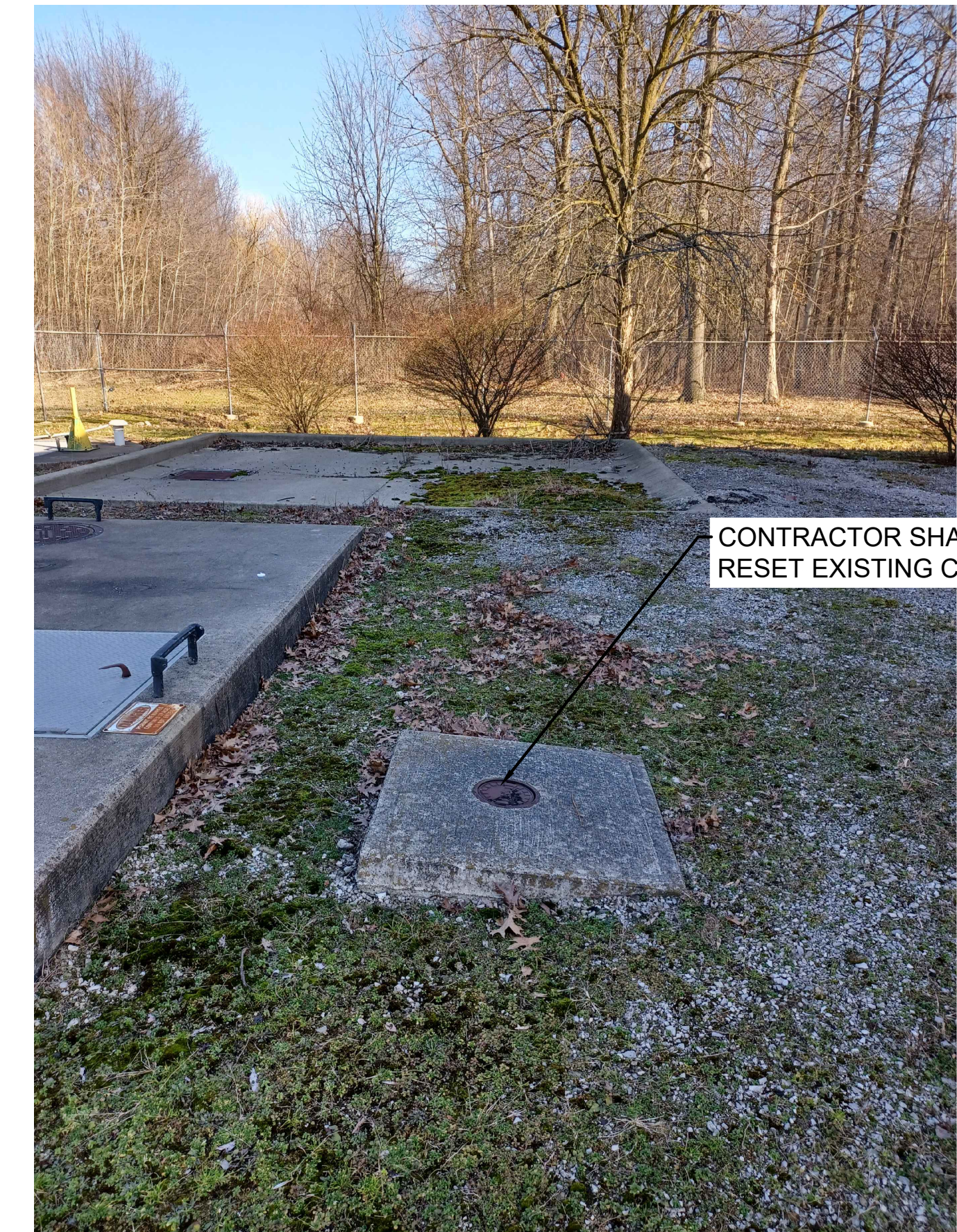
PHOTO 7 - PALMER AVE. TANK VALVE BOX
