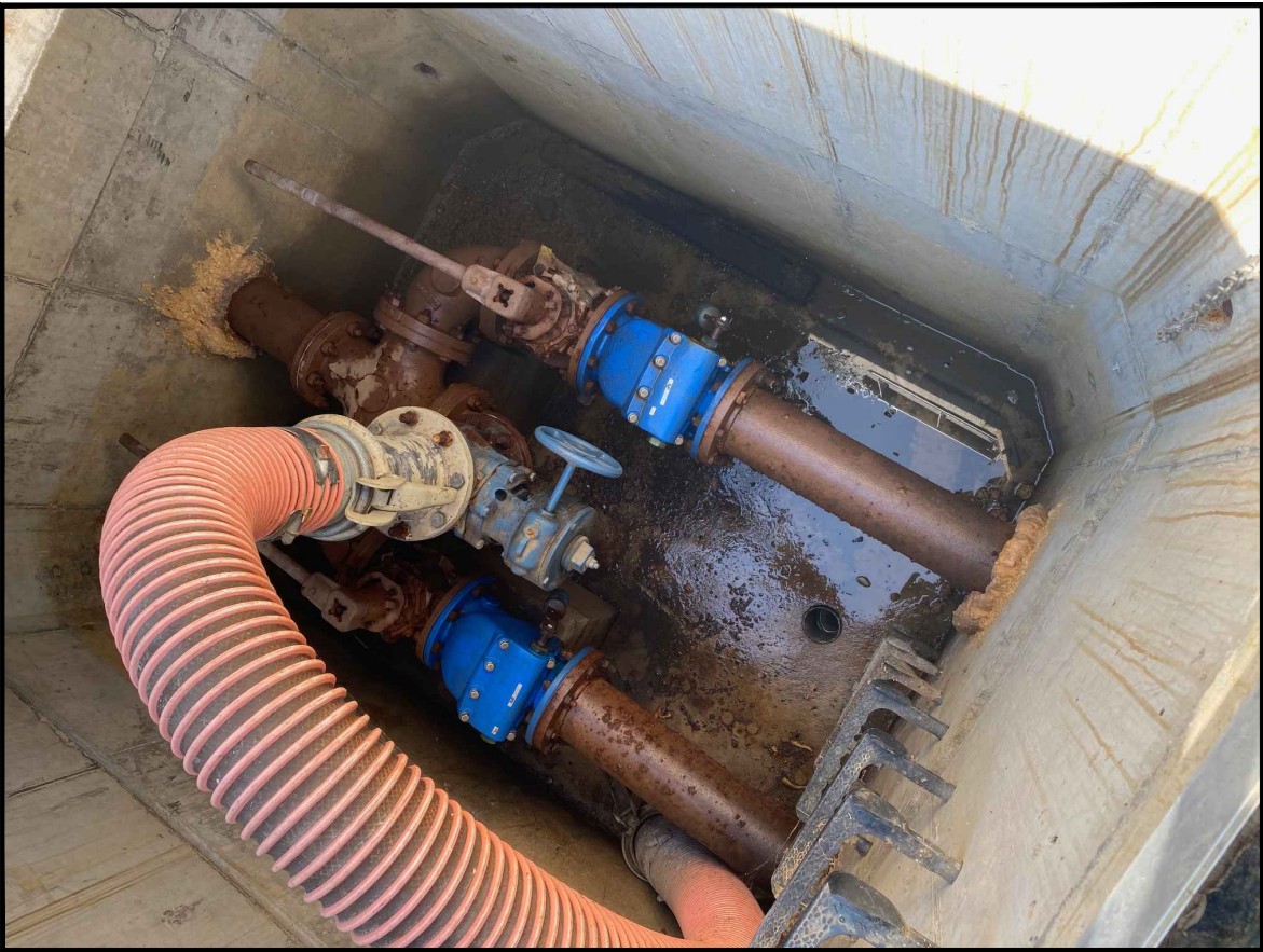
EXISTING 8-FT X 8-FT VALVE VAULT AND QUICK CONNECT HOSE
