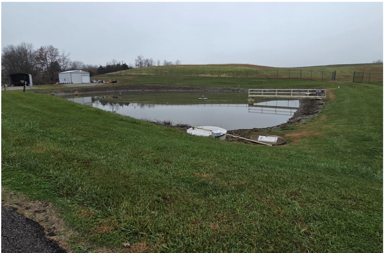
Figure 1. Project Location, looking north toward existing lagoon.
