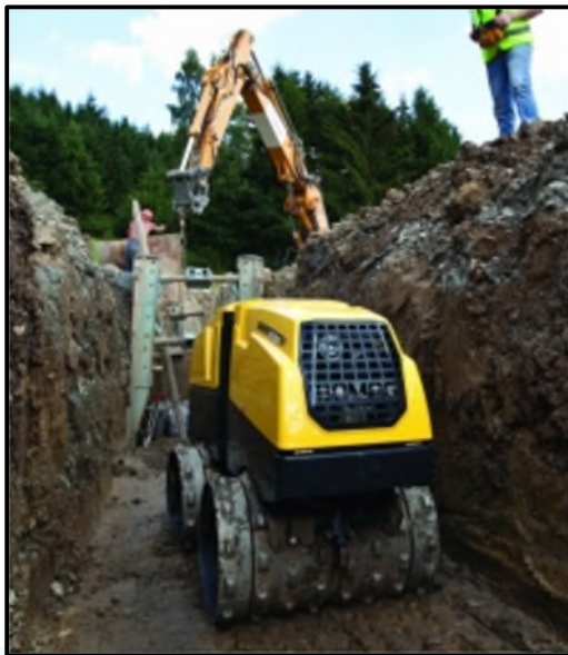
FIGURE NO. 1: Remote Controlled Sheepfoot Trench Compactor
