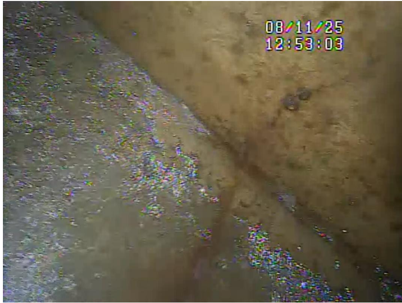
Fig. 3 crack in ceiling 50' E. of outlet structure 2025
