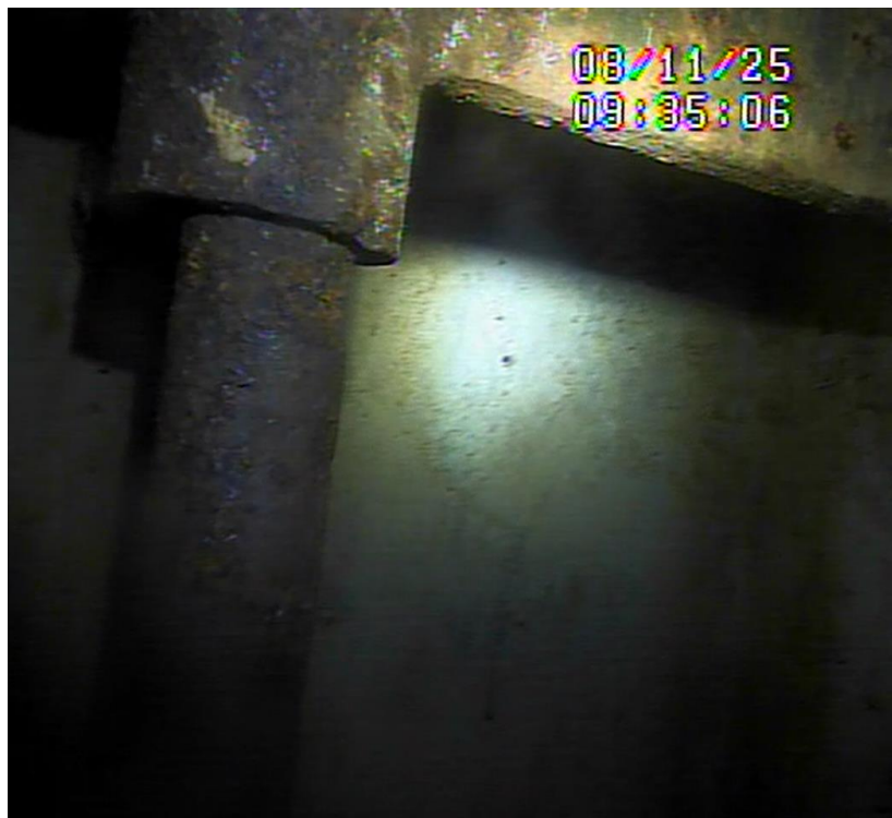
Fig. 6 Wear on Stem at Stem Guide 3
