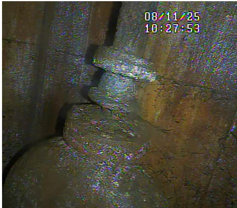
Fig. 7 Stem Attached to Gate valve
