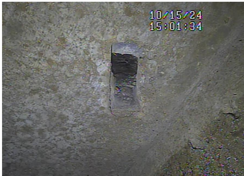
Fig. 2 2x4 void at 45' on outlet structure (no new photo)
