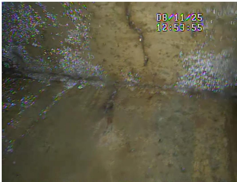
Fig. 4 crack in right wall at 65' E. of outlet structure 2025
