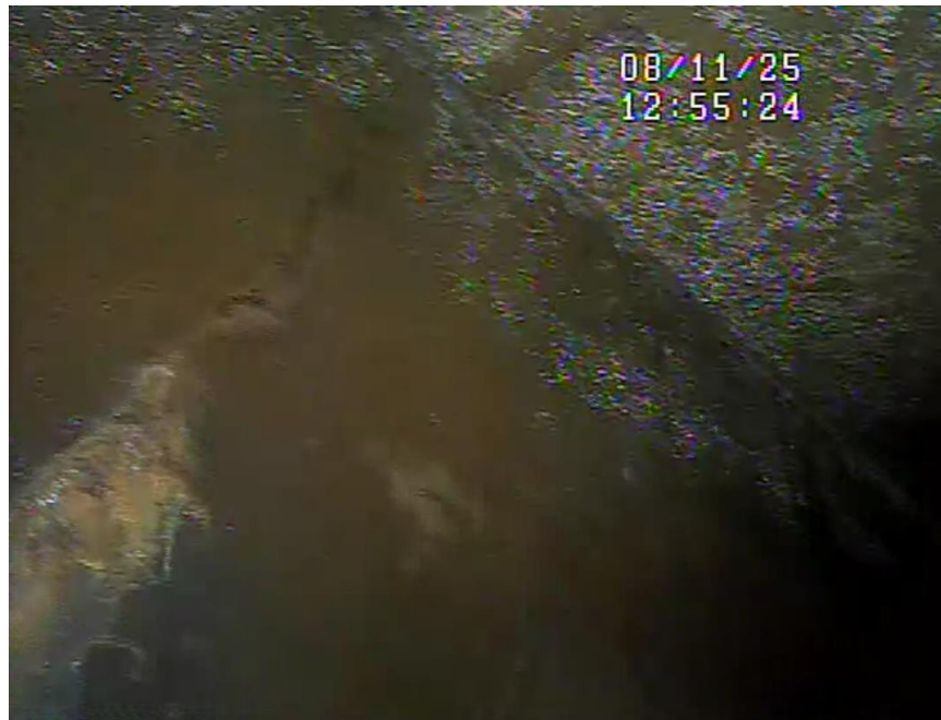
Fig. 5 crack in ceiling at 110' E. of outlet structure 2025
