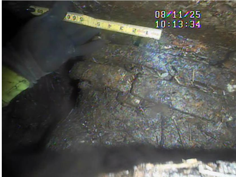
Fig. 9 Typical Condition of Gate Mounting Bolts
