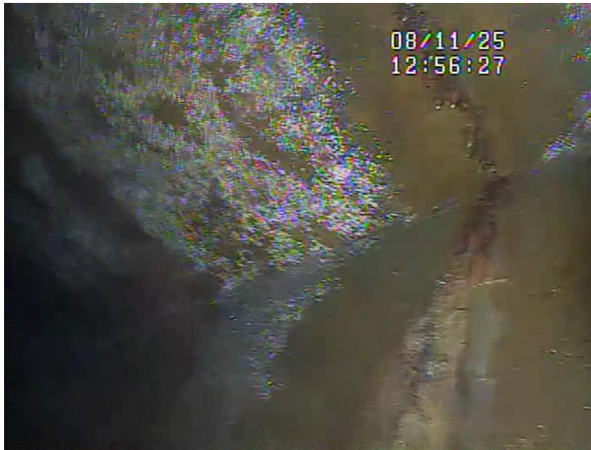
Fig. 7 crack in right wall 165' E. of outlet structure 2025
