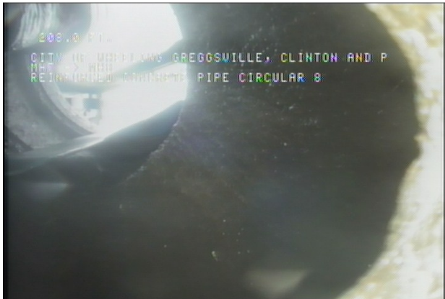
6, 00:11:06, 208.00ft Downstream Manhole, Survey Ends / MH8
