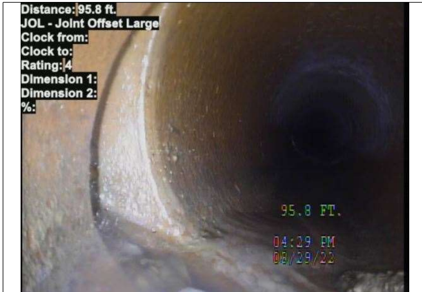
At: 95.8 ft. JOL - Joint Offset Large Joint: No
