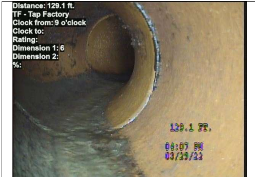
At: 129.1 ft. 9/. TF - Tap Factory Joint: No
