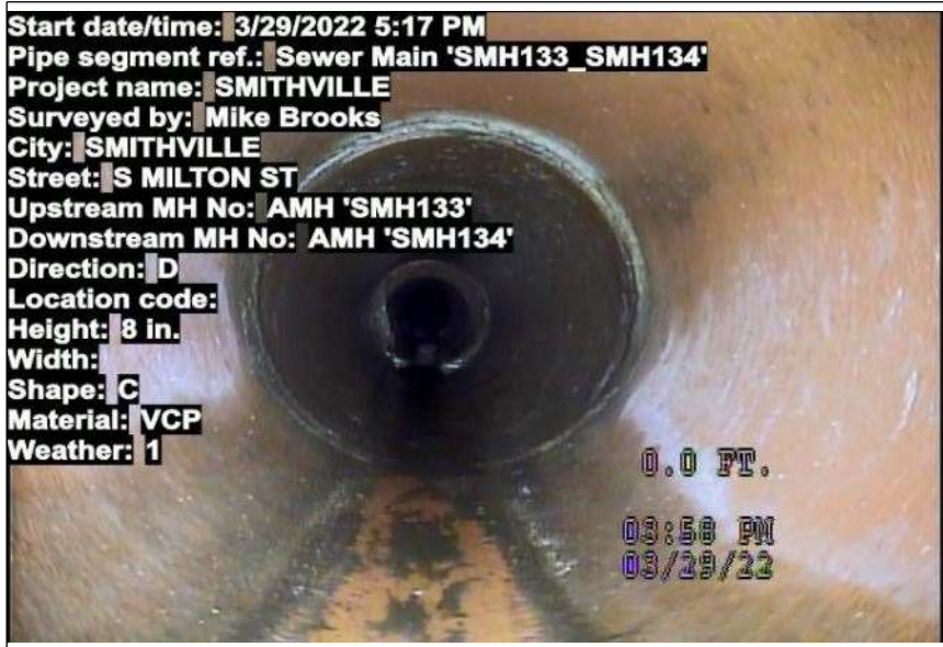
At: 0 ft. AMH - Manhole Joint: No SMH133
