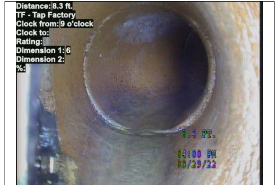
At: 8.3 ft. 9/. TF - Tap Factory Joint: No
