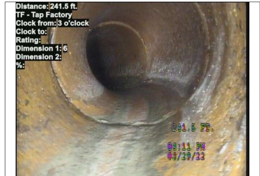
At: 241.5 ft. 3/. TF - Tap Factory Joint: No
