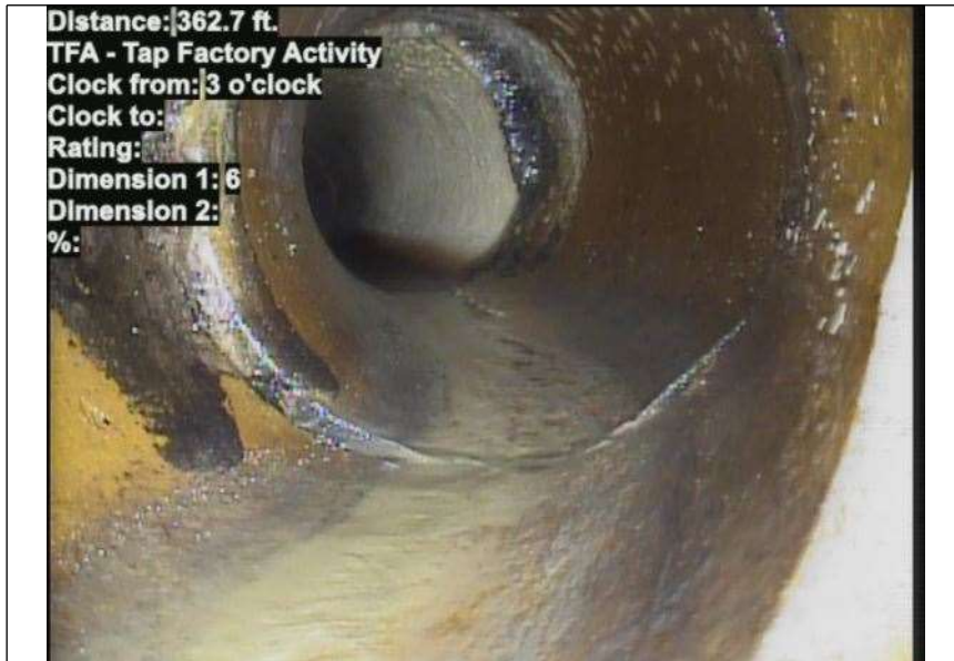
At: 362.7 ft. 3/. TFA - Tap Factory Activity Joint: No
