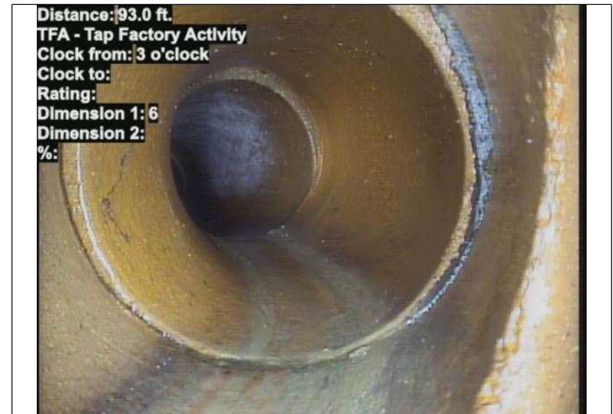
At: 93 ft. 3/ TFA - Tap Factory Activity Joint: No
