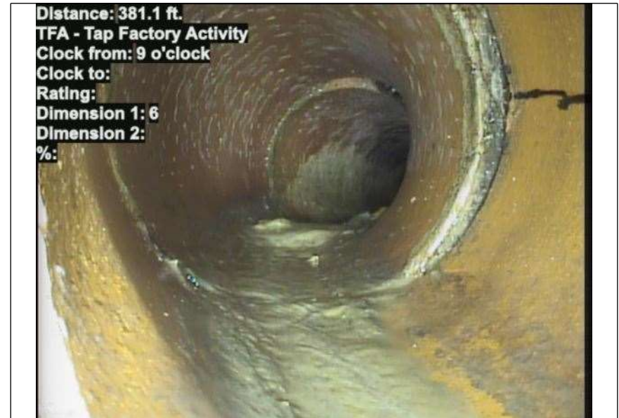
At: 381.1 ft. 9/. TFA - Tap Factory Activity Joint: No
