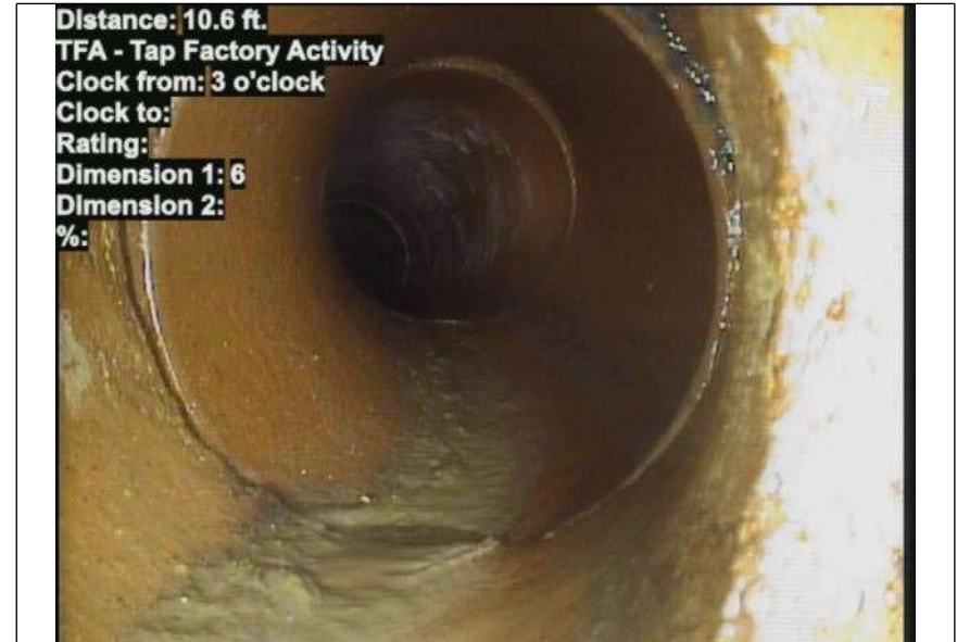
At: 10.6 ft. 3/. TFA - Tap Factory Activity Joint: No
