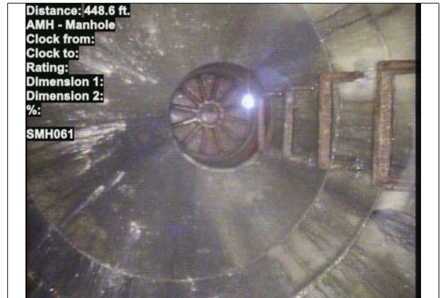
At: 448.6 ft. AMH - Manhole Joint: No SMH061
