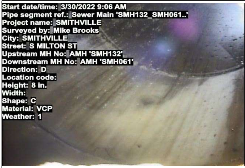
At: 0 ft. AMH - Manhole Joint: No SMH132
