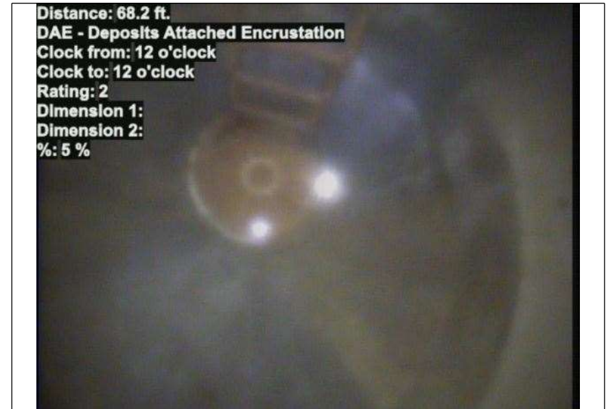
At: 68.2 ft. DAE - Deposits Attached Encrustation 12/12 Joint: No 5 %
