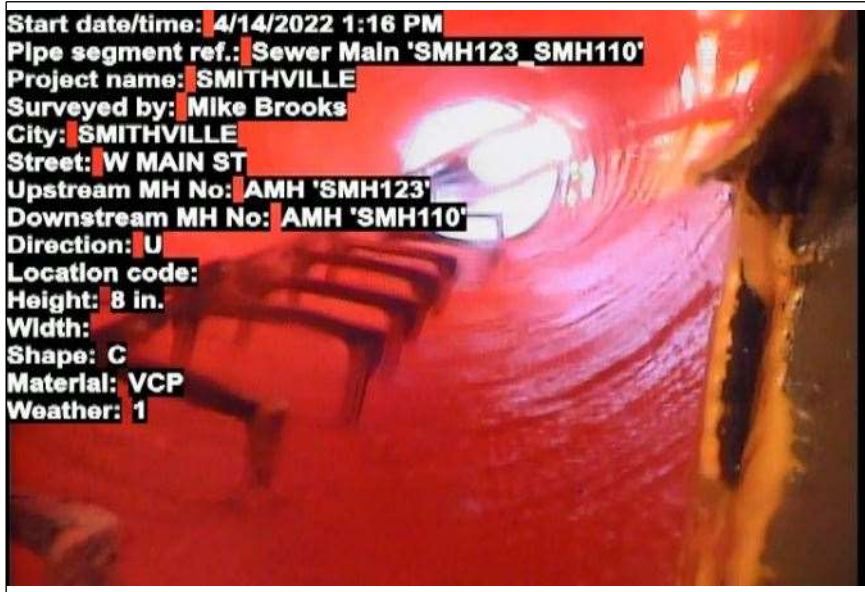
At: 0 ft. AMH - Manhole Joint: No SMH110
