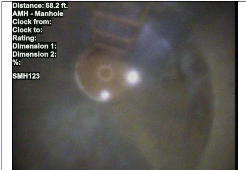
At: 68.2 ft. AMH - Manhole Joint: No SMH123
