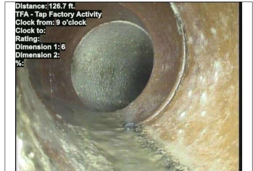
At: 126.7 ft. 9/. TFA - Tap Factory Activity Joint: No
