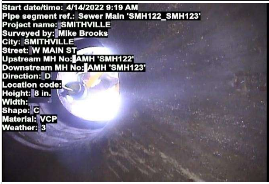
At: 0 ft. AMH - Manhole Joint: No SMH122
