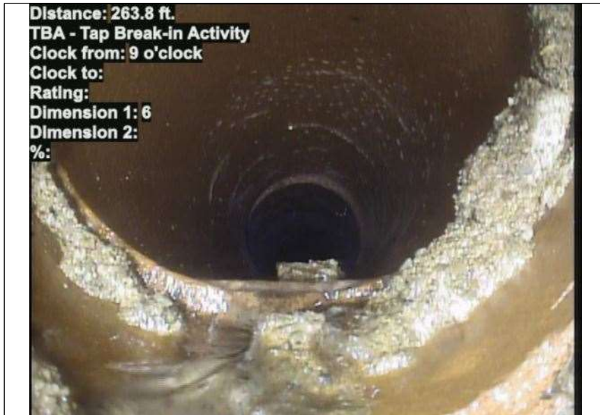
At: 263.8 ft. 9/. TBA - Tap Break-in Activity Joint: No
