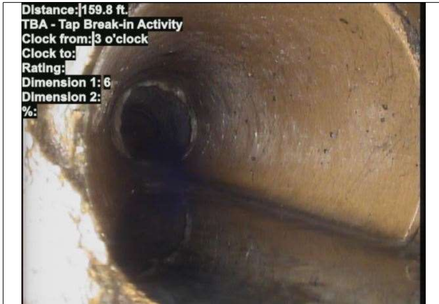
At: 159.8 ft. 3/. TBA - Tap Break-in Activity Joint: No
