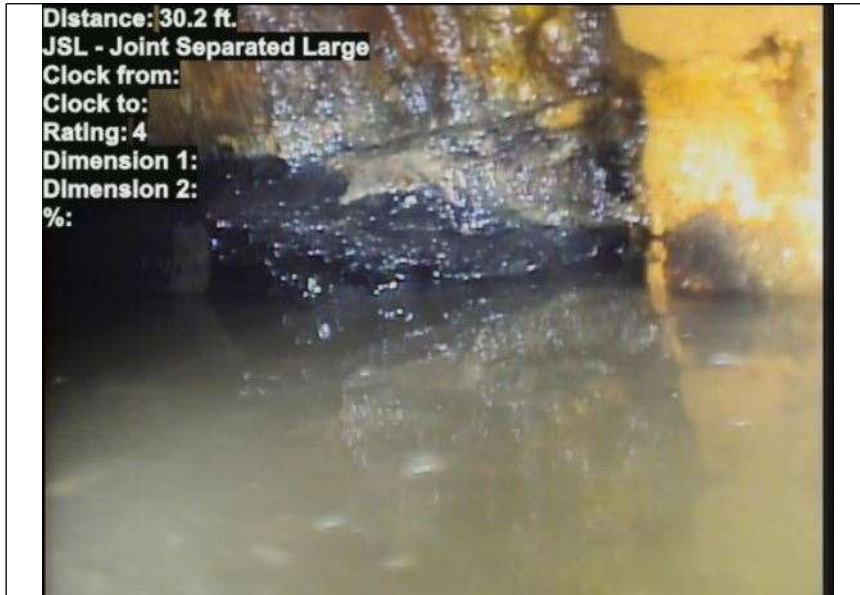
At: 30.2 ft. JSL - Joint Separated Large Joint: No
