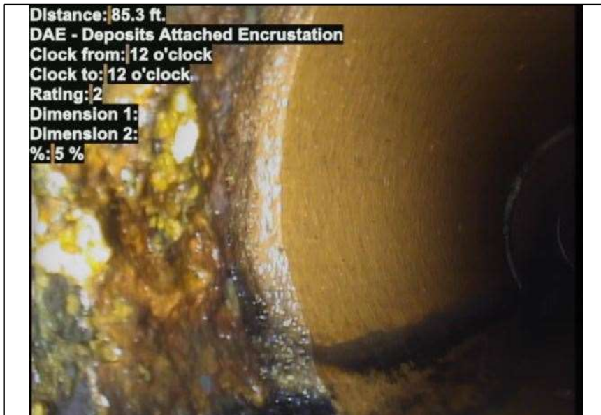
At: 85.3 ft. RPR - Point Repair Replacement Joint: No CAST IRON
