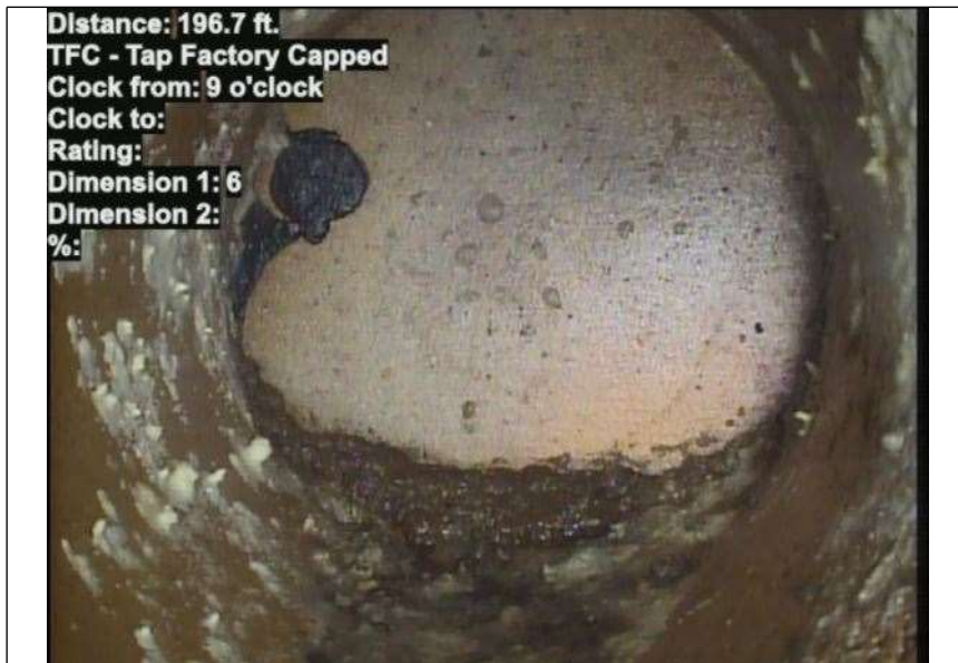
At: 196.7 ft. 9/. TFC - Tap Factory Capped Joint: No
