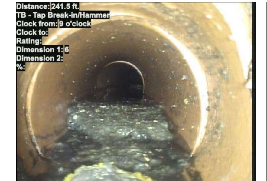
At: 241.5 ft. 9/. TB - Tap Break-in/Hammer Joint: No
