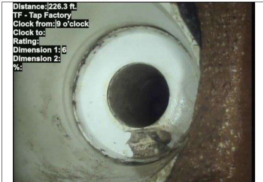
At: 226.3 ft. 9/. TF - Tap Factory Joint: No
