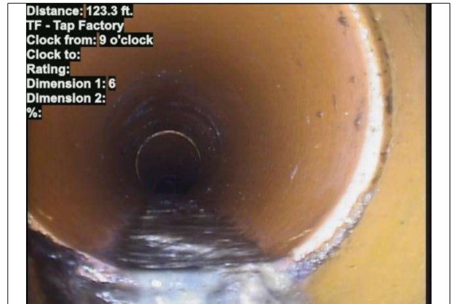
At: 123.3 ft. 9/ TF - Tap Factory Joint: No
