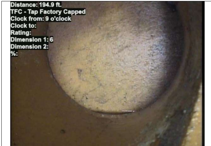
At: 194.9 ft. 9/. TFC - Tap Factory Capped Joint: No
