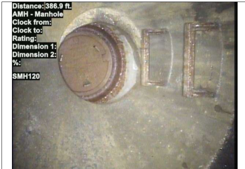
At: 386.9 ft. AMH - Manhole Joint: No SMH120
