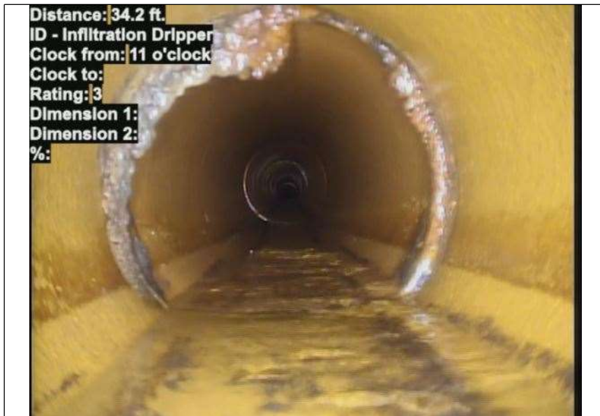
At: 34.2 ft. 11/. ID - Infiltration Dripper Joint: No
