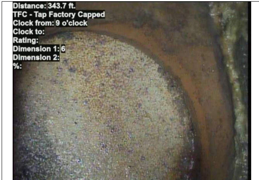
At: 343.7 ft. 9/. TFC - Tap Factory Capped Joint: No
