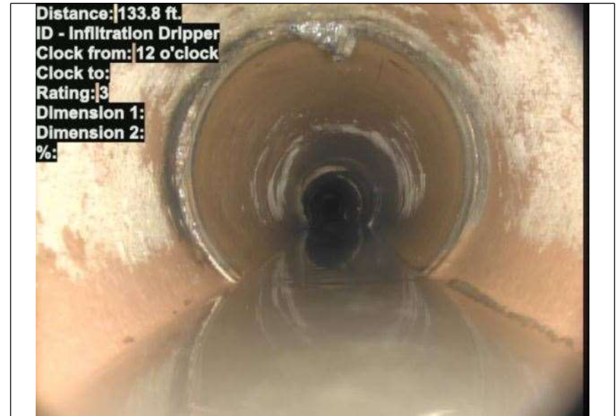
At: 133.8 ft. 12/ ID - Infiltration Dripper Joint: No
