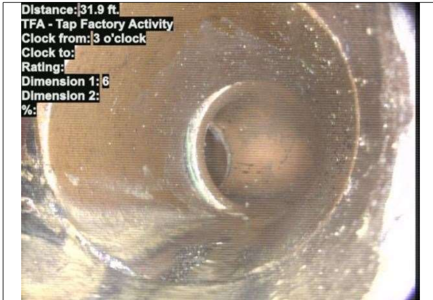
At: 31.9 ft. 3/. TFA - Tap Factory Activity Joint: No
