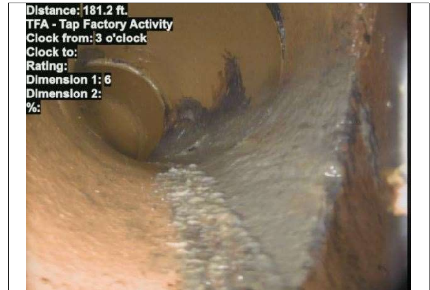
At: 181.2 ft. 3/. TFA - Tap Factory Activity Joint: No
