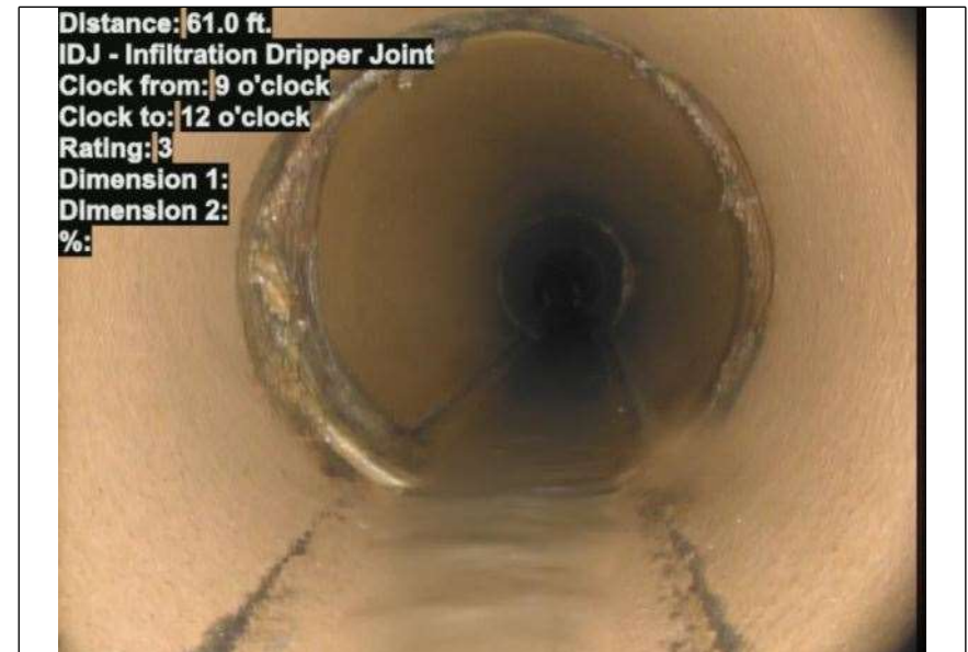
At: 61 ft. 9/12 IDJ - Infiltration Drifter Joint Joint: Yes
