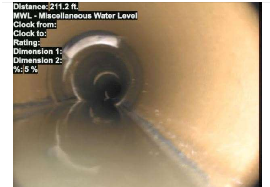
At: 211.2 ft. MWL - Miscellaneous Water Level Joint: No 5 %
