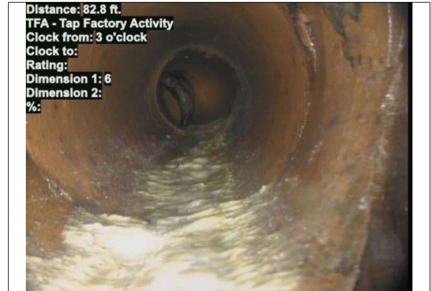
At: 82.8 ft. 3/ TFA - Tap Factory Activity Joint: No
