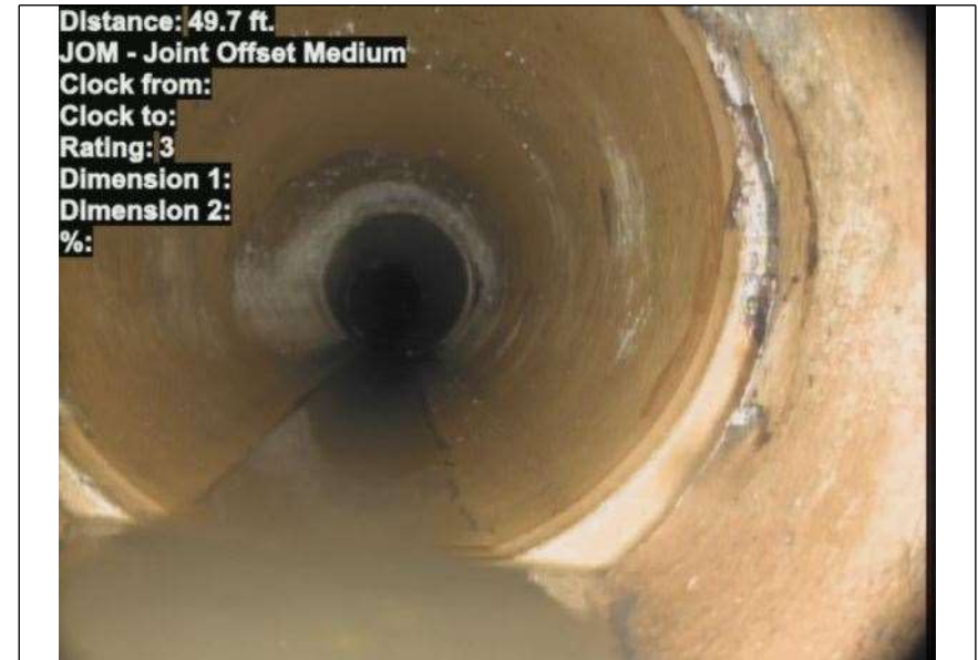
At: 49.7 ft. JOM - Joint Offset Medium Joint: No
