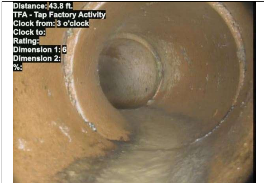
At: 43.8 ft. 3/ TFA - Tap Factory Activity Joint: No
