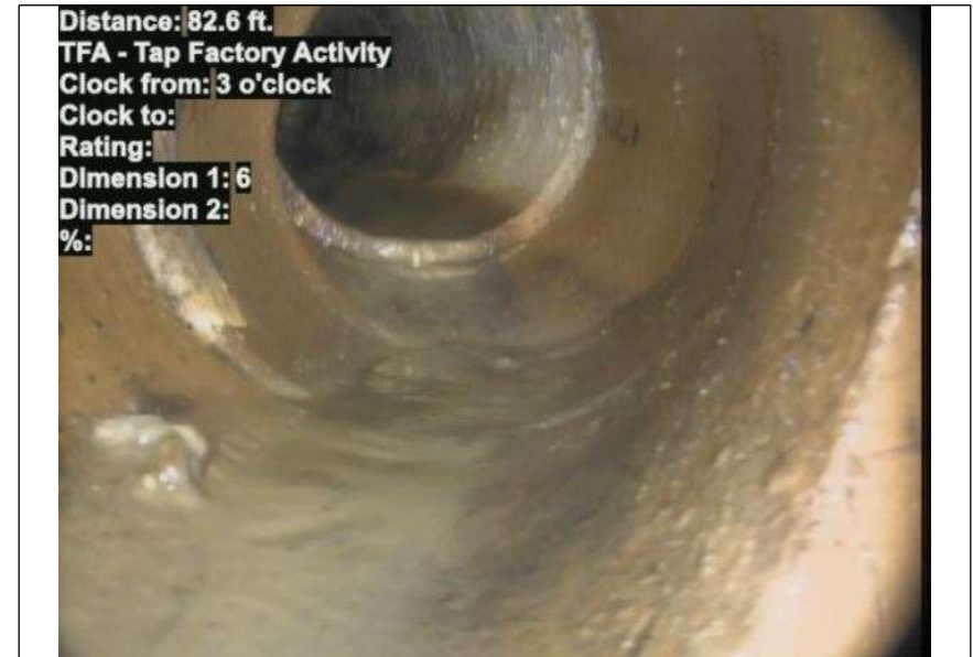
At: 82.6 ft. 3/ TFA - Tap Factory Activity Joint: No
