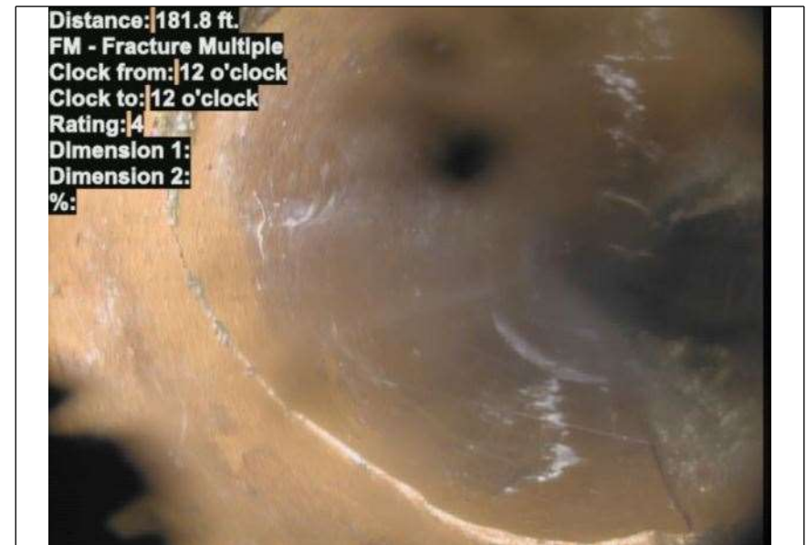
At: 181.8 ft. FM - Fracture Multiple 12/12
