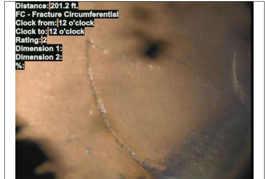
At: 201.2 ft. FC - Fracture Circumferential 12/12 Joint: No
