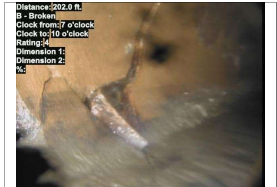
At: 202 ft. 7/10 B - Broken Joint: No
