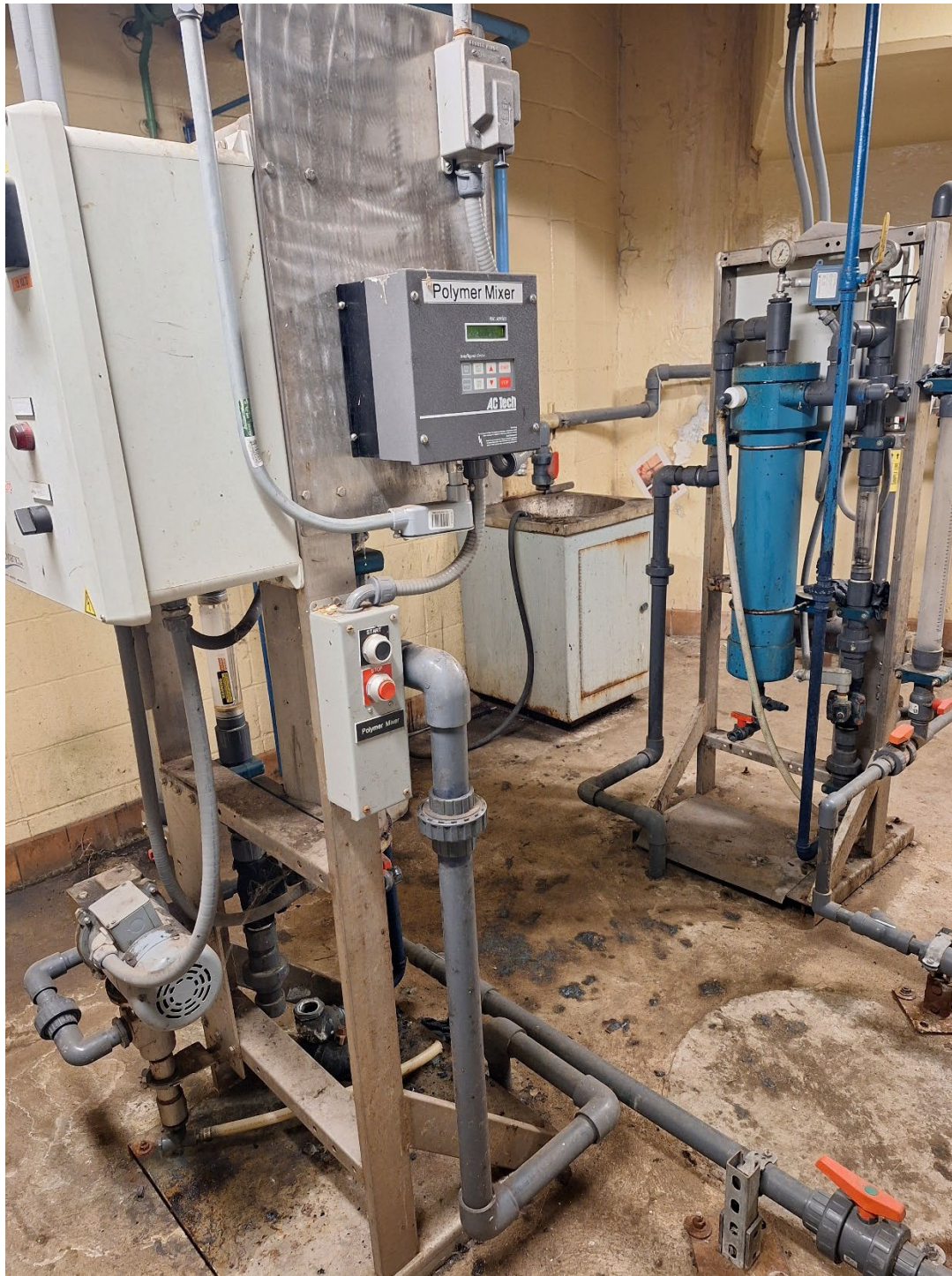
Existing Polymer Blend #1 on the left. Polymer Blend #2 on the right. Located on the 1st Floor, Polymer Room.
