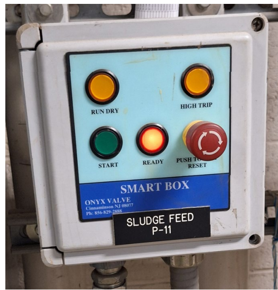
Existing Sludge Pumps P11 & P12 ONYX Valve Smart Box located next to the local control panels.
