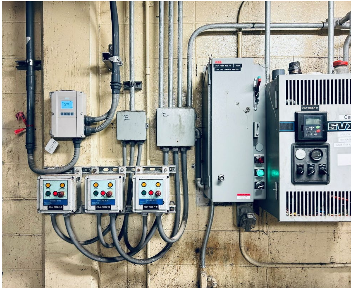
Existing Poly Feed Pumps P17, P18, P19 & Smart Boxes. Located on the 1st Floor Polymer Room
