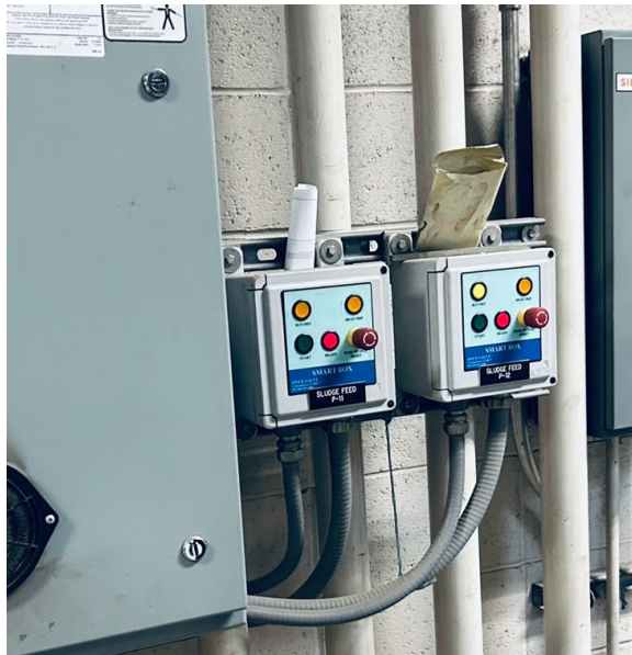
Existing Sludge Pumps P11 & P12 ONYX Valve Smart Box located next to the local control panels.
