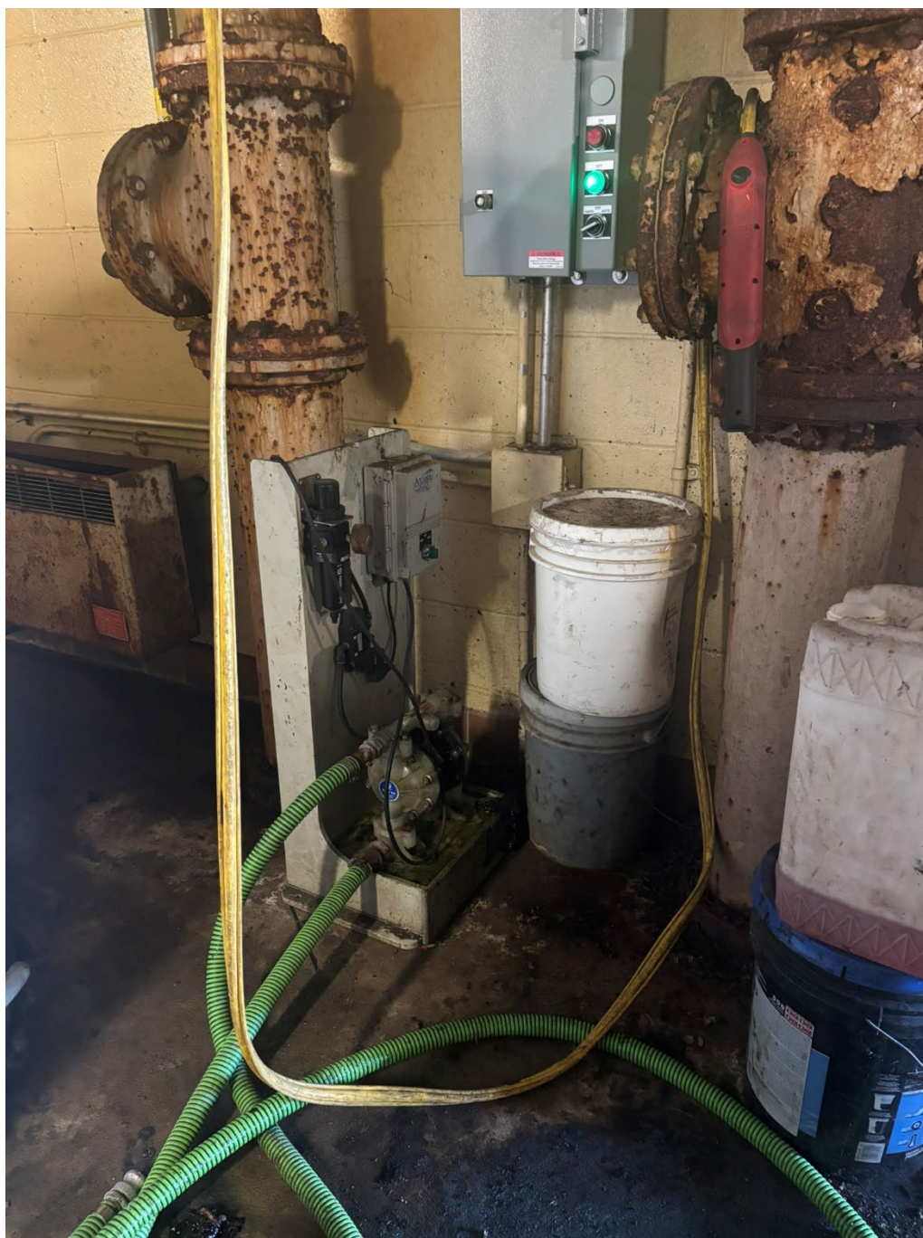
Existing Polymer Tote Transfer Pump. Located on the 1st Floor, Polymer Room
