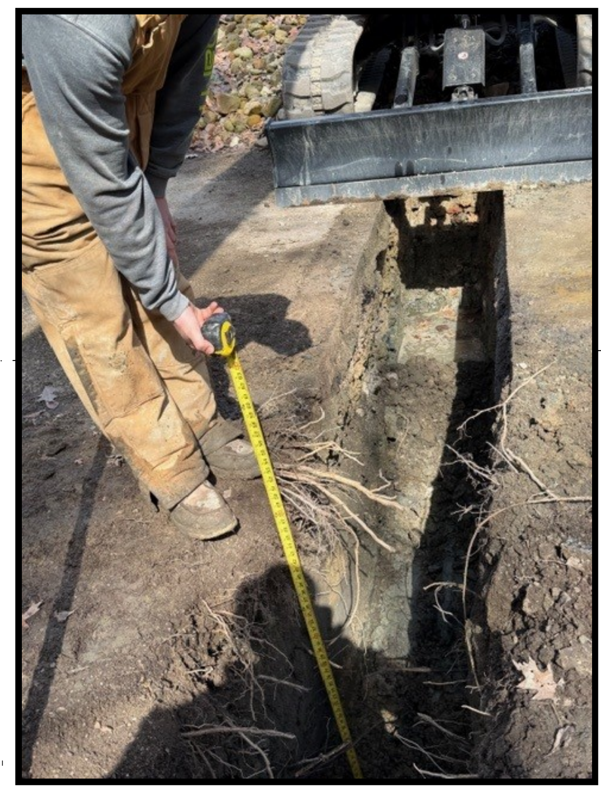
Aerial Crossing Utility Trench (4) Photo Not to Scale
