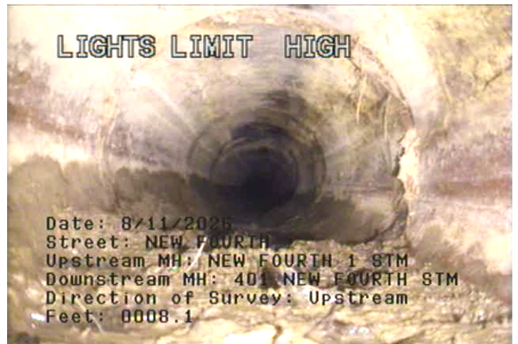
JOL - Joint Offset (displaced): Large @ 8.1 ft.
