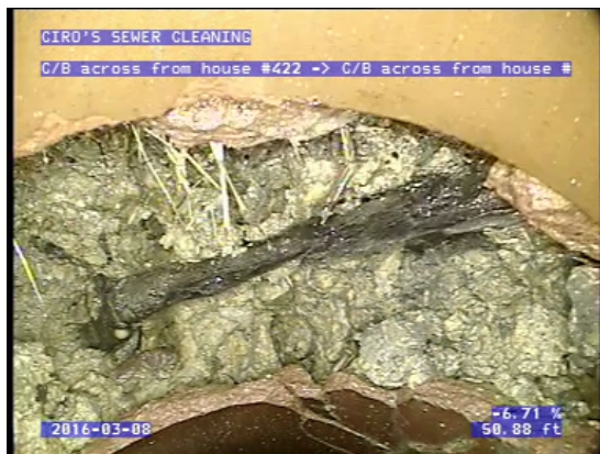
STS - New Fourth St. – Hole in Crown; Soil Visible
