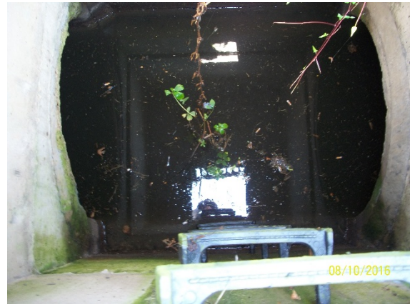
Storm Manhole ID 100098 Standing Water Invert
