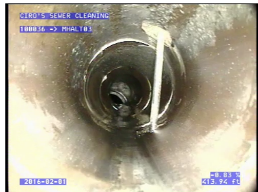
STS - Third St. – Utility Bored Through Storm Sewer
