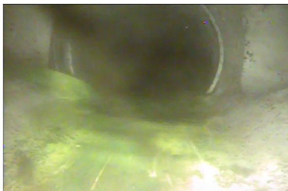
600 Third St. – 3:00 and 9:00 Tee Connection on Lateral With Dyed Water Entering (Camera in SAS Lateral Looking Towards Sanitary Main)
