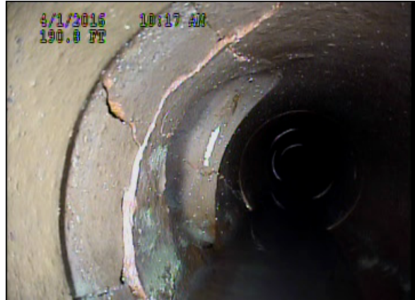
SAS - Chestnut St. – Multiple Fractures
