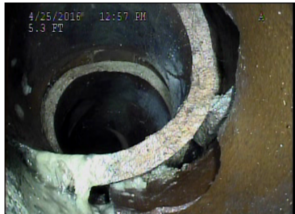
SAS - Second St. – Broken Tee Connection
