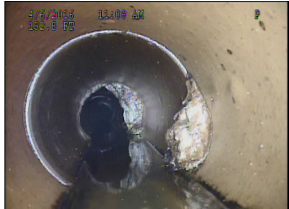
SAS - Joughin St. - Mineral Deposits at Joints
