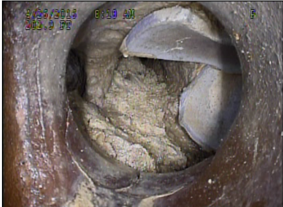
SAS - Second St. – Lateral with Heavy Debris
