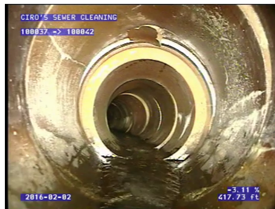
STS - Harding School – Repair with Smaller Pipe
