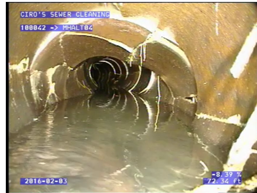
STS - Harding School- Fractured, Deformed Pipe
