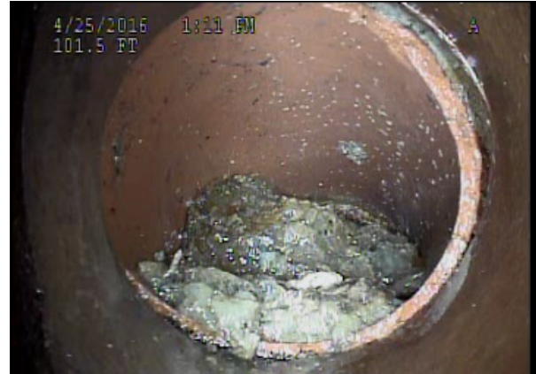
SAS - Second St. – Lateral with Heavy Debris
