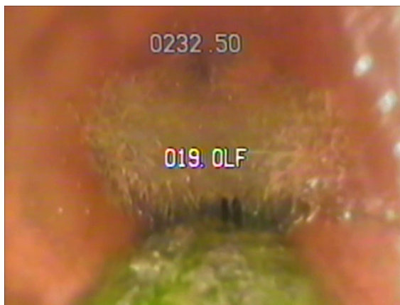
517 Fifth St. – Large Root Ball (Camera in SAS Lateral Looking Towards House)
