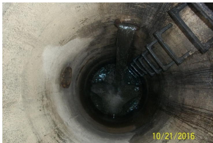
Sanitary Manhole at Third St. and Vine St. During Wet Weather Flow
