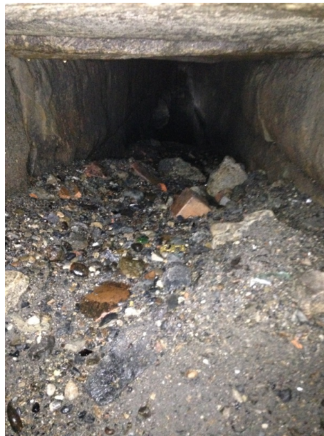
STS - High St. – Box Culvert Before Cleaning
