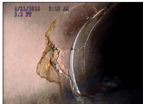
SAS - Fifth St. – Hole, Multiple Fractures
