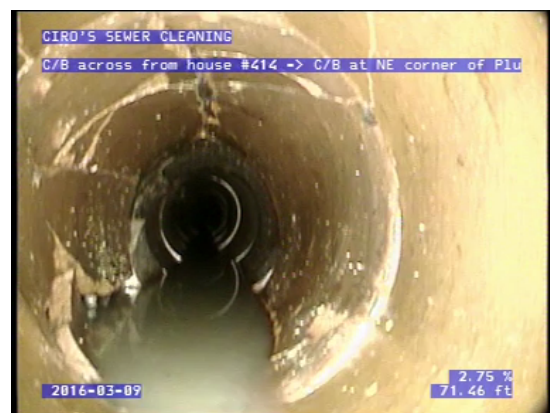
STS - New Fourth St. – Fractures/Broken Pipe
