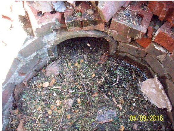
Catch Basin Located on York St. Loose Bricks and Full of Debris
