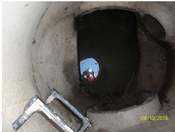
Storm Manhole Asset ID 100056 Standing Water in Invert
