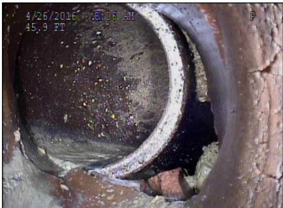
SAS - Second St. – Broken Tee Connection
