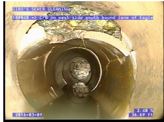
STS - New Fourth St. – Large Hole; Soil Visible
