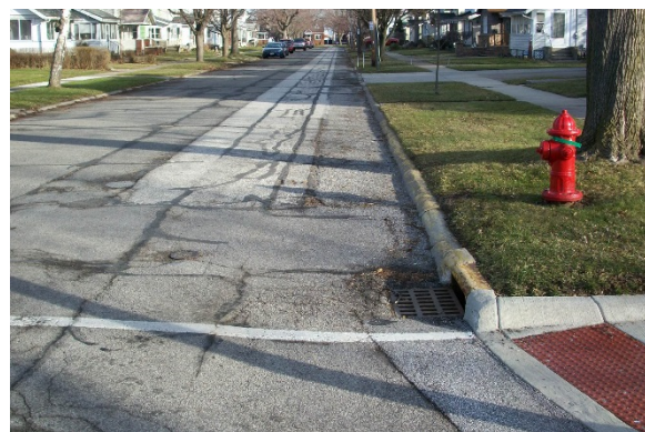
Chestnut St. Typical Curb and Catch Basin Collection System
