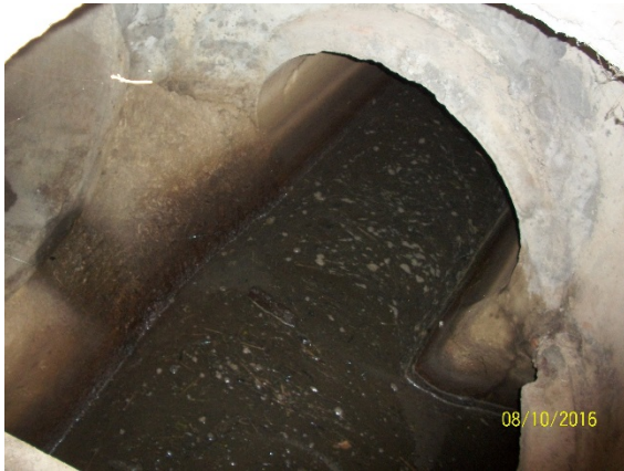
Storm Manhole ID 100128 Standing Water Invert
