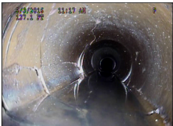
SAS - East St. – Multiple Fractures
