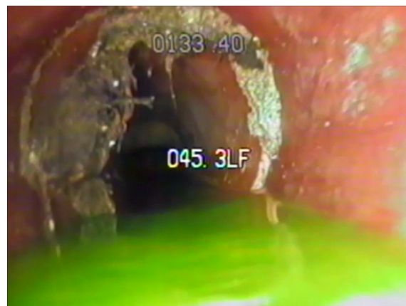
533 Third St. – Medium Root Ball (Camera in SAS Lateral Looking Towards House)
