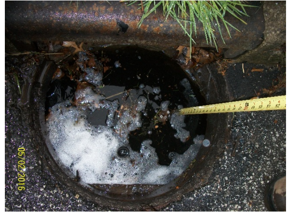
Catch Basin Located on Second St. Clogged With Debris, Water Backed Up
