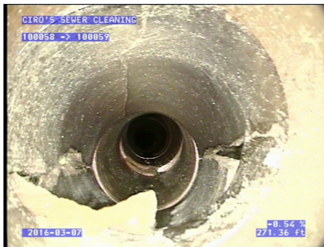
STS - East St. – Broken Pipe Looking Downstream
