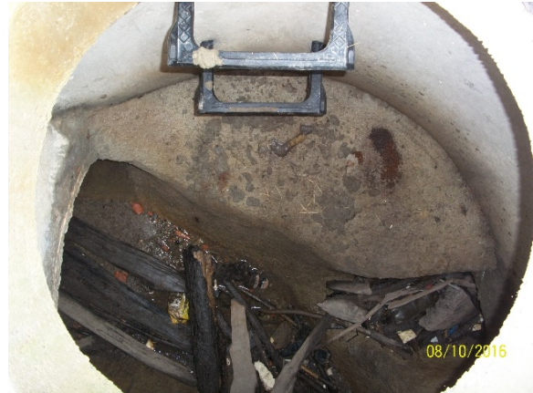
Storm Manhole Asset ID 100127 Large Amounts of Wood Debris
