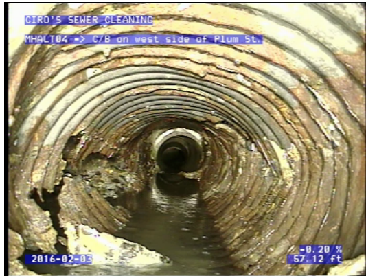
STS - Plum St. – CMP Deformed; Hole in Pipe
