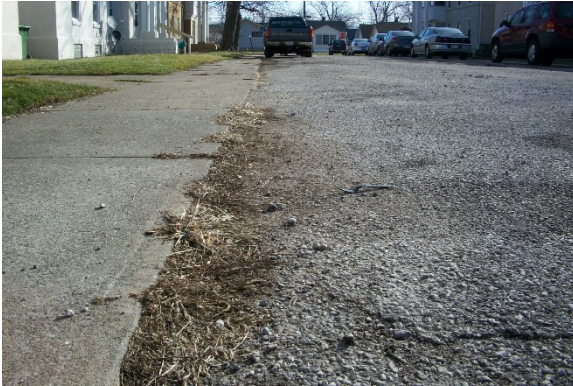
Paradise Ct. No Curb For Stormwater Conveyance
