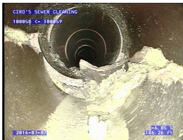
STS - East St. – Broken Pipe Looking Upstream
