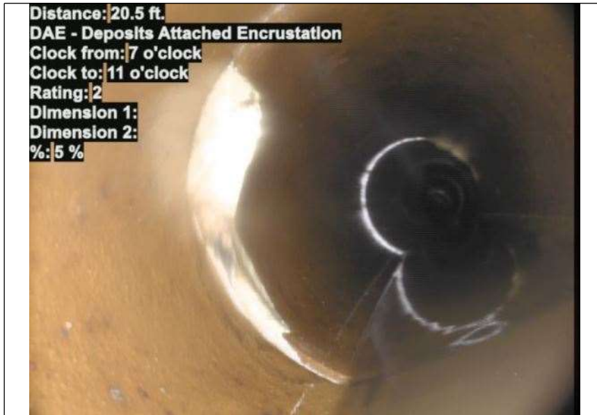
At: 20.5 ft. 7/11 DAE - Deposits Attached Encrustation Joint: No 5 %
