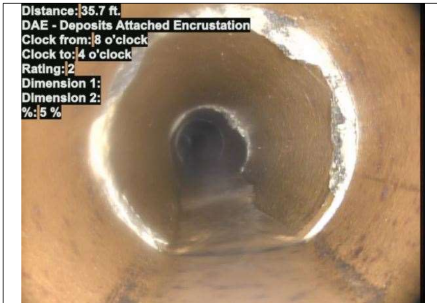
At: 35.7 ft. 8/4 DAE - Deposits Attached Encrustation Joint: No 5 %
