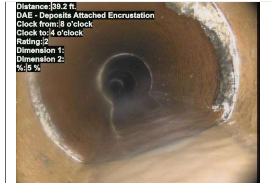
At: 39.2 ft. 8/4 DAE - Deposits Attached Encrustation Joint: No 5 %
