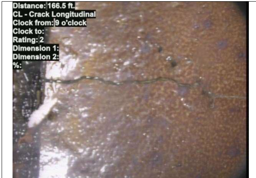
At: 166.5 ft. 9/. CL - Crack Longitudinal Joint: No
