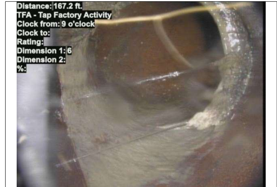
At: 167.2 ft. 9/. TFA - Tap Factory Activity Joint: No
