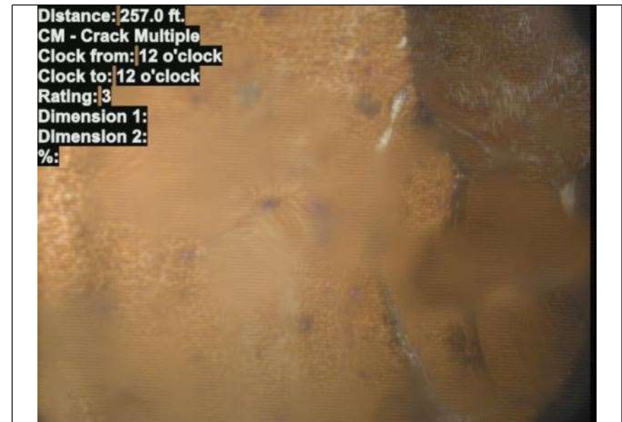
At: 257 ft. 12/12 CM - Crack Multiple
