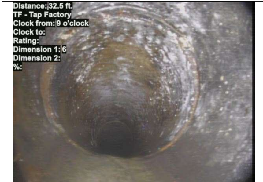
At: 32.5 ft. 9/ TF - Tap Factory Joint: No
