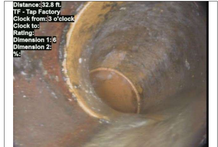
At: 32.8 ft. 3/ TF - Tap Factory Joint: No
