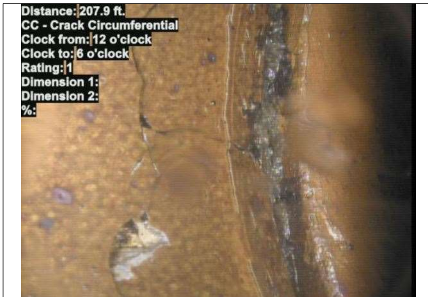
At: 207.9 ft. CC - Crack Circumferential 12/6
