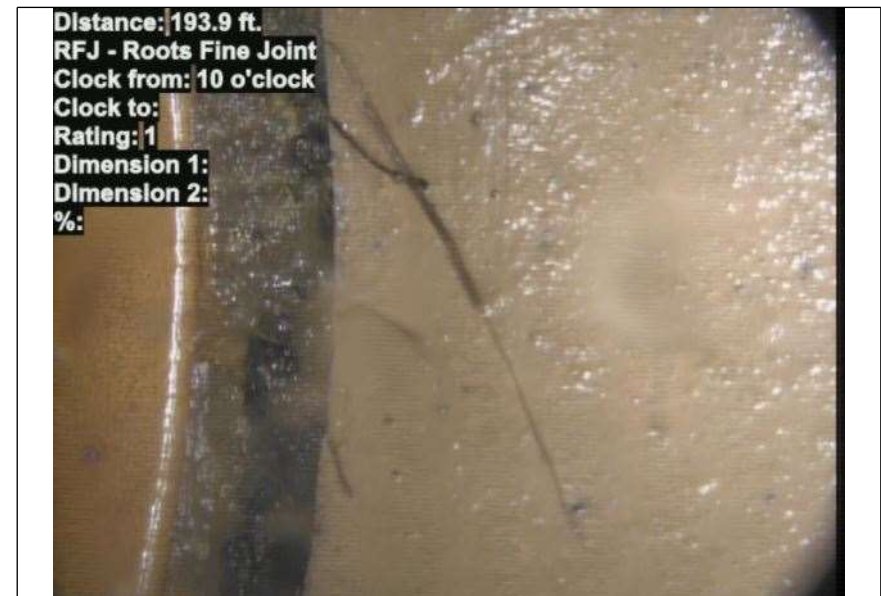
At: 193.9 ft. 10/. RFJ - Roots Fine Joint Joint: Yes
