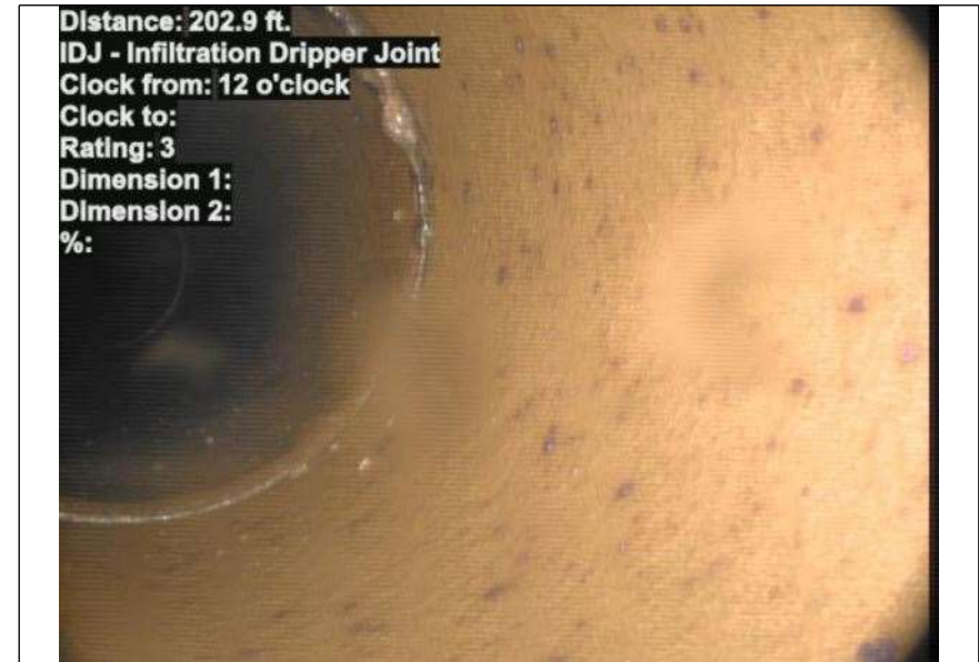
At: 202.9 ft. 12/ IDJ - Infiltration Dripper Joint
