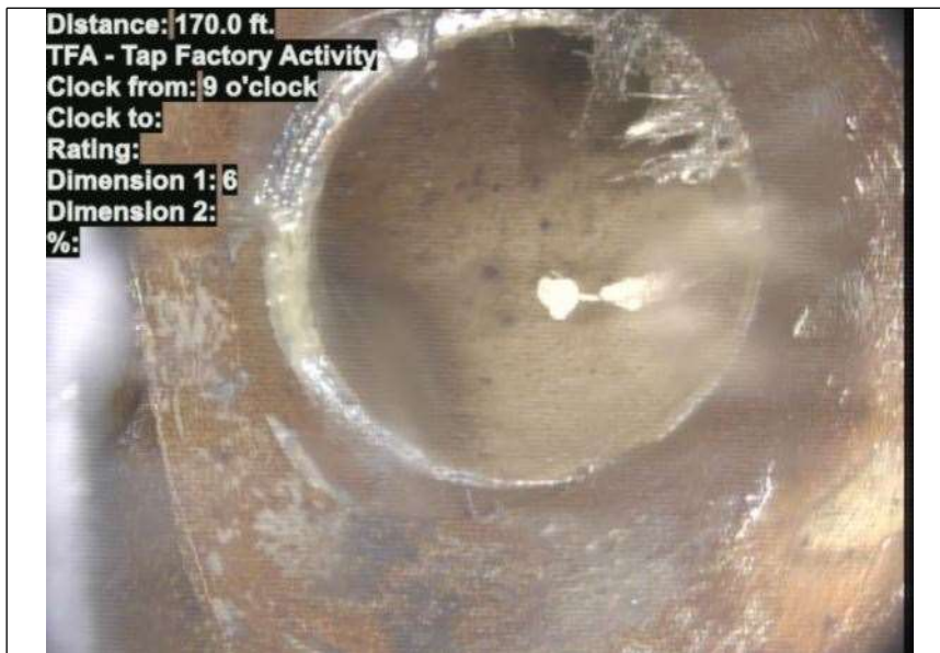
At: 170 ft. 9/. TFA - Tap Factory Activity Joint: No
