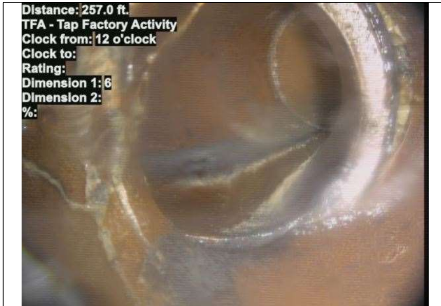
At: 257 ft. 12/. TFA - Tap Factory Activity Joint: No
