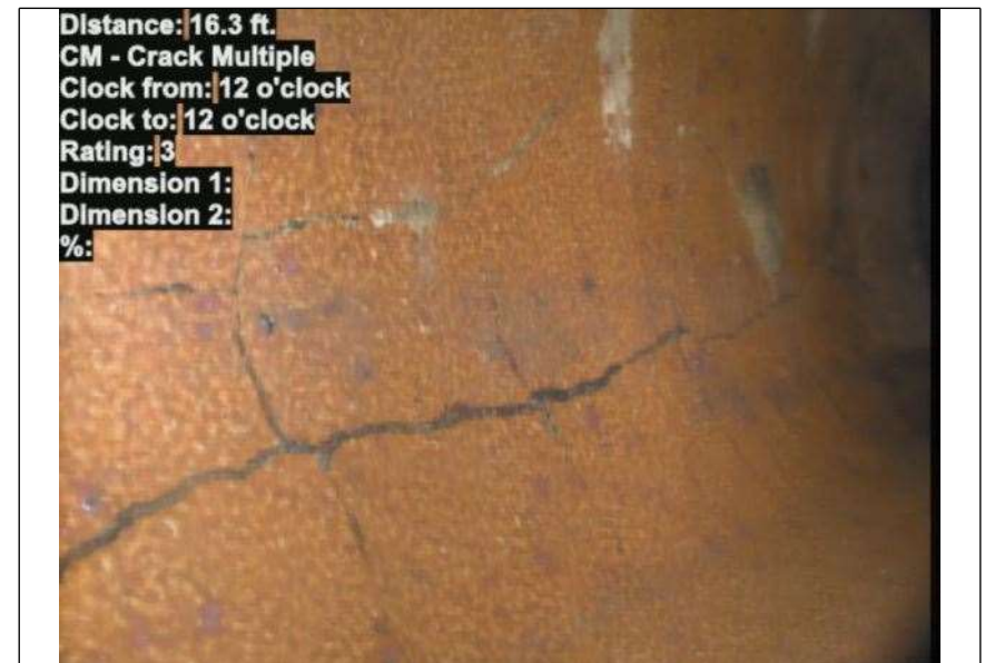
At: 16.3 ft. CM - Crack Multiple 12/12 Joint: No
