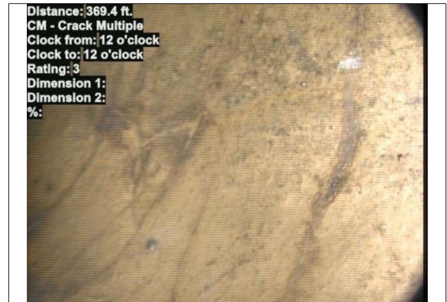
At: 369.4 ft. CM - Crack Multiple
