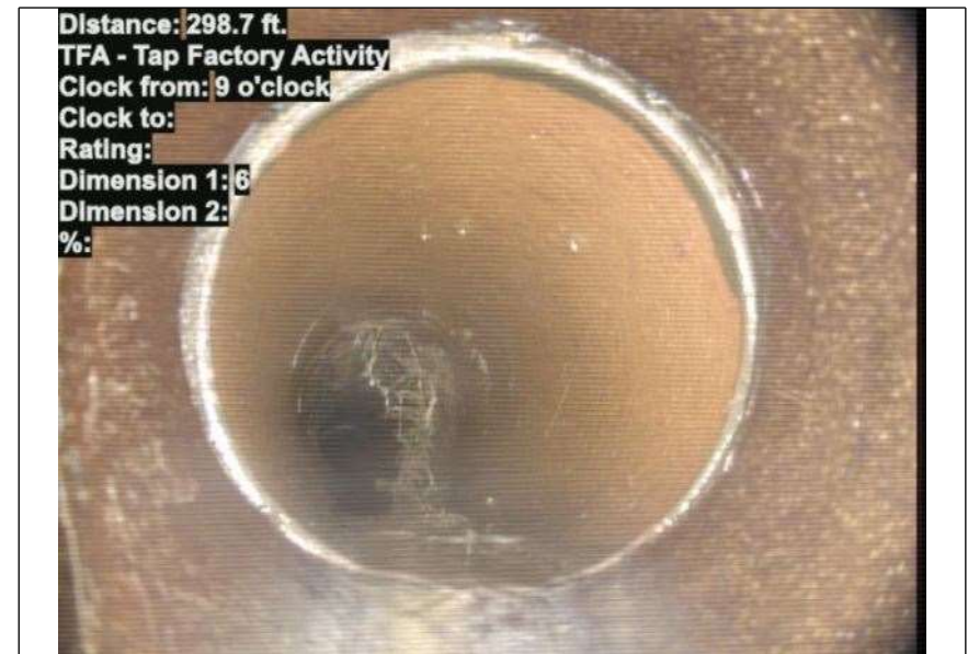
At: 298.7 ft. 9/. TFA - Tap Factory Activity Joint: No
