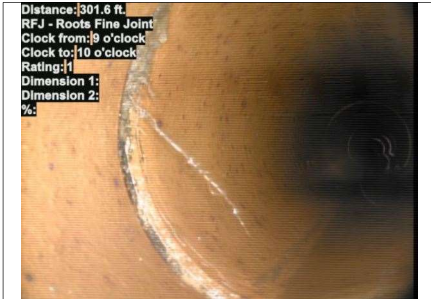
At: 301.6 ft. RFJ - Roots Fine Joint 9/10
