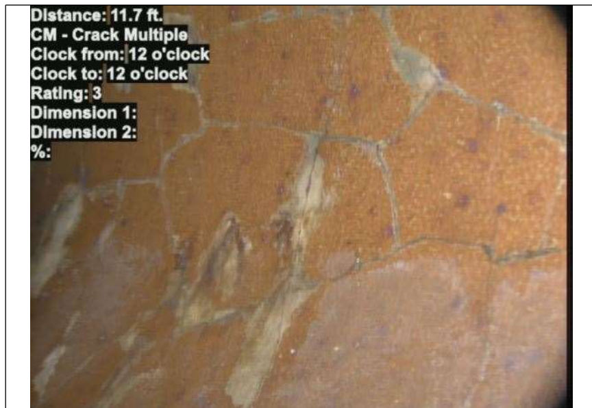
At: 11.7 ft. CM - Crack Multiple 12/12 Joint: No
