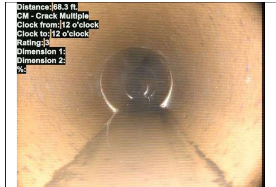
At: 68.3 ft. CM - Crack Multiple
