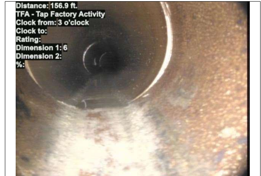
At: 156.9 ft. 3/. TFA - Tap Factory Activity Joint: No
