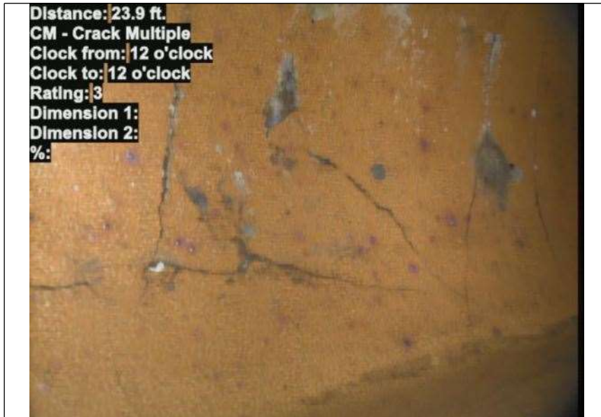
At: 23.9 ft. CM - Crack Multiple 12/12
