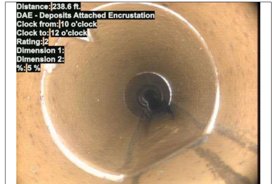
At: 238.6 ft. 10/12 DAE - Deposits Attached Encrustation Joint: No 5 %
