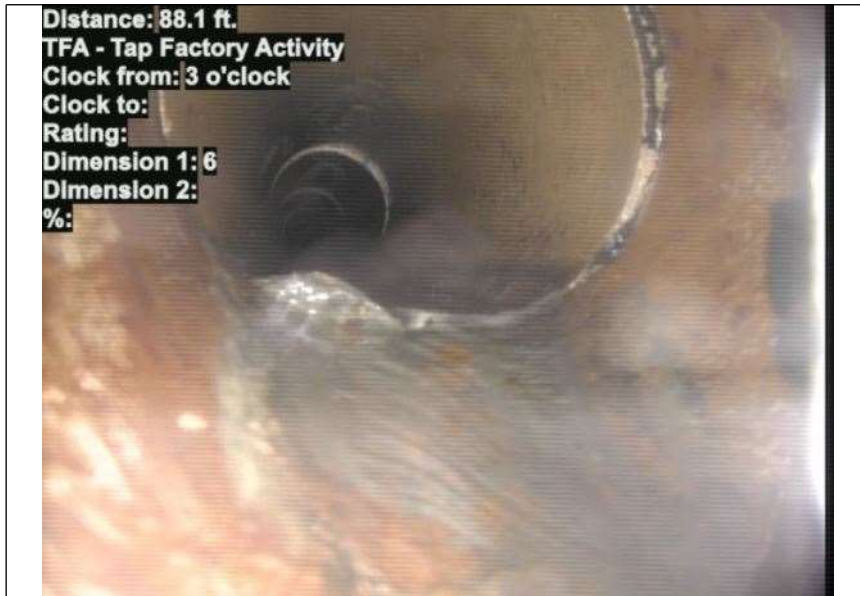
At: 88.1 ft. 3/. TFA - Tap Factory Activity Joint: No
