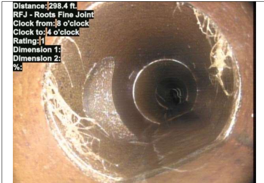
At: 298.4 ft. 8/4 RFJ - Roots Fine Joint Joint: Yes
