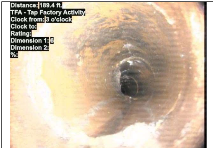
At: 189.4 ft. 3/. TFA - Tap Factory Activity Joint: No
