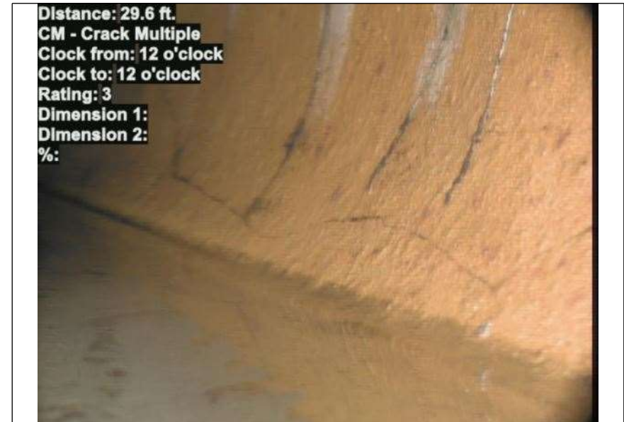
At: 29.6 ft. CM - Crack Multiple 12/12
