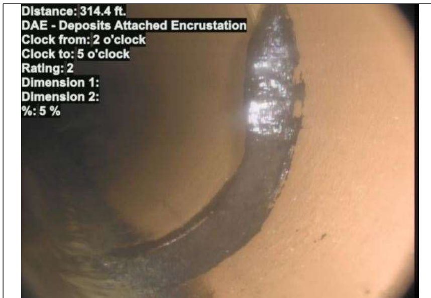
At: 314.4 ft. 2/5 DAE - Deposits Attached Encrustation Joint: No 5 %
