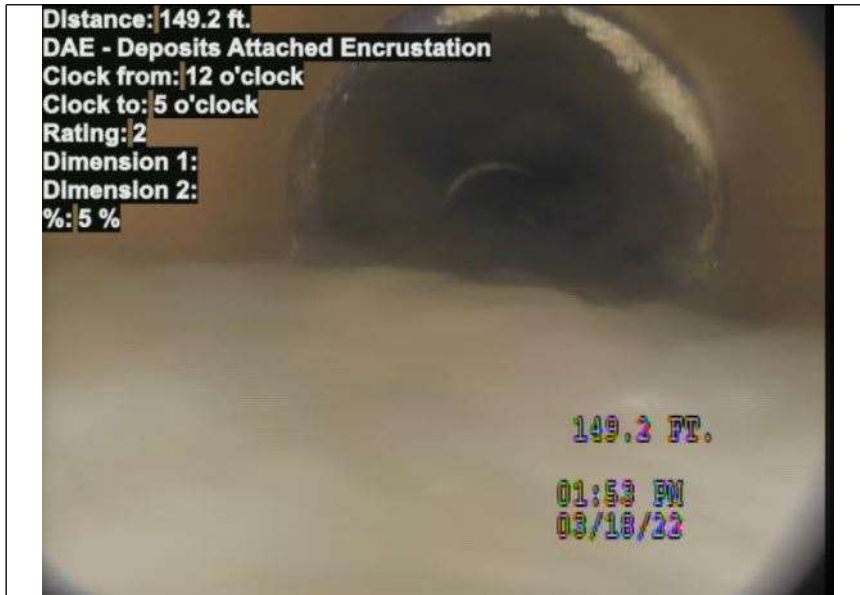
At: 149.2 ft. DAE - Deposits Attached Encrustation 12/5
