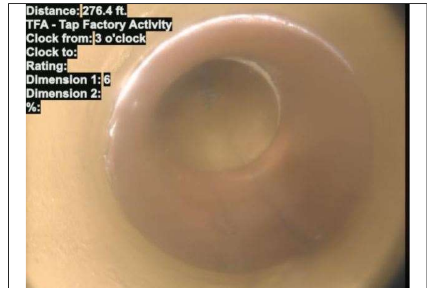
At: 276.4 ft. 3/. TFA - Tap Factory Activity Joint: No
