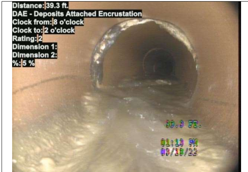
At: 39.3 ft. 8/2 DAE - Deposits Attached Encrustation Joint: No 5 %
