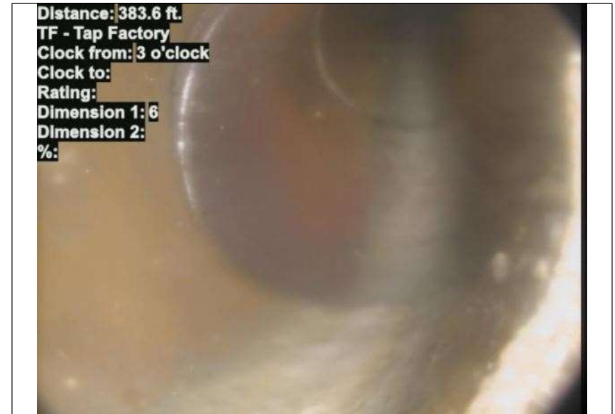
At: 383.6 ft. 3/. TF - Tap Factory Joint: No
