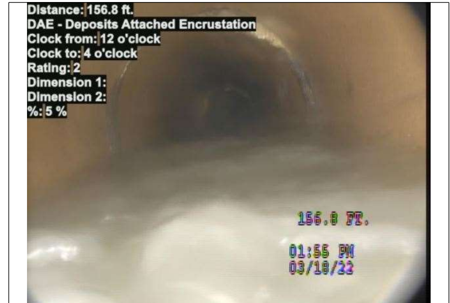
At: 156.8 ft. DAE - Deposits Attached Encrustation 12/4
