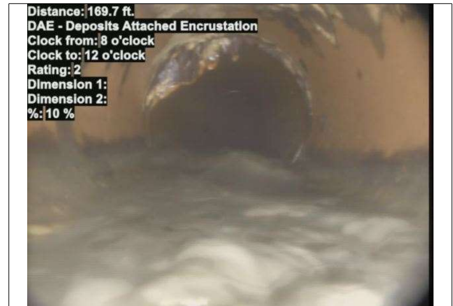
At: 169.7 ft. DAE - Deposits Attached Encrustation 8/12
