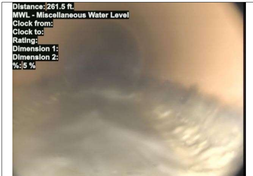
At: 261.5 ft. MWL - Miscellaneous Water Level Joint: No 5 %
