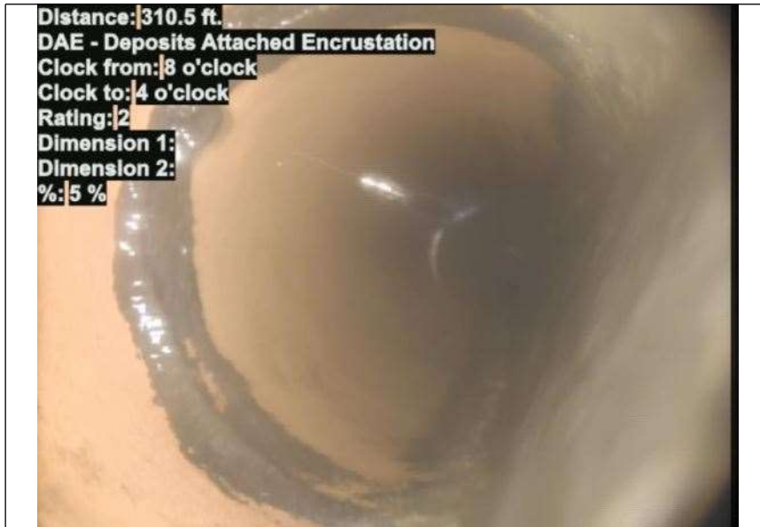
At: 310.5 ft. 8/4 DAE - Deposits Attached Encrustation Joint: No 5 %
