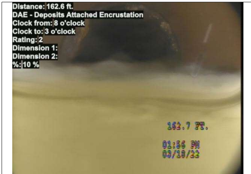
At: 162.6 ft. 8/3 DAE - Deposits Attached Encrustation
