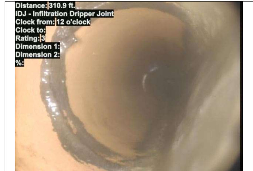
At: 310.9 ft. 12/. IDJ - Infiltration Dripper Joint Joint: Yes
