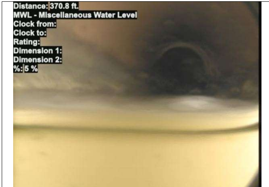
At: 370.8 ft. MWL - Miscellaneous Water Level Joint: No 5 %
