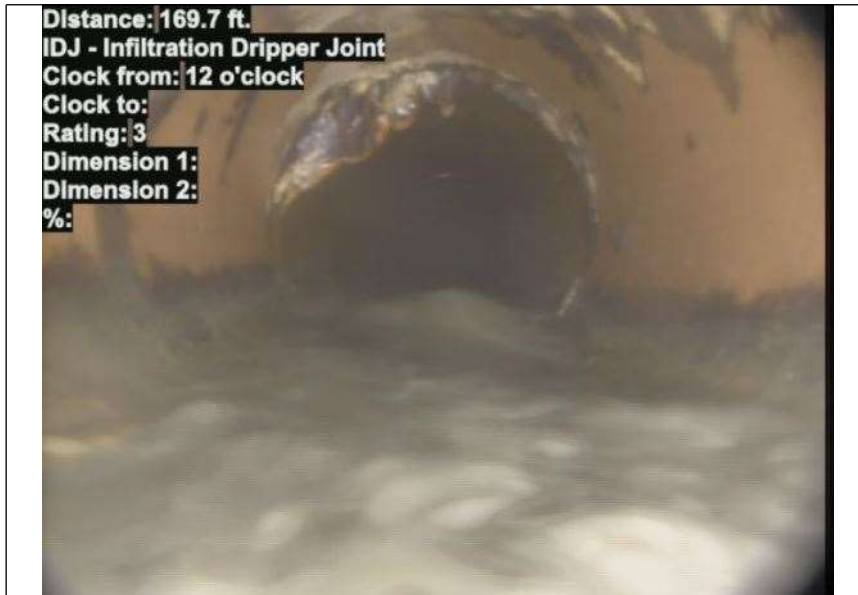
At: 169.7 ft. 12/. IDJ - Infiltration Dripper Joint Joint: Yes
