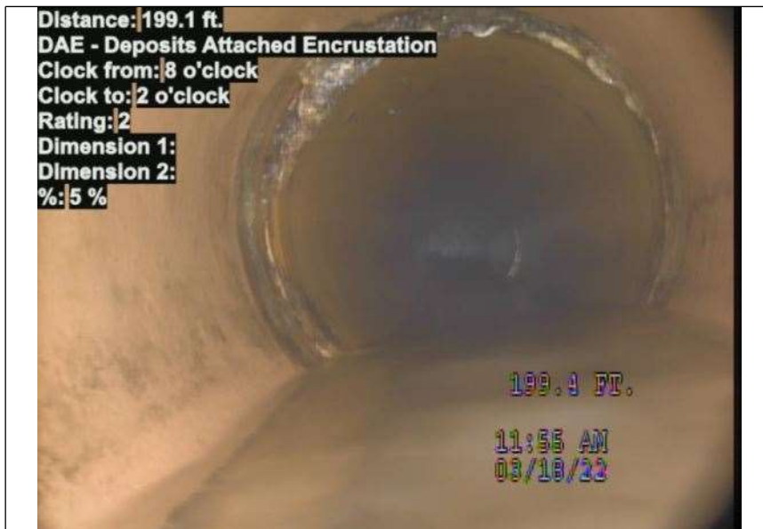
At: 199.1 ft. 8/2 DAE - Deposits Attached Encrustation Joint: No 5 %
