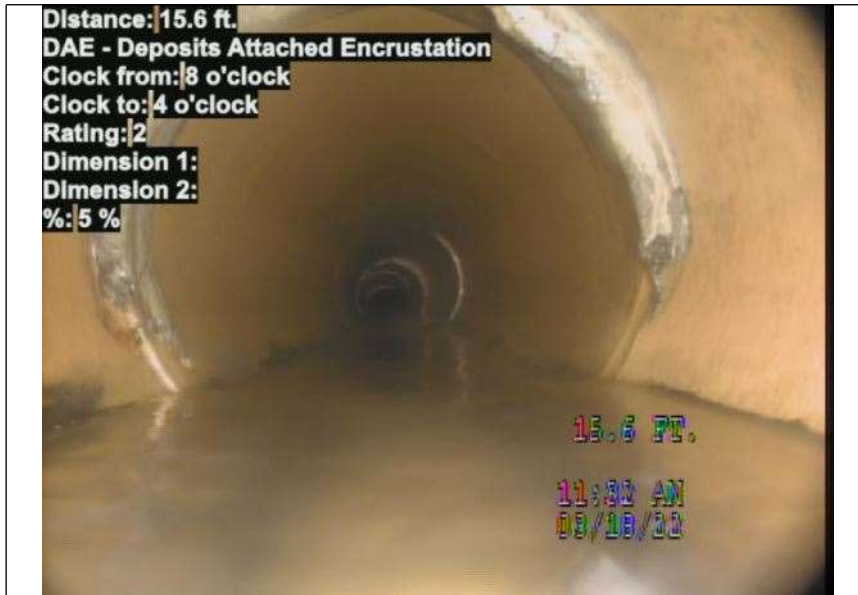
At: 15.6 ft. 8/4 DAE - Deposits Attached Encrustation Joint: No 5 %
