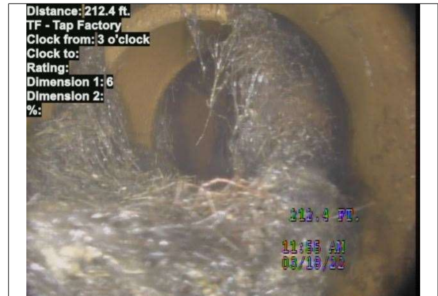
At: 212.4 ft. 3/. TF - Tap Factory Joint: No RFL
