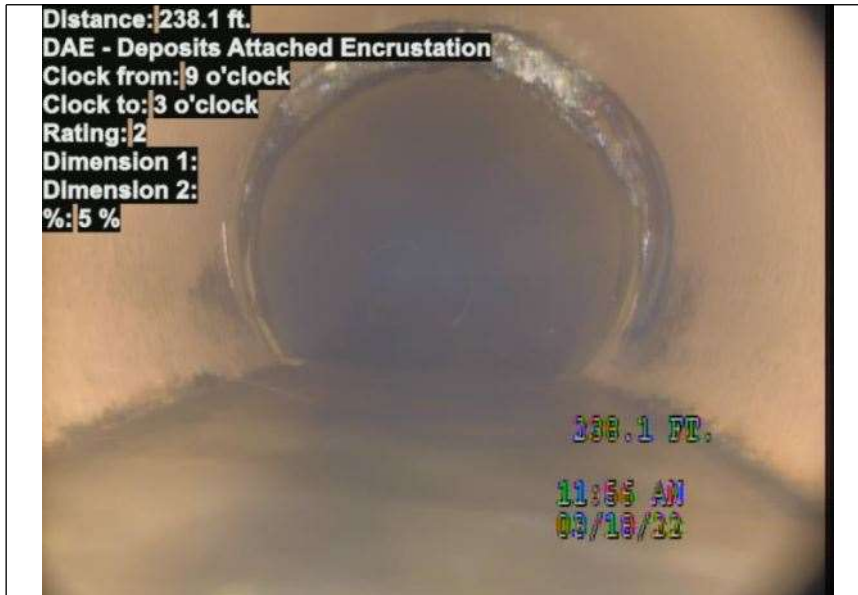
At: 238.1 ft. 9/3 DAE - Deposits Attached Encrustation Joint: No 5 %
