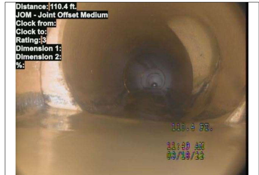
At: 110.4 ft. JOM - Joint Offset Medium Joint: No
