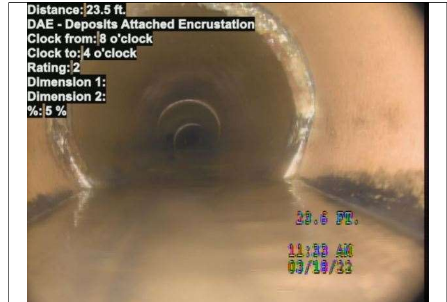
At: 23.5 ft. 8/4 DAE - Deposits Attached Encrustation Joint: No 5 %
