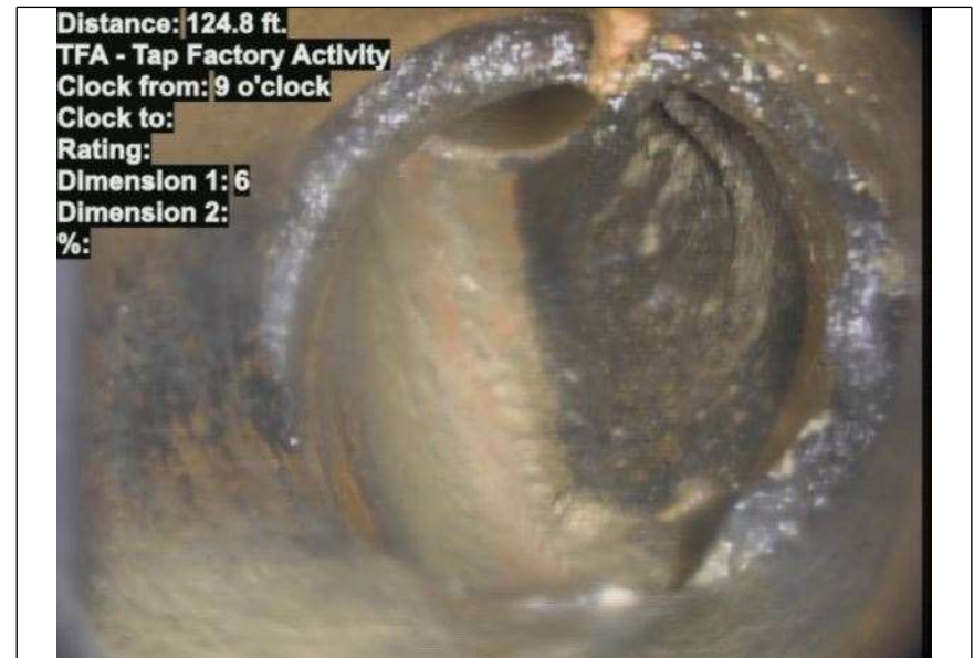
At: 124.8 ft. 9/ TFA - Tap Factory Activity Joint: No
