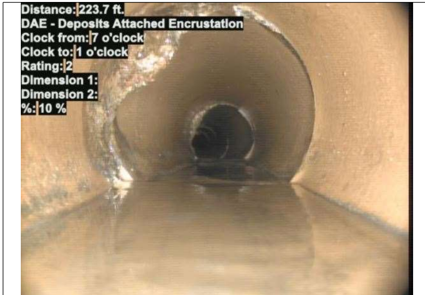
At: 223.7 ft. 7/1 DAE - Deposits Attached Encrustation Joint: No 10 %
