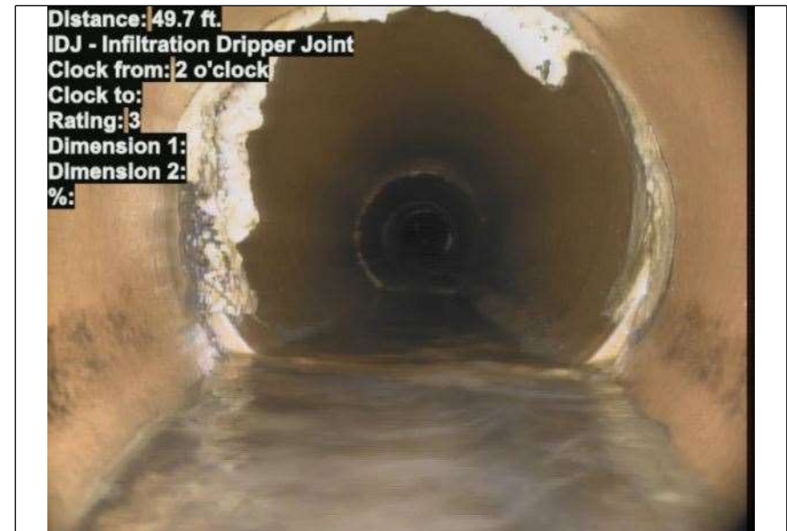
At: 49.7 ft. 2/ IDJ - Infiltration Dripper Joint Joint: Yes
