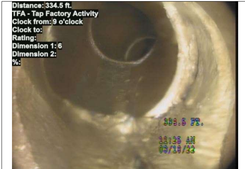
At: 334.5 ft. 9/. TFA - Tap Factory Activity Joint: No
