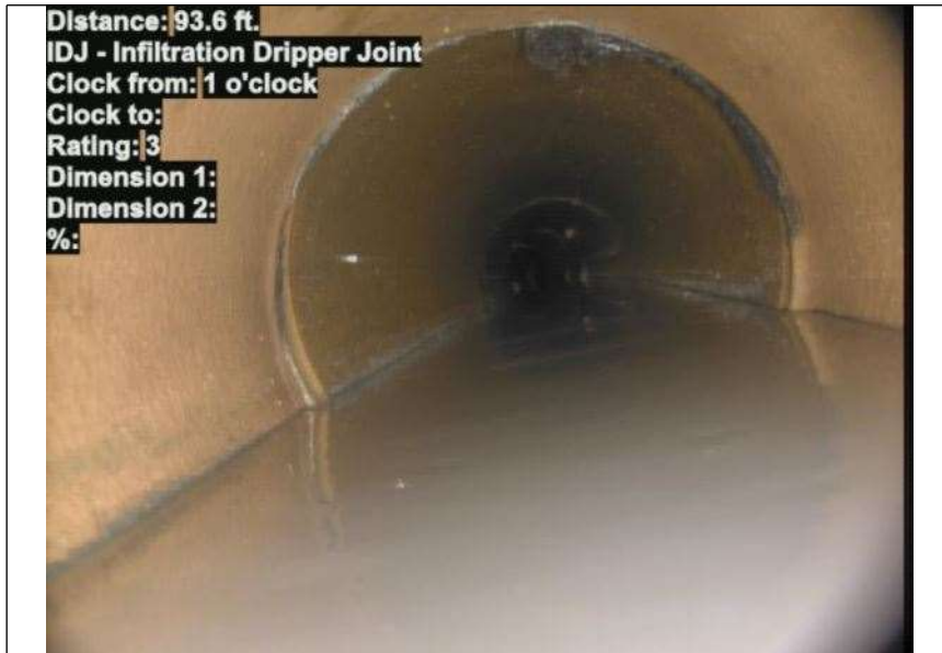
At: 93.6 ft. 1/ IDJ - Infiltration Dripper Joint Joint: Yes
