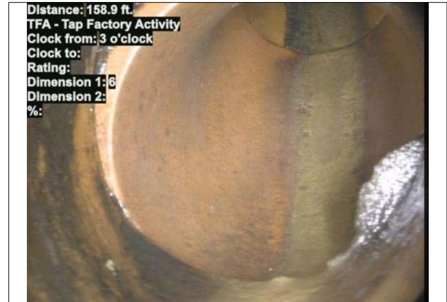
At: 158.9 ft. 3/. TFA - Tap Factory Activity Joint: No
