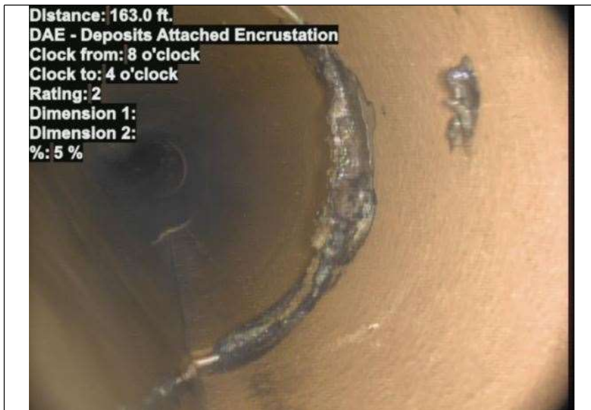
At: 163 ft. 8/4 DAE - Deposits Attached Encrustation Joint: No 5 %
