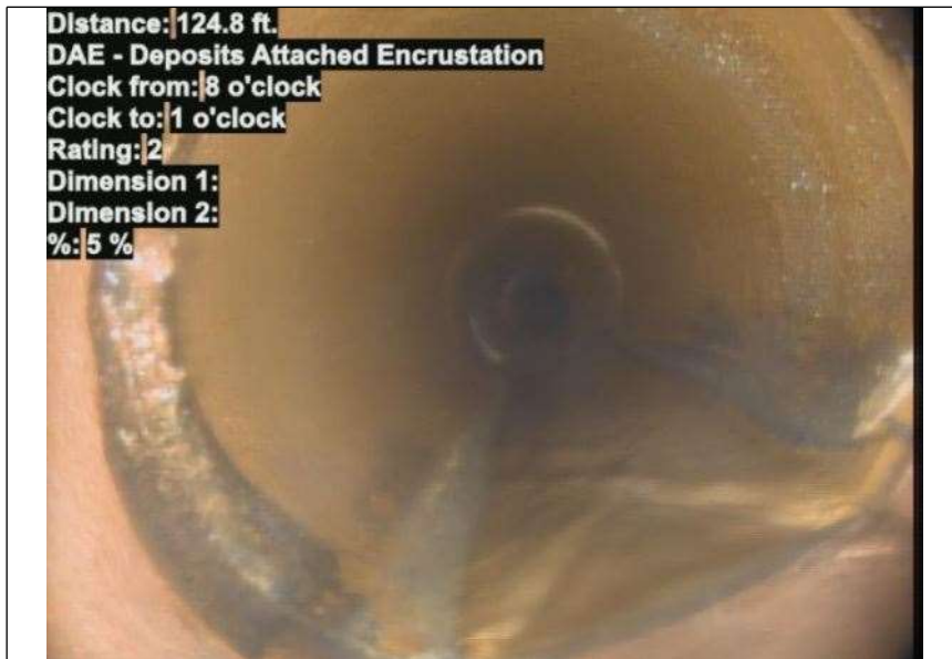
At: 124.8 ft. 8/1 DAE - Deposits Attached Encrustation Joint: No 5 %
