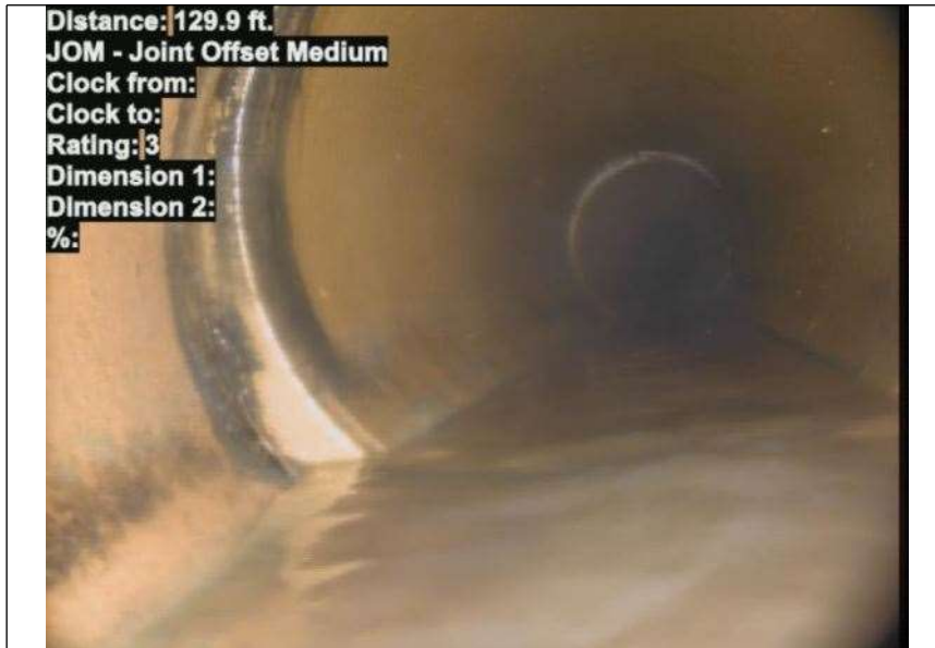
At: 129.9 ft. JOM - Joint Offset Medium Joint: No
