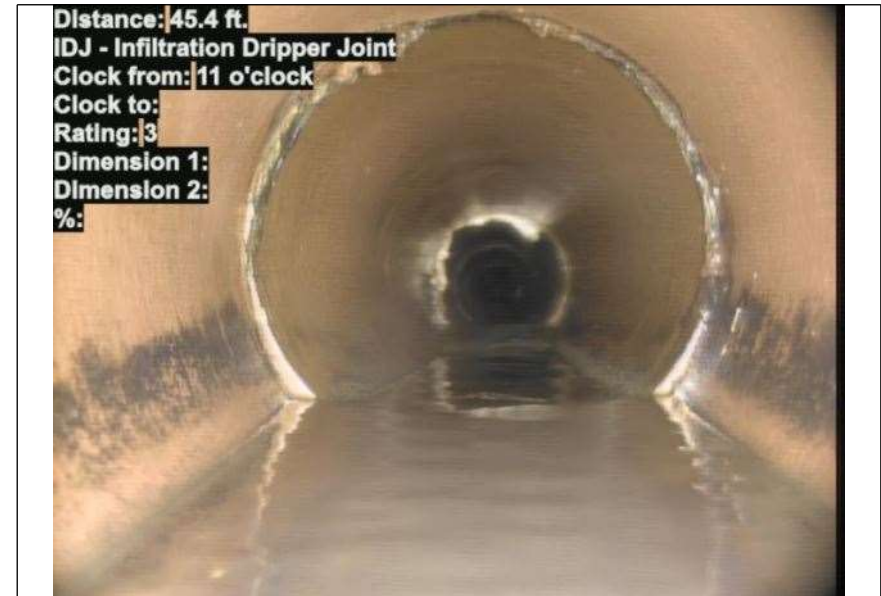
At: 45.4 ft. 11/ IDJ - Infiltration Dripper Joint Joint: Yes
