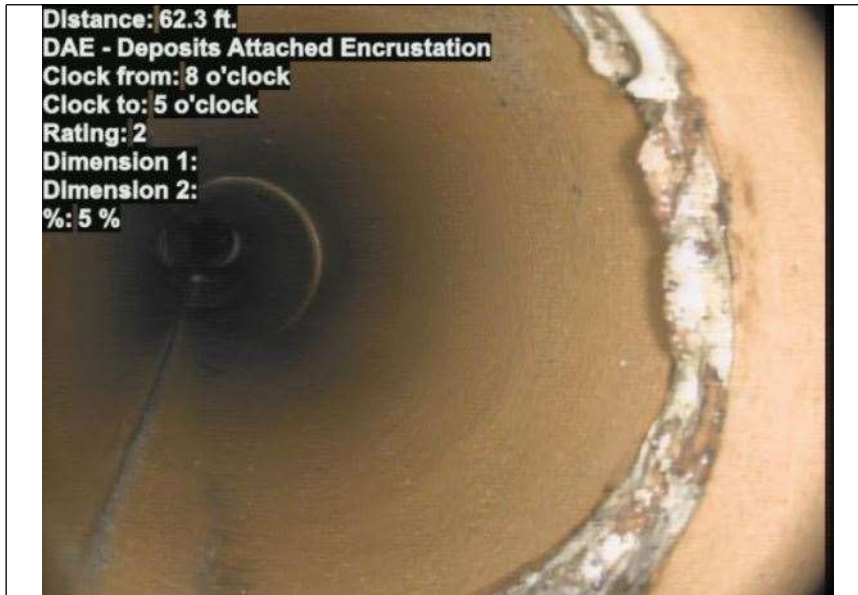
At: 62.3 ft. 8/5 DAE - Deposits Attached Encrustation Joint: No 5 %
