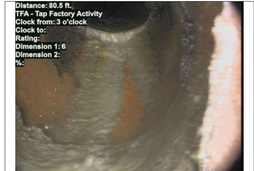
At: 80.5 ft. 3/ TFA - Tap Factory Activity Joint: No
