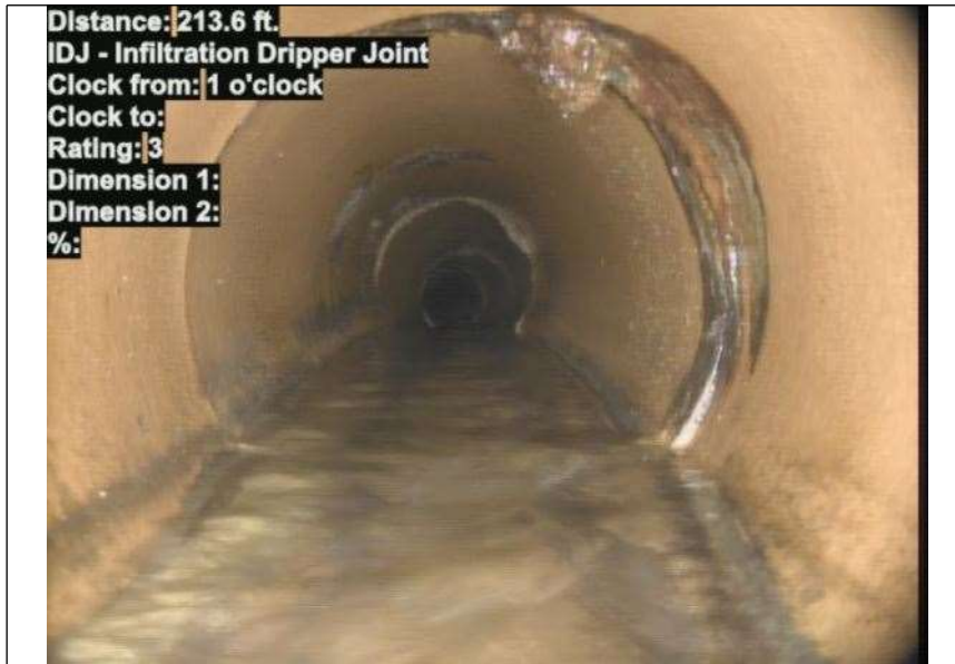
At: 213.6 ft. 1/. IDJ - Infiltration Dripper Joint Joint: Yes
