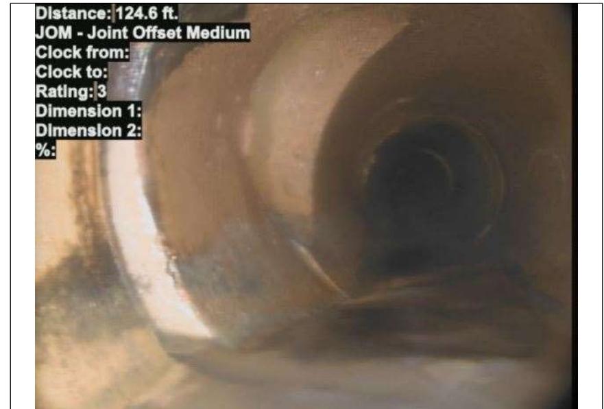
At: 124.6 ft. JOM - Joint Offset Medium Joint: No
