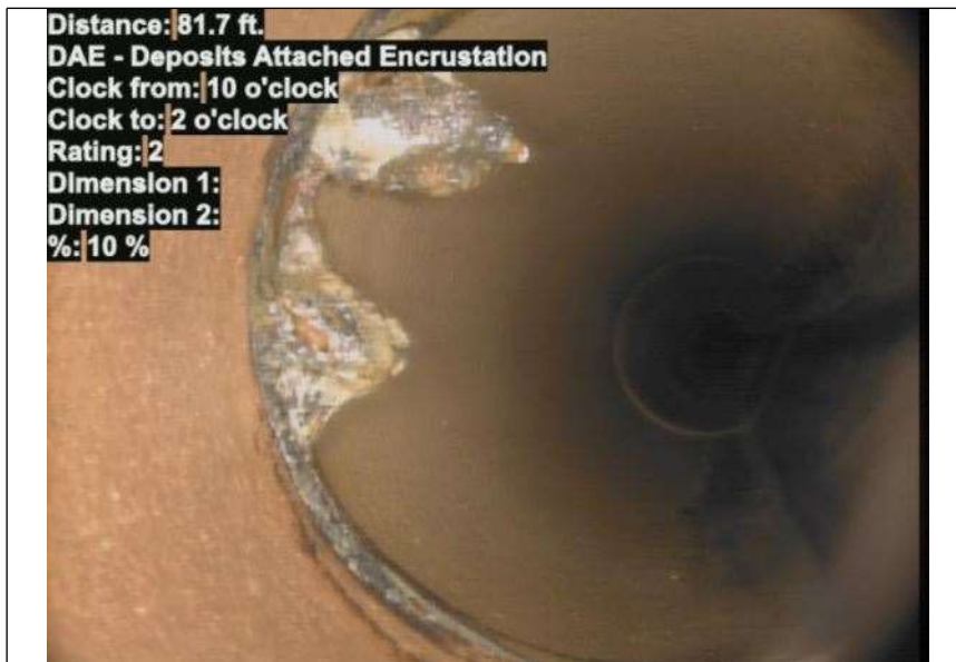
At: 81.7 ft. 10/2 DAE - Deposits Attached Encrustation Joint: No 10 %
