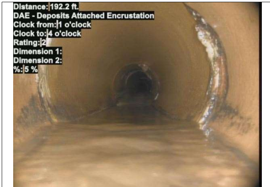
At: 192.2 ft. 1/4 DAE - Deposits Attached Encrustation Joint: No 5 %
