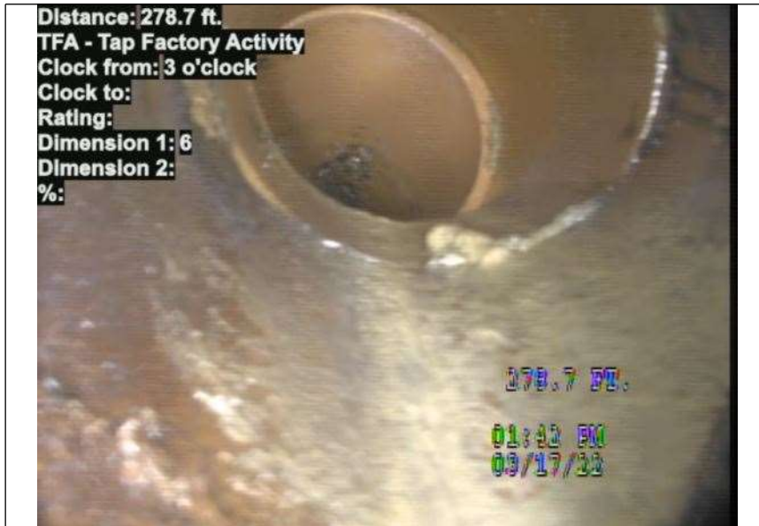
At: 278.7 ft. 3/. TFA - Tap Factory Activity Joint: No
