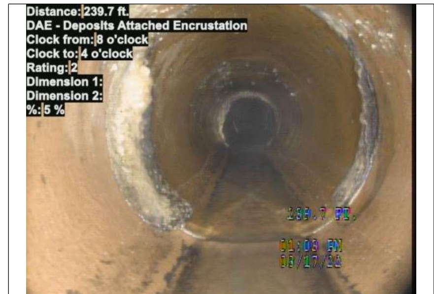
At: 239.7 ft. 8/4 DAE - Deposits Attached Encrustation Joint: No 5 %
