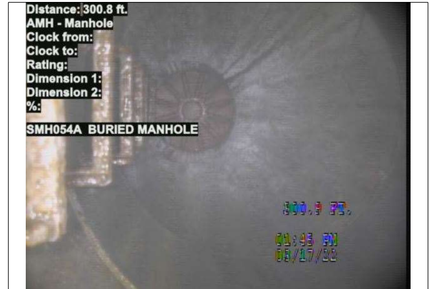
At: 300.9 ft. AMH - Manhole Joint: No SMH054A BURIED MANHOLE
