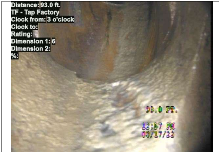
At: 93 ft. 3/. TF - Tap Factory Joint: No
