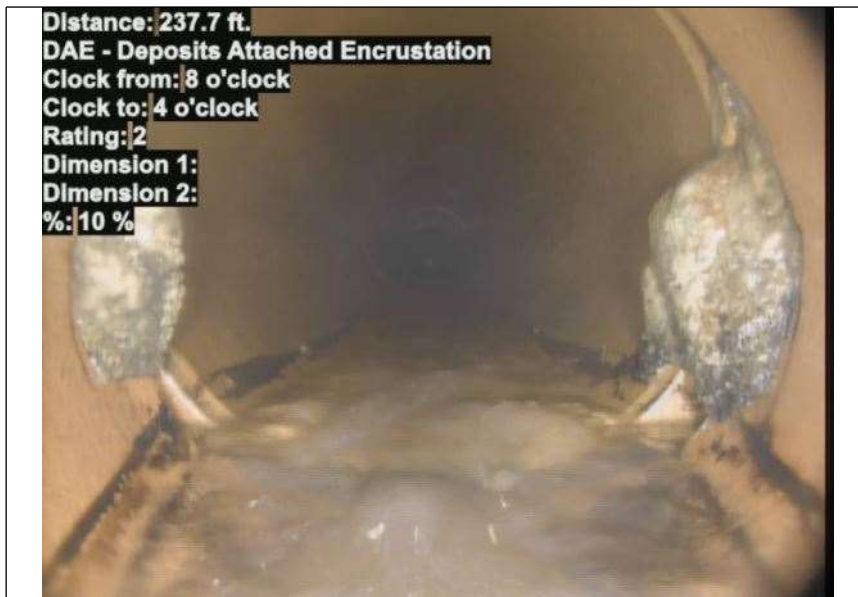
At: 237.7 ft. 8/4 DAE - Deposits Attached Encrustation
