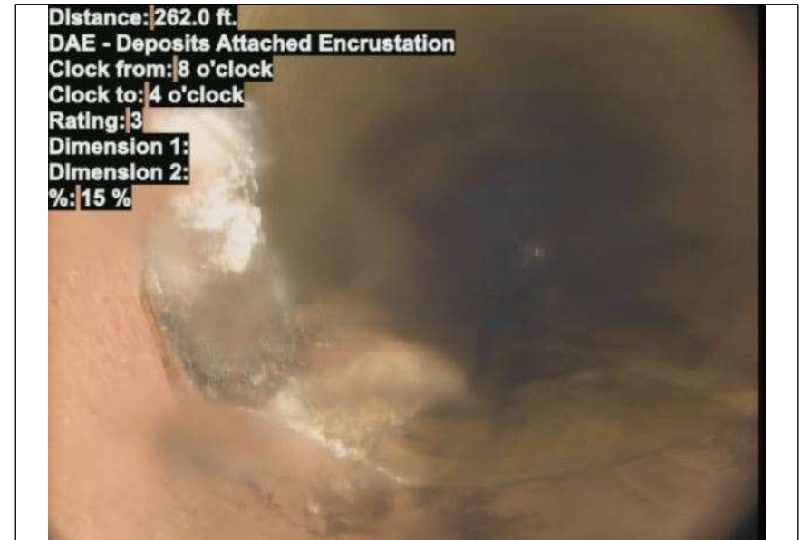
At: 262 ft. 8/4 DAE - Deposits Attached Encrustation
