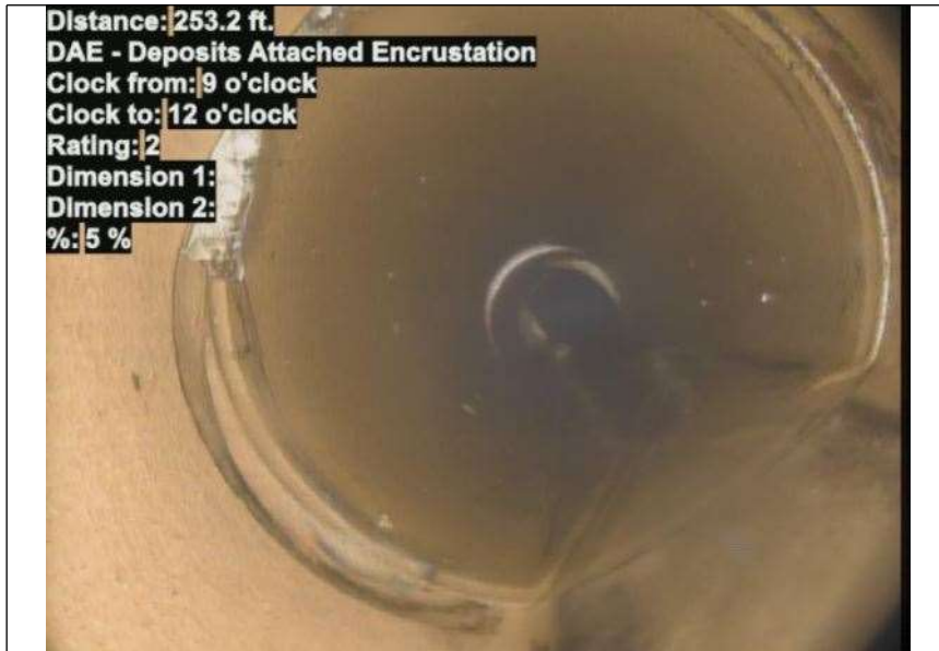
At: 253.2 ft. DAE - Deposits Attached Encrustation 9/12
