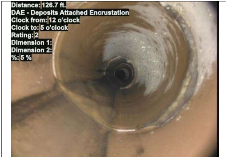
At: 126.7 ft. DAE - Deposits Attached Encrustation 12/5
