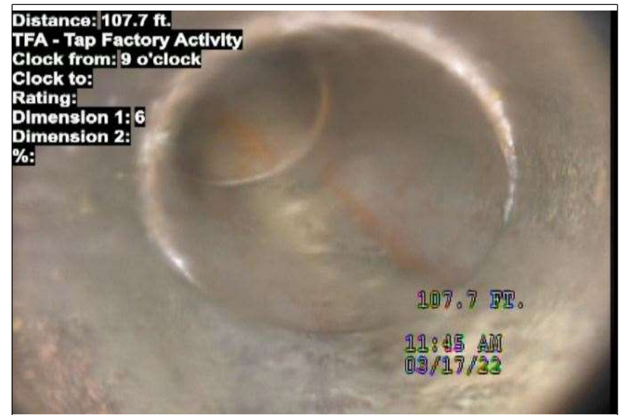
At: 107.7 ft. 9/. TFA - Tap Factory Activity Joint: No
