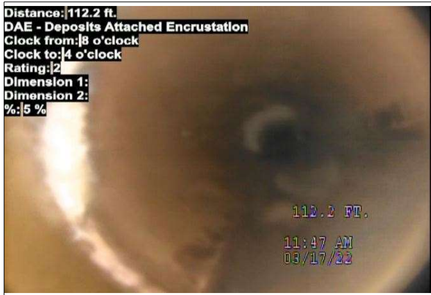
At: 112.2 ft. 8/4 DAE - Deposits Attached Encrustation Joint: No 5 %
