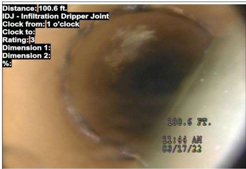
At: 100.6 ft. 1/. IDJ - Infiltration Dripper Joint Joint: Yes
