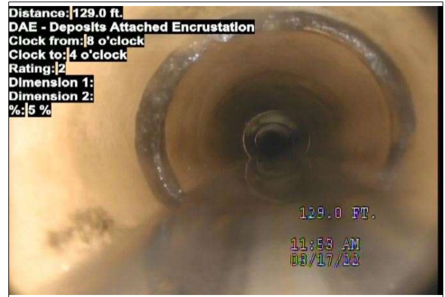
At: 129 ft. 8/4 DAE - Deposits Attached Encrustation Joint: No 5 %
