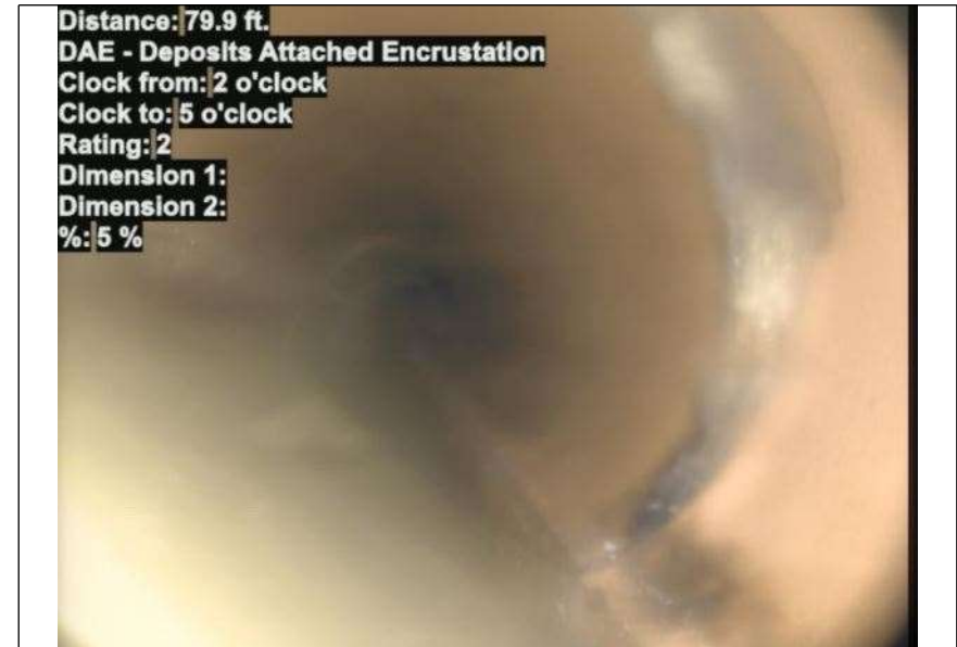
At: 79.9 ft. 2/5 DAE - Deposits Attached Encrustation Joint: No 5 %
