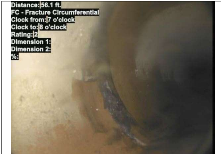
At: 56.1 ft. 7/8 FC - Fracture Circumferential Joint: No
