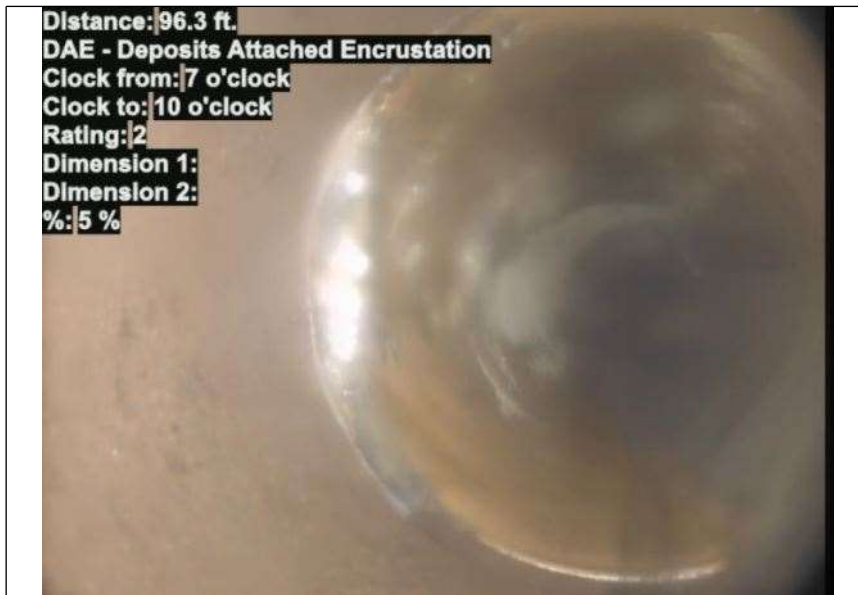
At: 96.3 ft. 7/10 DAE - Deposits Attached Encrustation Joint: No 5 %
