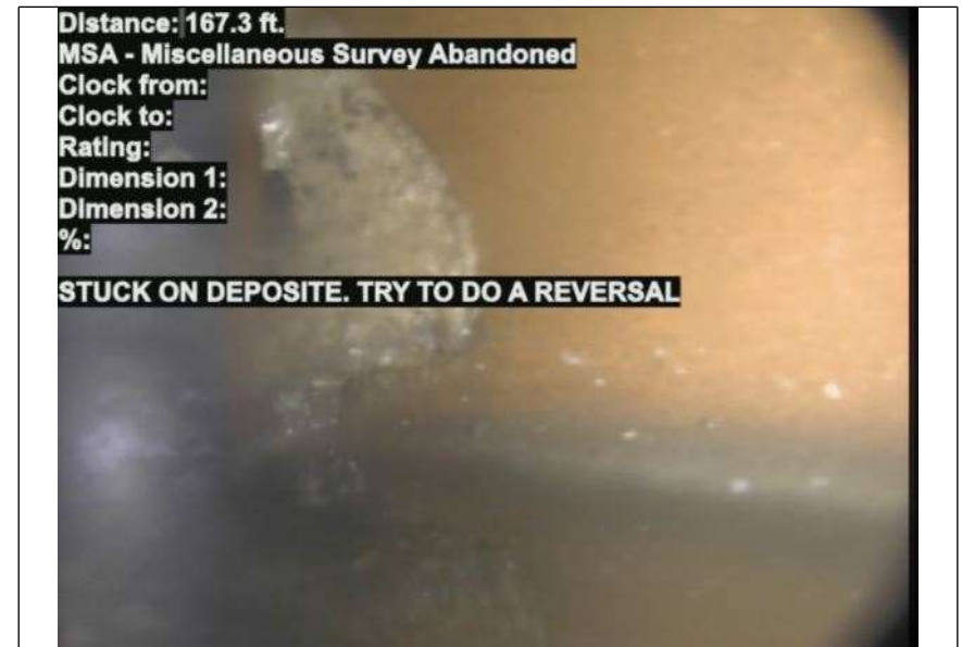
At: 167.4 ft. MSA - Miscellaneous Survey Abandoned Joint: No STUCK ON DEPOSITE. TRY TO DO A REVERSAL
