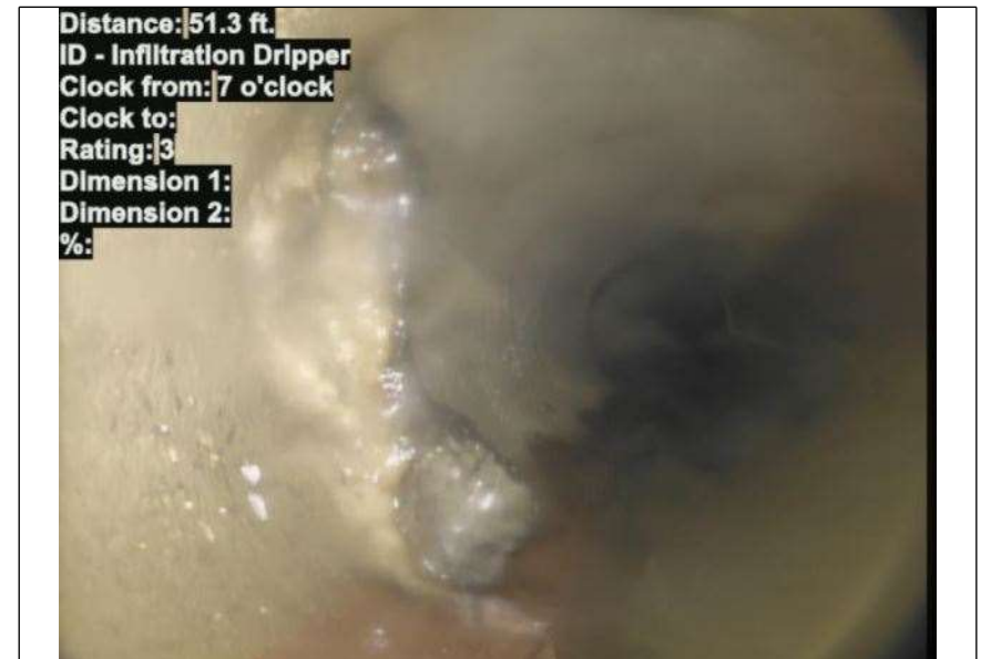
At: 51.3 ft. 7/ ID - Infiltration Dripper Joint: No
