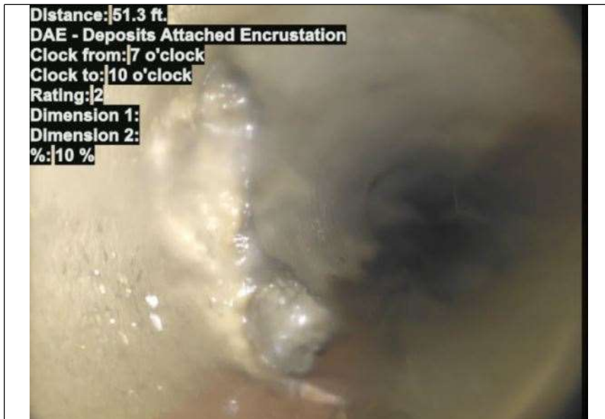
At: 51.3 ft. 7/10 DAE - Deposits Attached Encrustation Joint: No 10 %
