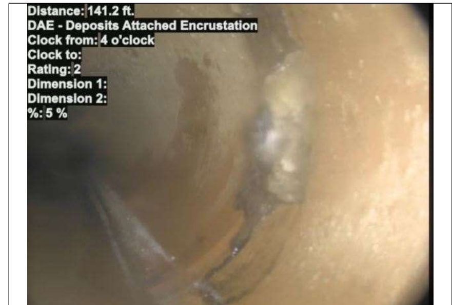
At: 141.2 ft. 8/4 DAE - Deposits Attached Encrustation Joint: No 5 %
