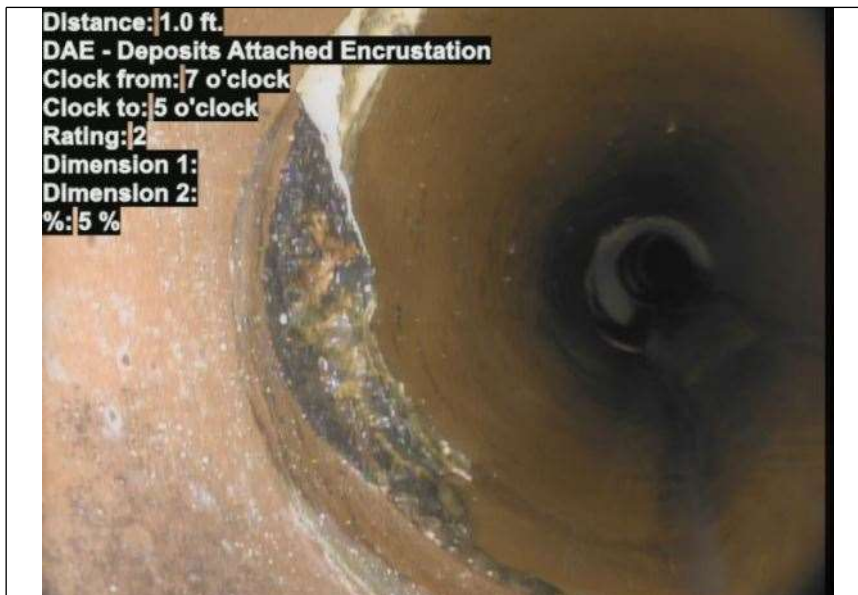
At: 1 ft. 7/5 DAE - Deposits Attached Encrustation Joint: No 5 %
