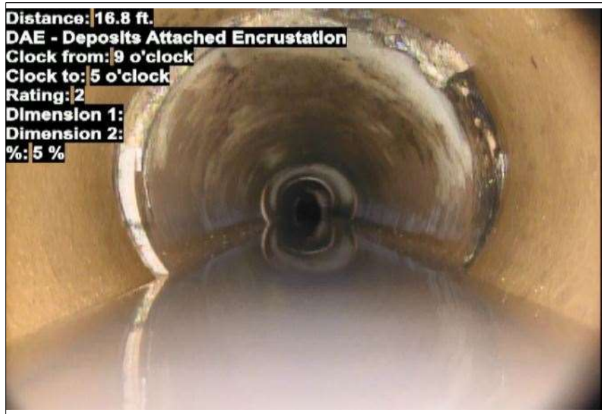
At: 16.8 ft. 9/5 DAE - Deposits Attached Encrustation Joint: No 5 %
