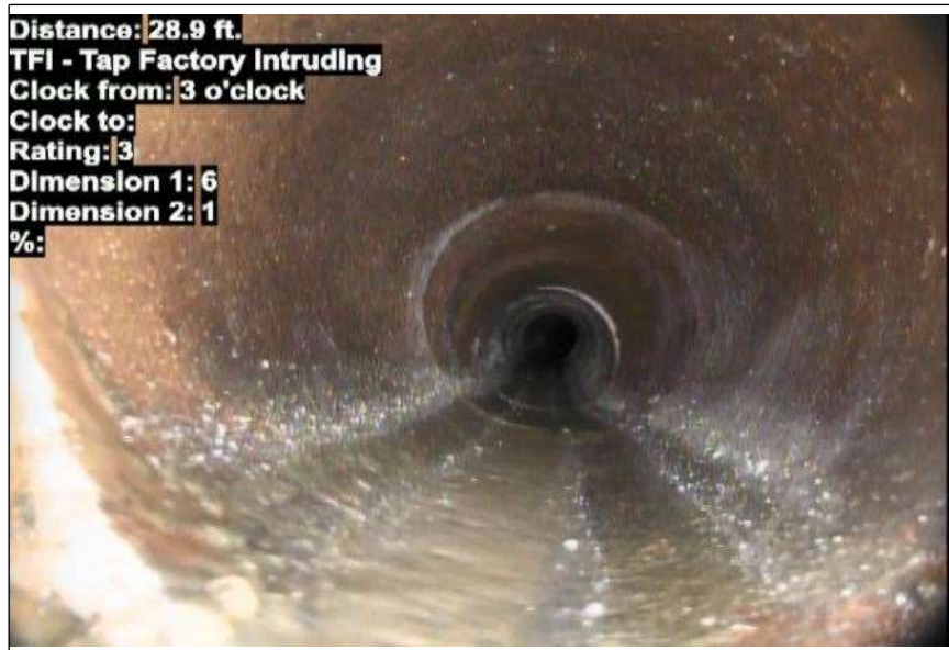
At: 28.9 ft. 3/. TFI - Tap Factory Intruding Joint: No
