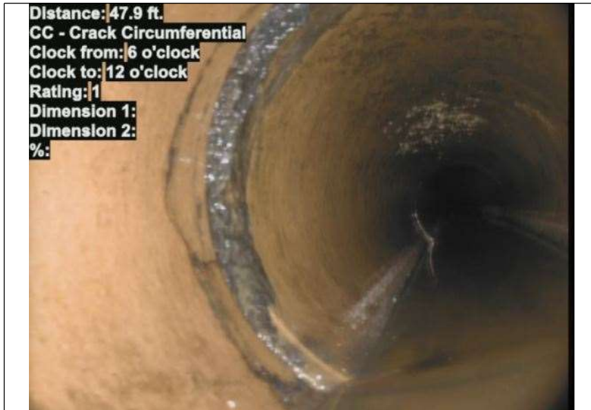
At: 47.9 ft. 6/12 CC - Crack Circumferential Joint: No
