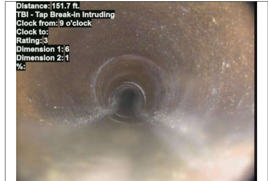
At: 151.7 ft. 9/. TBI - Tap Break-in Intruding Joint: No
