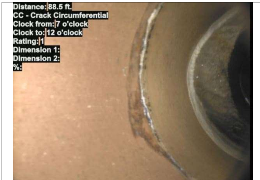
At: 88.5 ft. 7/12 CC - Crack Circumferential Joint: No
