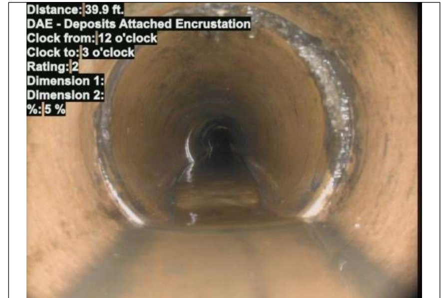
At: 39.9 ft. 12/3 DAE - Deposits Attached Encrustation Joint: No 5 %
