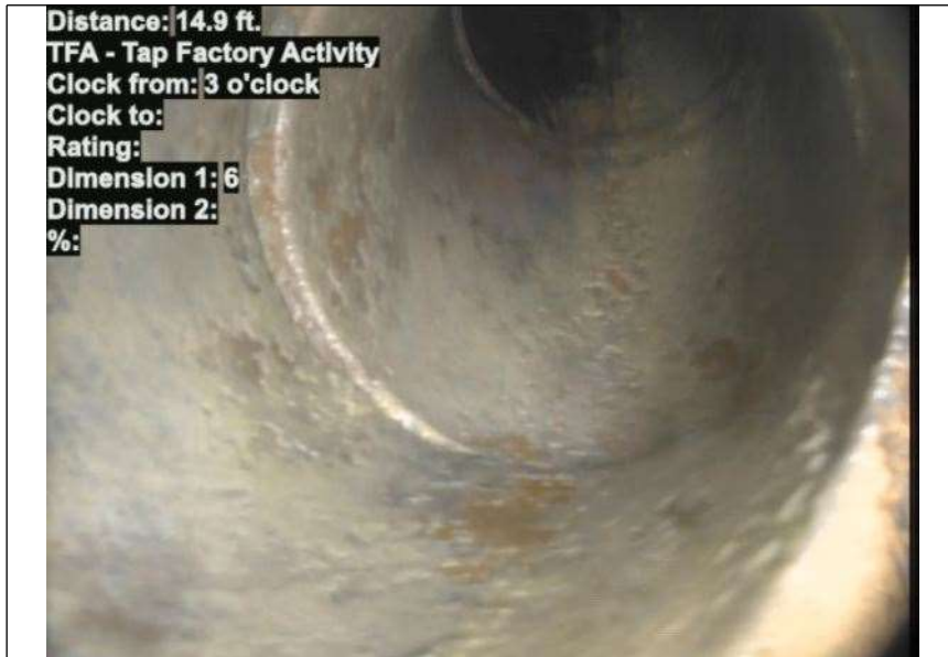
At: 14.9 ft. 3/ TFA - Tap Factory Activity Joint: No
