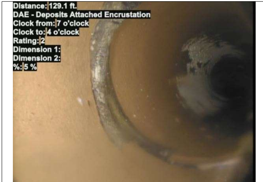
At: 129.1 ft. 7/4 DAE - Deposits Attached Encrustation Joint: No 5 %
