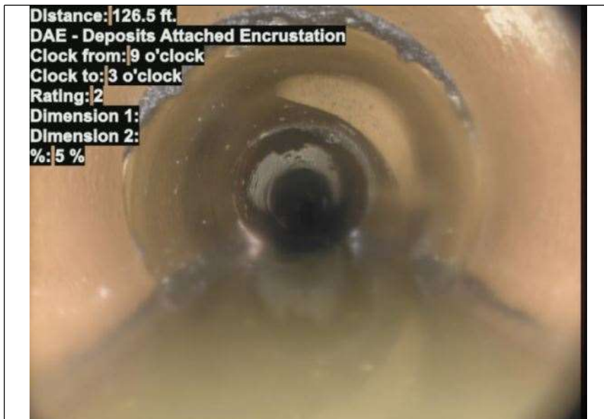
At: 126.5 ft. 9/3 DAE - Deposits Attached Encrustation Joint: No 5 %
