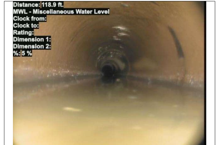
At: 118.9 ft. MWL - Miscellaneous Water Level Joint: No 5 %
