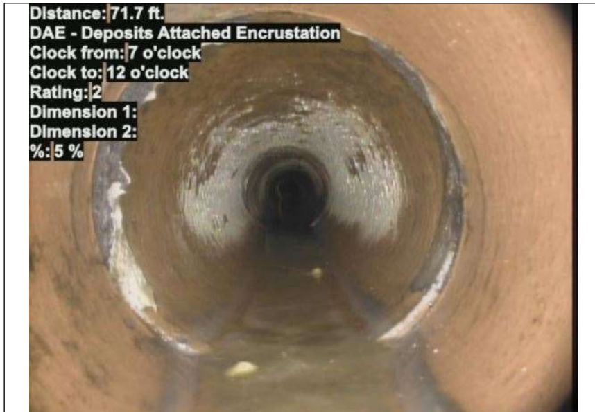
At: 71.7 ft. 7/12 DAE - Deposits Attached Encrustation Joint: No 5 %
