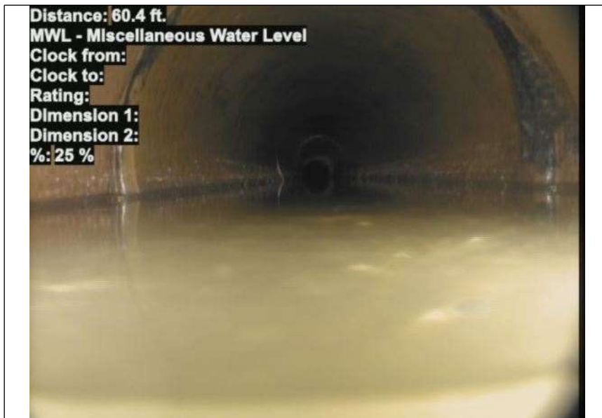
At: 60.4 ft. MWL - Miscellaneous Water Level Joint: No 25 %
