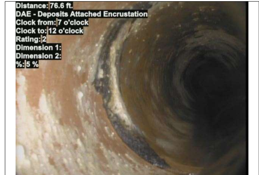
At: 76.6 ft. 7/12 DAE - Deposits Attached Encrustation Joint: No 5 %
