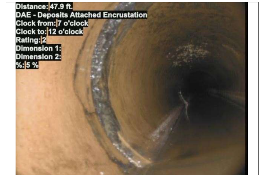
At: 47.9 ft. 7/12 DAE - Deposits Attached Encrustation Joint: No 5 %
