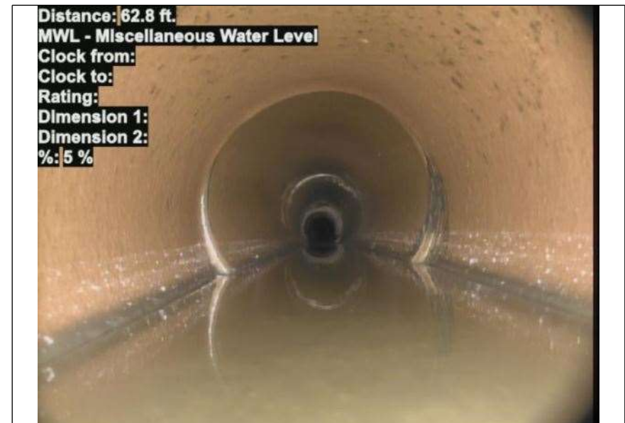
At: 62.8 ft. MWL - Miscellaneous Water Level Joint: No 5 %
