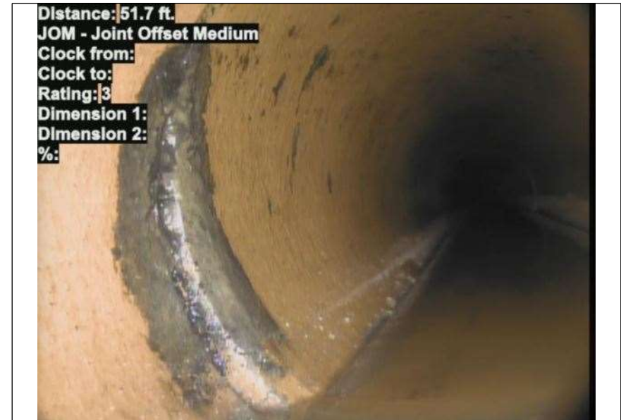
At: 51.7 ft. JOM - Joint Offset Medium Joint: No
