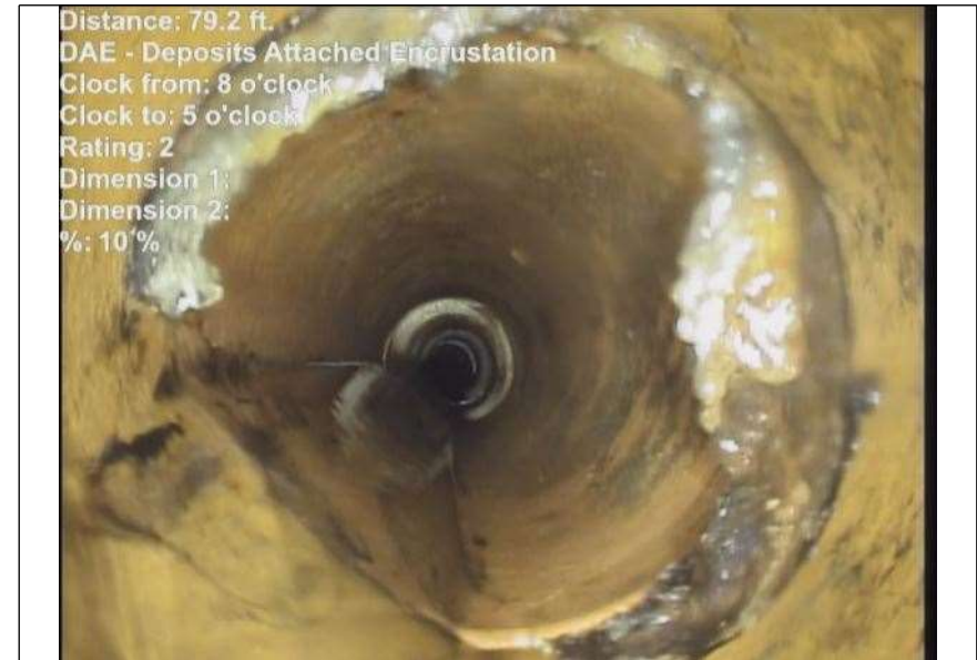
At: 79.2 ft. 8/5 DAE - Deposits Attached Encrustation Joint: No 10 %
