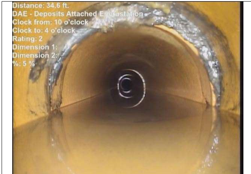
At: 34.6 ft. 10/4 DAE - Deposits Attached Encrustation Joint: No 5 %
