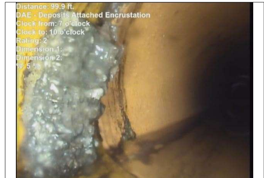
At: 99.9 ft. 7/10 DAE - Deposits Attached Encrustation Joint: No 5 %
