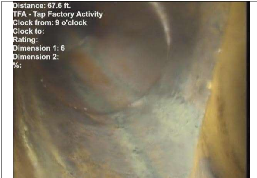
At: 67.6 ft. 9/ TFA - Tap Factory Activity Joint: No
