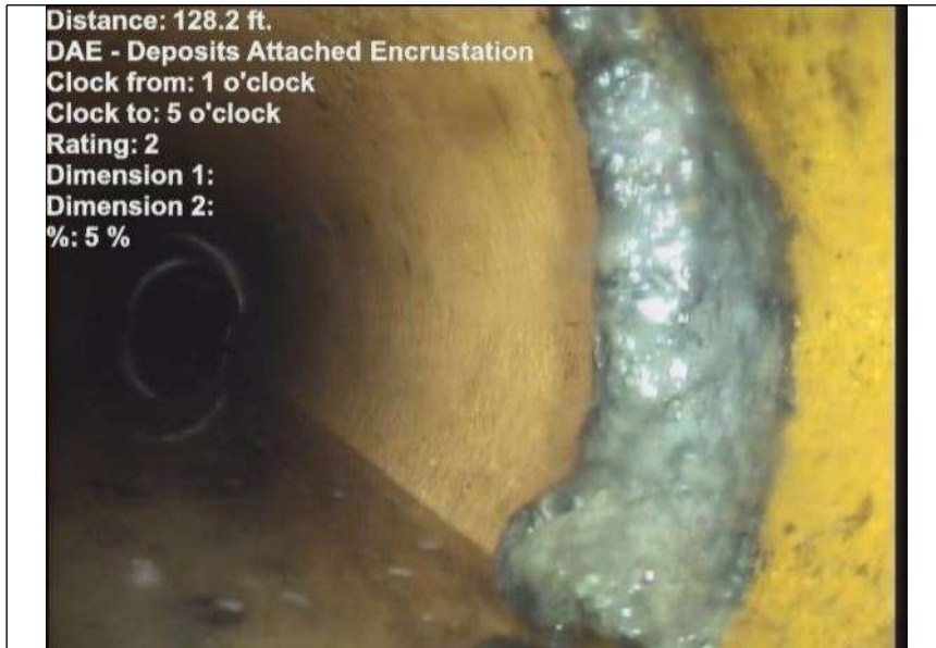
At: 128.2 ft. 1/5 DAE - Deposits Attached Encrustation Joint: No 5 %
