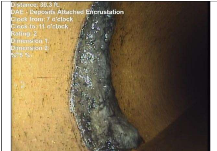
At: 30.3 ft. 7/11 DAE - Deposits Attached Encrustation Joint: No 5 %
