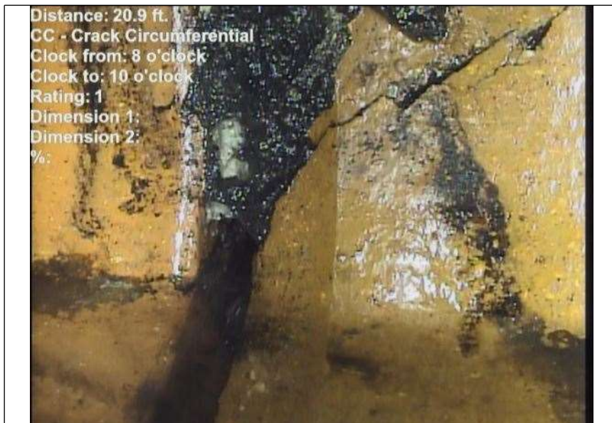
At: 20.9 ft. 8/10 CC - Crack Circumferential Joint: No
